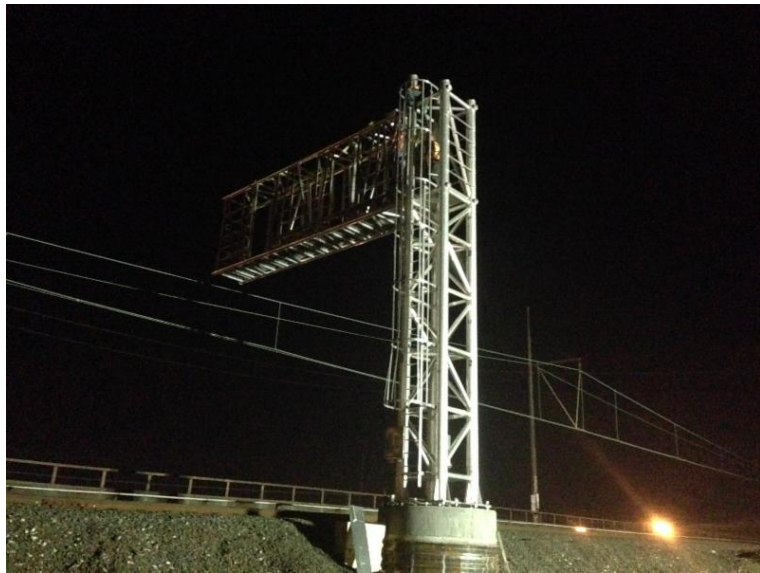
Installation of signal bridge 24
