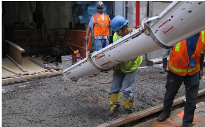
Pouring the new sidewalk at 44th Street
