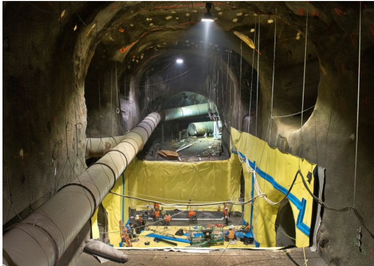
Waterproofing below 50th Street
