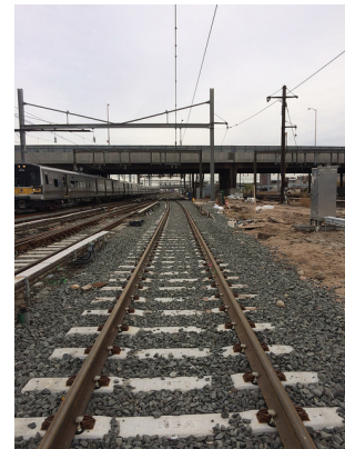
Installation of new track in Harold Interlocking
