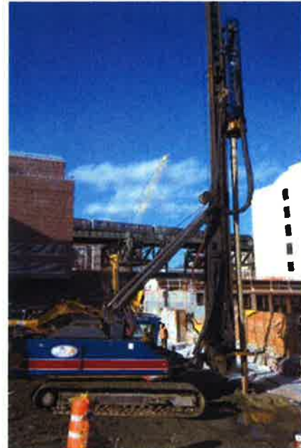
Pile driving operation underway at Northern Boulevard
