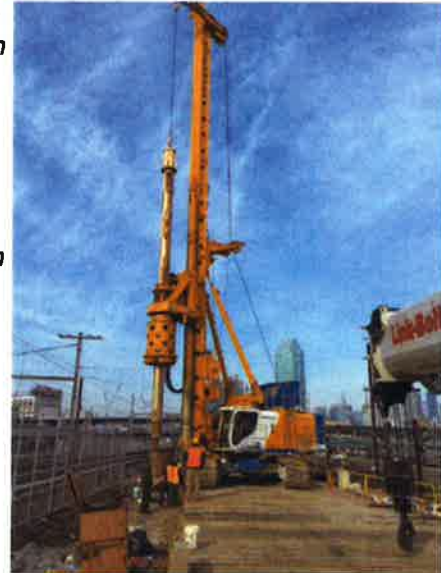
Secant pile installation for the East Approach
