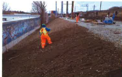
Grading adjacent to the future Westbound Bypass track area
