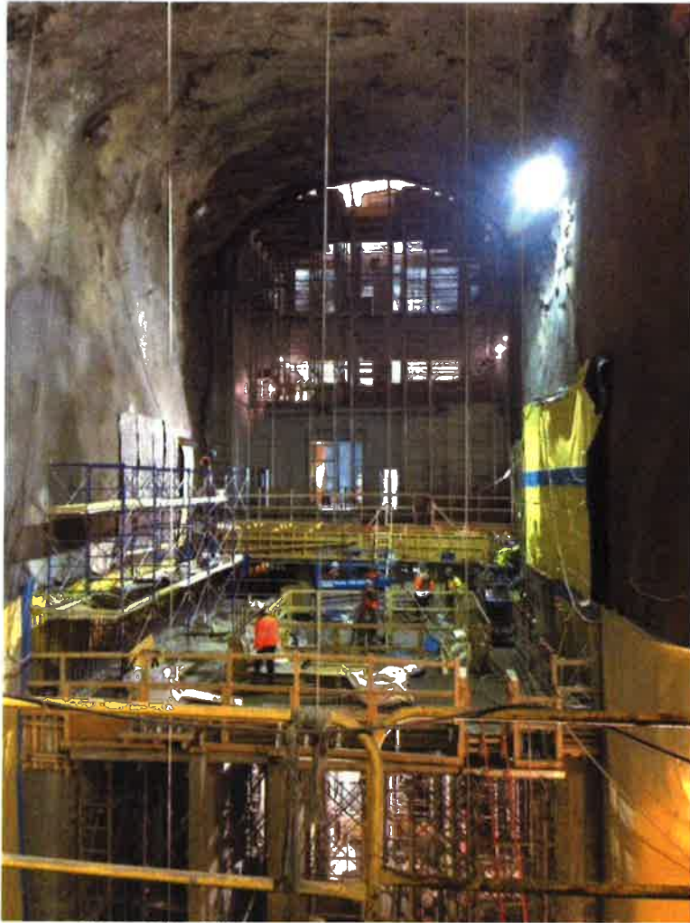
View of the 55th Street Vent Facility in the background
