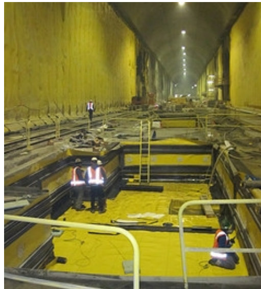
Waterproofing throughout the caverns
