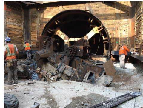
Removal of the cutterhead (Click the photo view a larger version)
