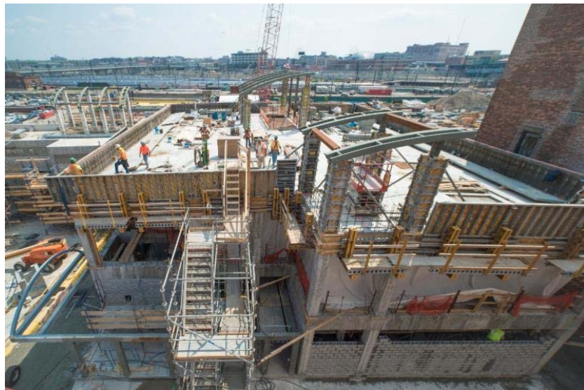
Construction of columns, floors and walls for the Yard Services Building
