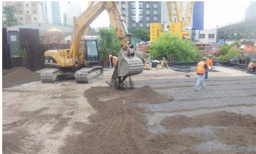
Partial backfilling of the Bellmouth underway during early July 2015
