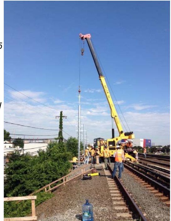
Erection of a supplemental steel pole within Woodside
