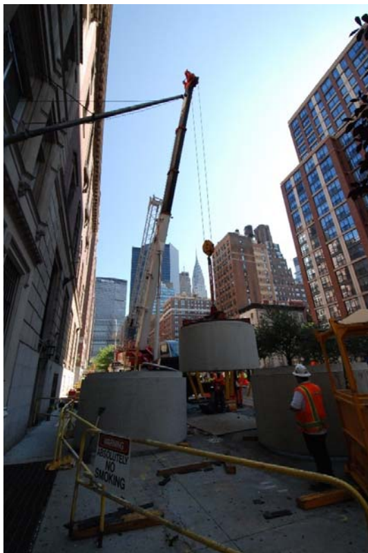
Installation of pre-cast concrete lining for the below ground ventilation facility
