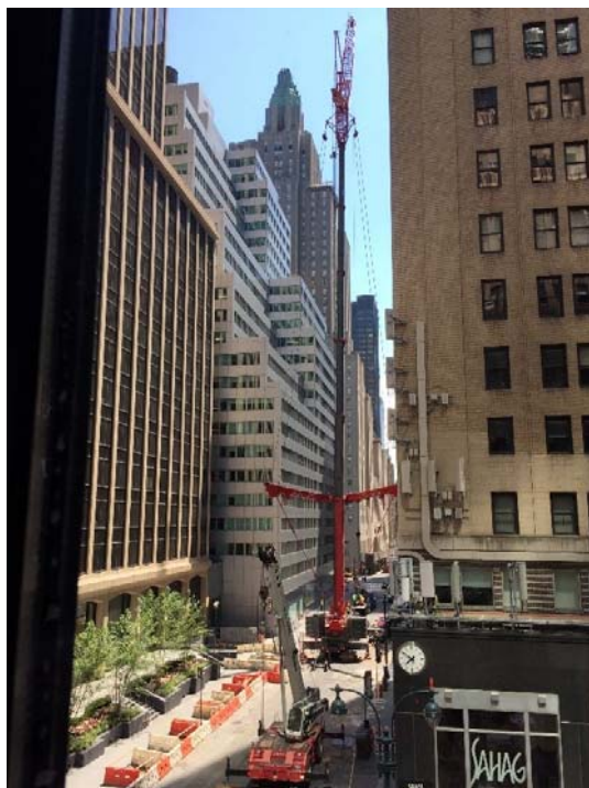
Cooling tower installation atop 300 Park Avenue
