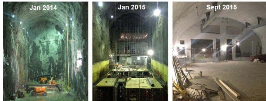
Timeline of 55th Street Ventilation Facility Construction Progress
