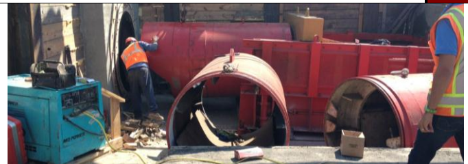
Tunneling Subcontractor Setting Shield for 12KV.
