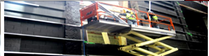
Metal Cladding Frame Install, Rear Face of Vent Building.
