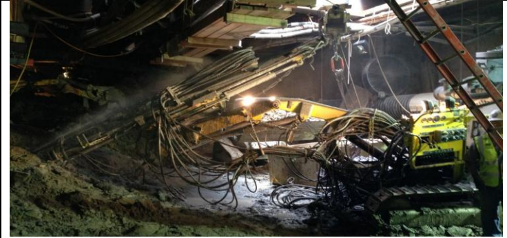
Drilling Relief Holes.
