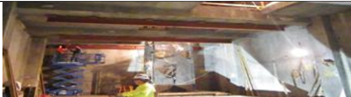
Hoist Beams Installation, Vent Shaft Floors.
