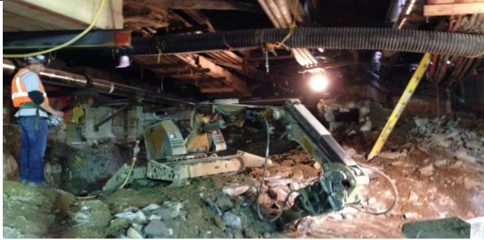
Hoe Ramming Below Decking – North.
