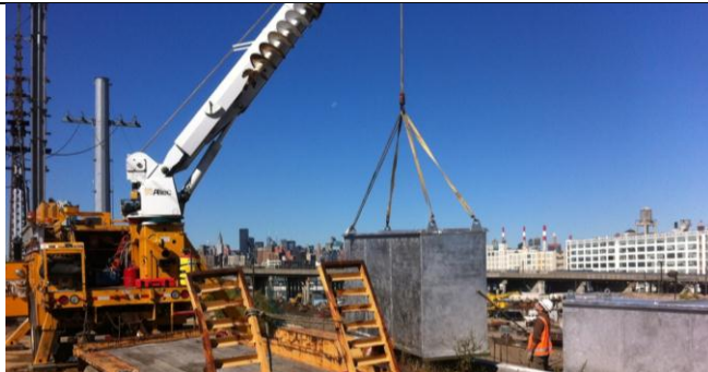
Installing Power Case at Signal Tower 34.
