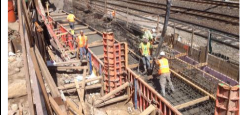
Pouring Pile Cap at 43 rd St. MLA Bridge West Abutment.
