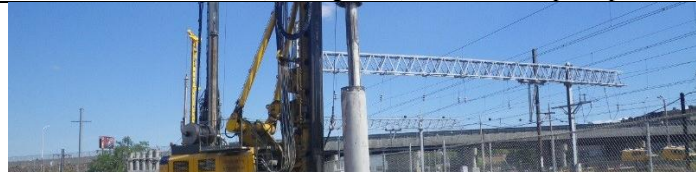
Drilling Secant Pile for Tunnel A Approach.
