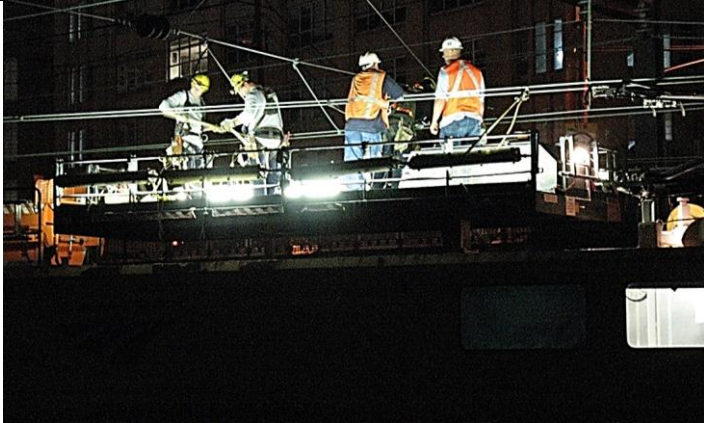
Catenary Wire Transfers on Line 3 from B-906E to B-918E.
