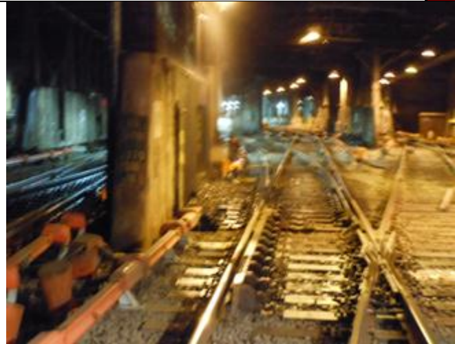
New Track Joint 2 (D & E) at Track #37 G.L 18+00.
