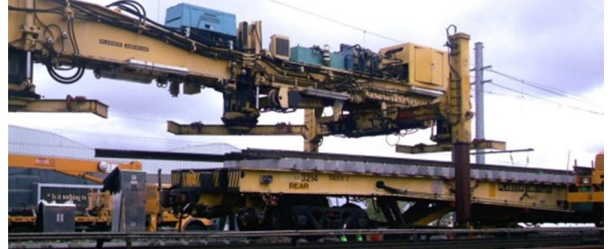
H2 (6156E) Switch Panel Installation on Port Washington 2 Track.
