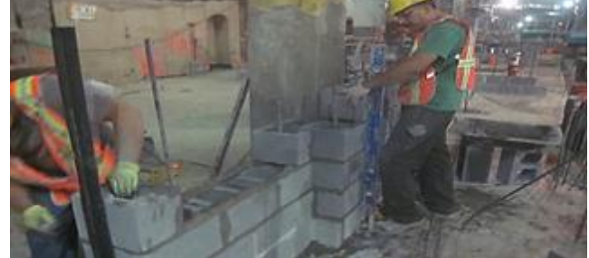
Constructing CMU Walls for Transformer Room.
