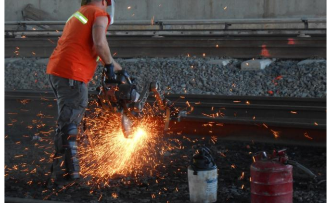
Cutting Scrap Rails from Line 2 and Line 4 (Summer Outage).
