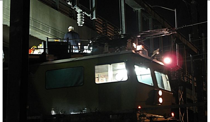
Remove Catenary Body Span Wires at B-926W.
