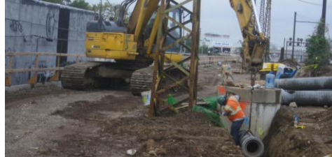
Installing Storm Sewer at 43-S2 Retaining Wall.
