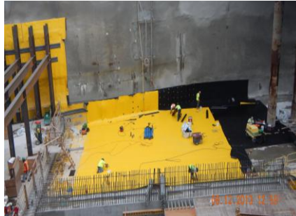
Installing Waterproofing for Track A Slab.
