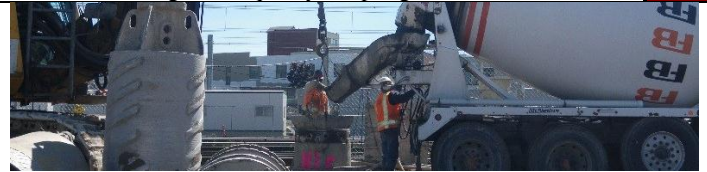
Pouring Concrete for Tunnel A Approach Secant Piles.
