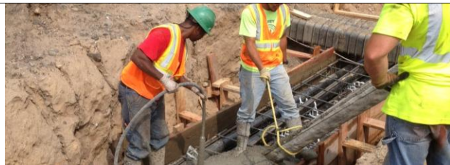
Pouring Concrete for Open Cut 12KV Ductbank.
