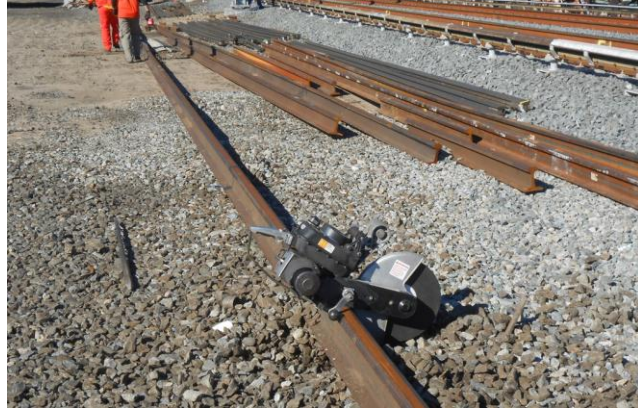
Cutting Old Rails and Cleaning Up the Work Area.
