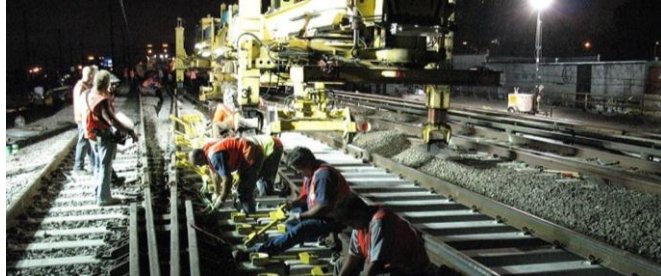
H2 (6156E) Switch Installation on Port Washington 2 Track.
