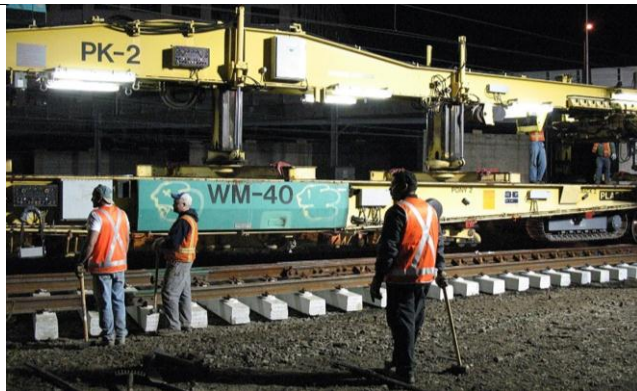
AG1 (835) Switch Installation on WWD LI Passenger Track.
