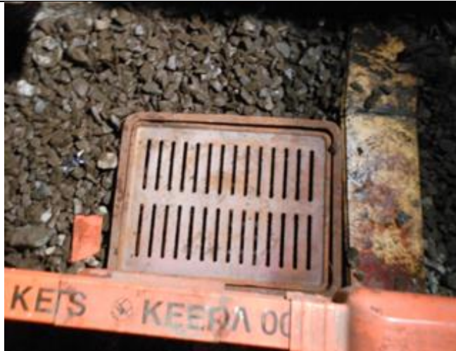
New Track Drain at Track #37 Completed by CM002.
