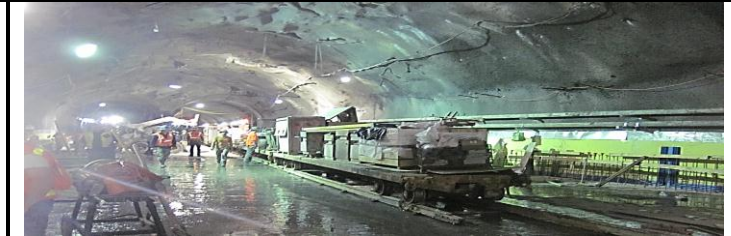
Demobilization in GCT4 Cross Over.
