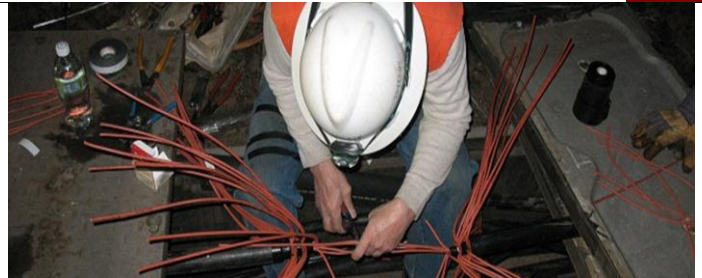
Splicing Cables for Signal Revision Near F1B Hut Location.
