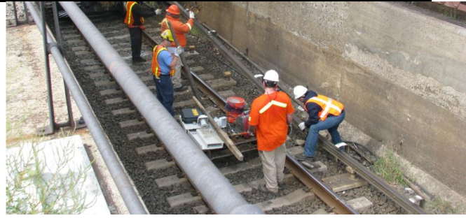
Track Shift and Re-Alignment at Hunters Point Ave.
