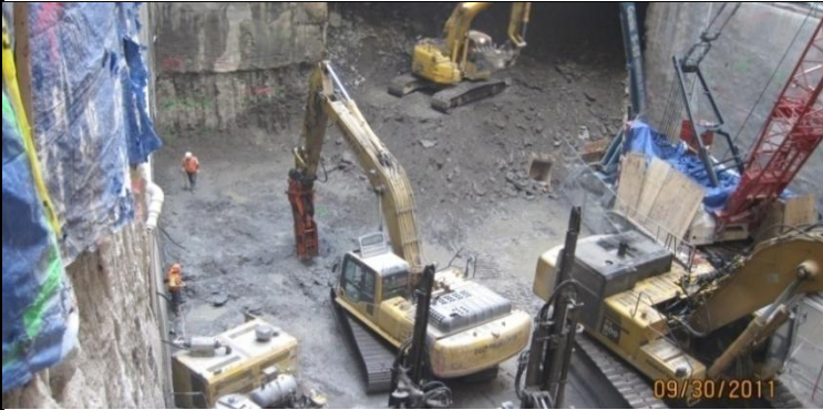
Vent Building Excavation and Rock Support and Shotcrete Installation.
