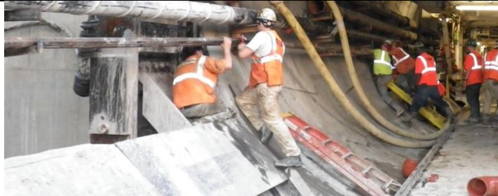
Extending Grout Lines.
