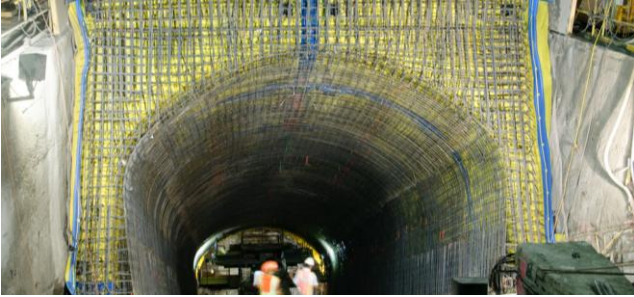
Rebar Installation in Wellway #4.
