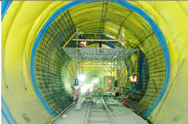
Tail Tunnel (T302) Arch Rebar Installation.
