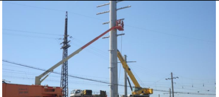
Signal Tower 22 Erection and Installation of Cross Arms.
