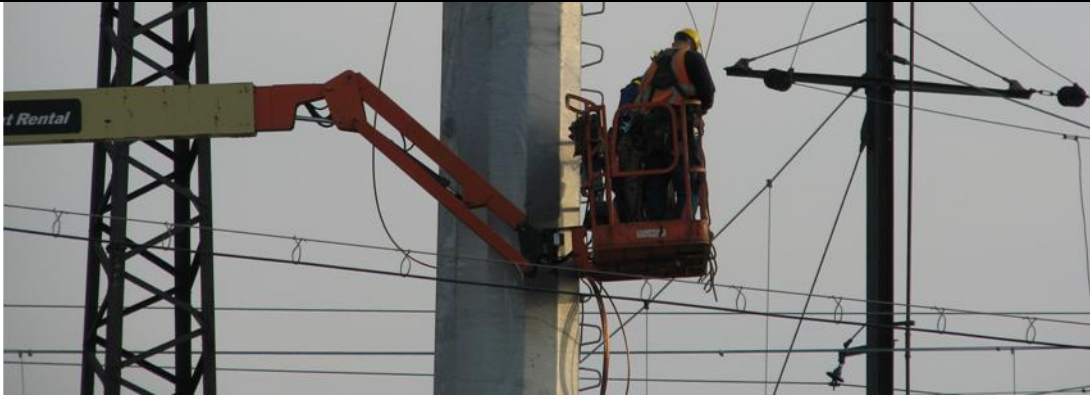
Pulling Signal Power Cables Between Towers 22 to 23.
