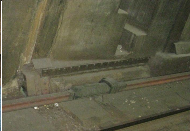
Longitudinal Expansion Joint Replacement at Track #40.
