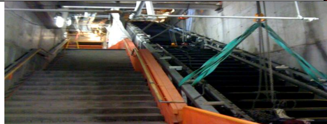
On-going installation of Escalator at 245 Park Avenue.
