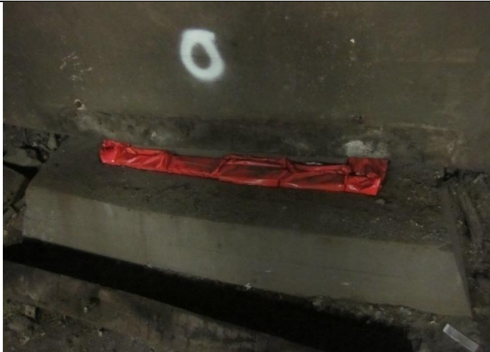
Firestopping installation at Track 34.
