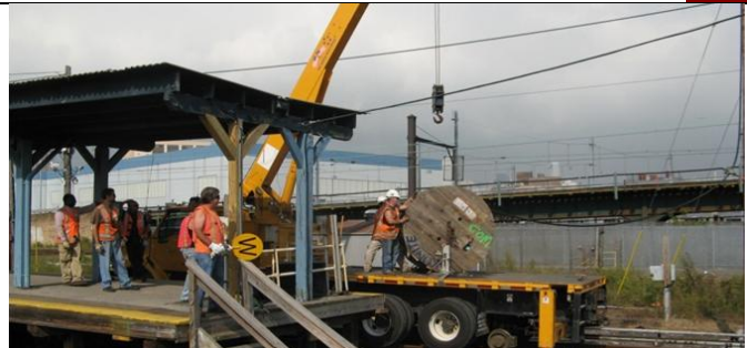
Pulling Communication Cable at Hunters Point Station.
