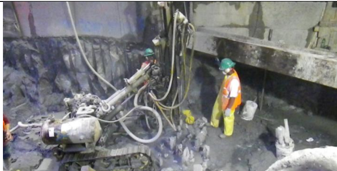
Drilling Rock Formation Using Air Track Drill.
