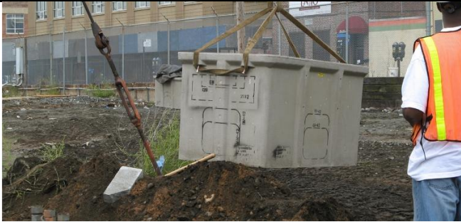
Installing Pull Box on South of Line 1 at Hunters Point Ave.
