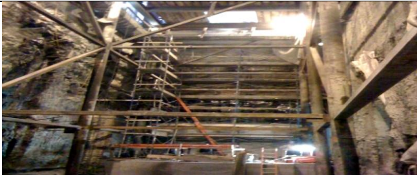
On-going Construction of Foundation Walls at 44 th Street.
