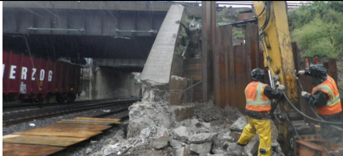
43rd St. Westbound Bypass Demolition of Existing Wing Wall.
