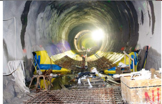
EB4 Invert Rebar Installation.
