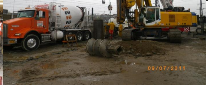
Concrete Being Placed in Secant Pile #2.
