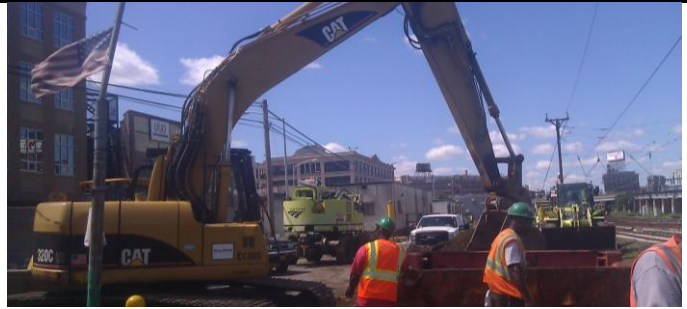
Excavating for Guy Anchor Installation.
