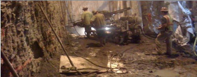
Installation of Final Row of Rock Anchors at 44 th Street.
