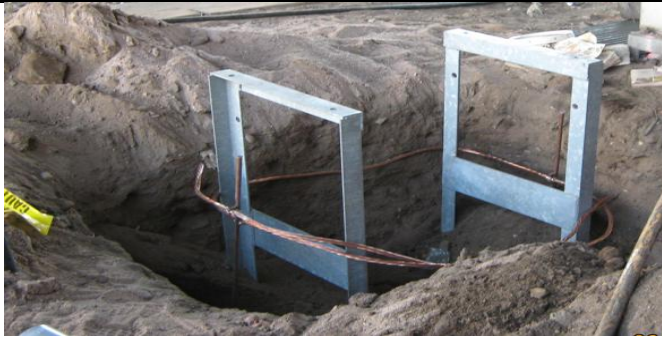
Leg Foundations for 37A Signal Case under Honeywell St.
