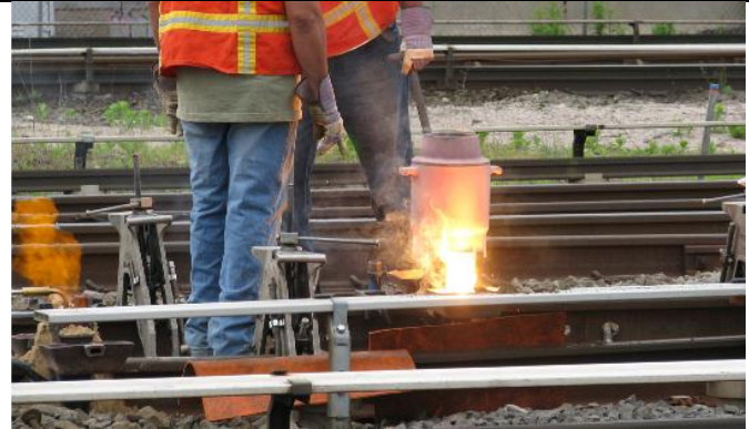
Boutet Welding on Westward LI Pass at East End of 823 Crossover.
