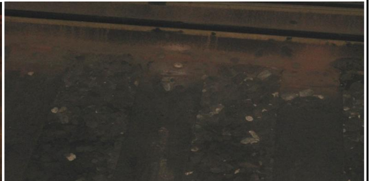
Upcoming Expansion Joint Replacement at Ballasted Track Bed.
