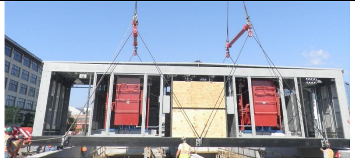
G02 Substation Installation.
