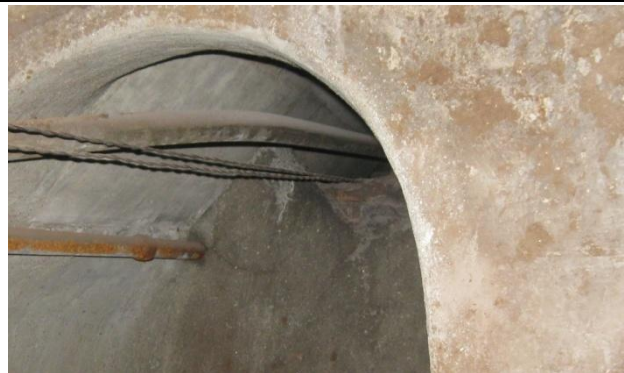
Flag and Power support to TC Electric Under GCT Platform R.
