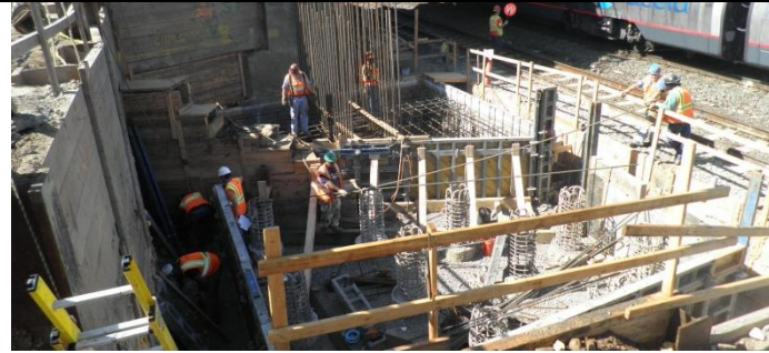
Pier 1 Installation at 43rd Street Bridge.
