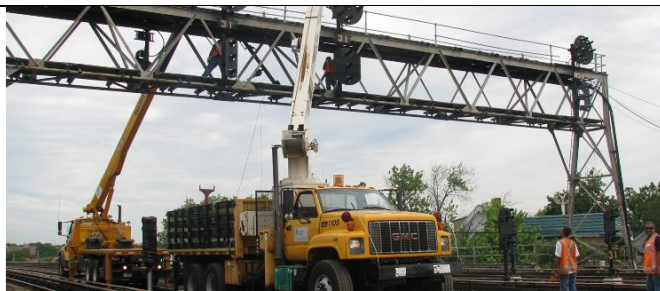
Remove Existing Signal on Bridge 30 at Location 30 (Woodside Station).
