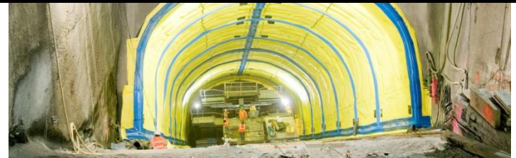
Escalator Shaft 4 Waterproofing.
