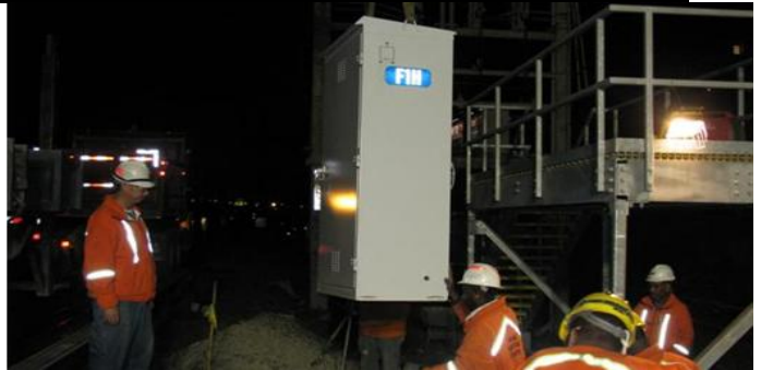
Installing F1H Signal Case West of Thomson Ave.
