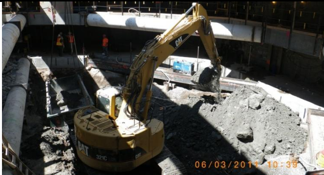
Continued Excavation for Level VI Slab.
