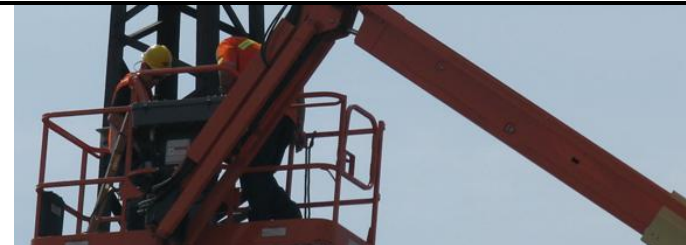
Install Support Brackets on Tower 26 (West of 39th St).
