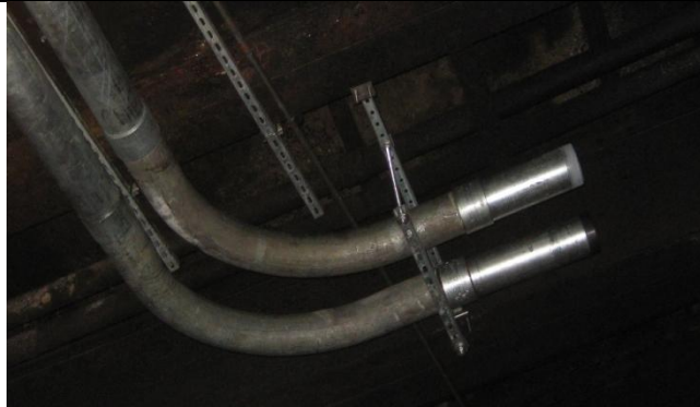
Flagman Protection for New Feeder Bends.
