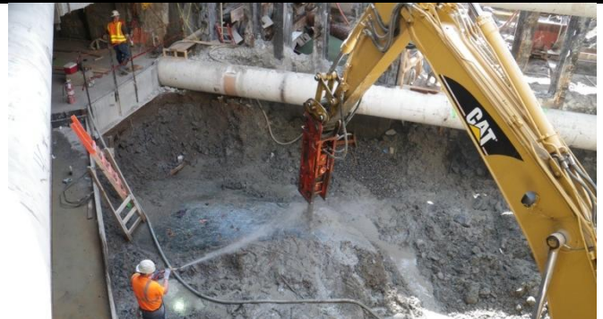
Dismantling Rock at Middle Part of EAC Excavation.
