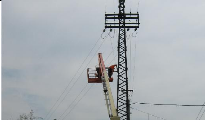
Installing Hardwares on Tower 26 and 1017 Pole.
