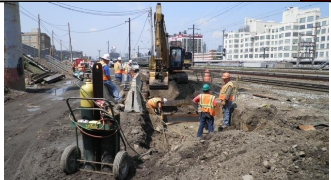
Installing Support of Excavation.
