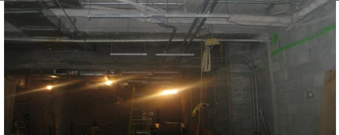
Fit-Out at 245 Park Ave (Ground Floor).
