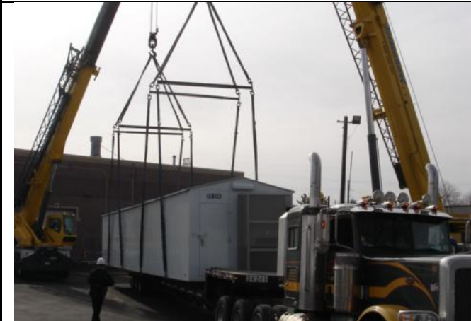
Installation of F2 CIH at Thomson Ave.
