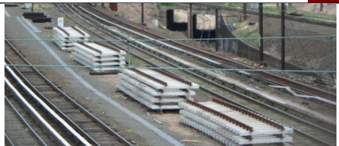
Track Panels for EWD LI Pass Construction.
