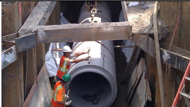
Installing 48 inch Sewer Pipe.
