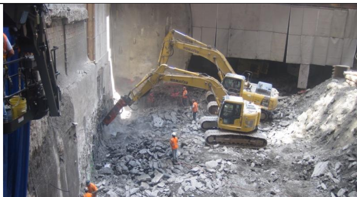
Vent Plant & Service Tunnel Excavation.
