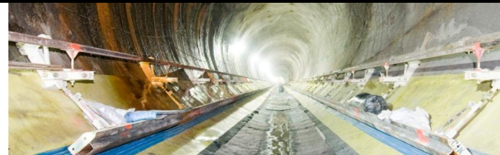
302 Tunnel Waterproofing.
