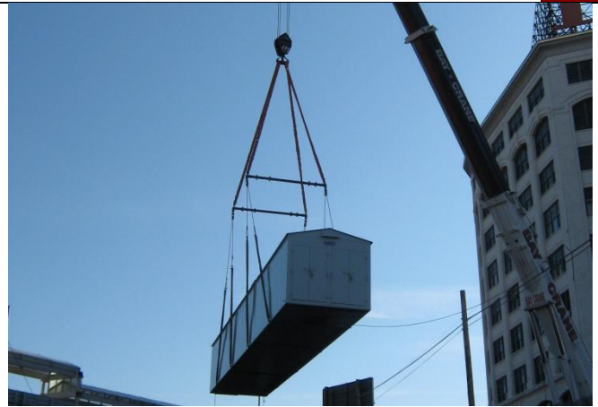
Installation of F2 CIH at Thomson Ave.
