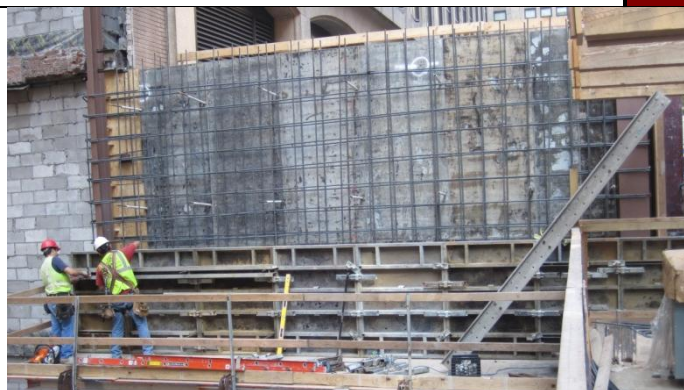
437 Madison Ave North Wall Form/Pour/Rebar.
