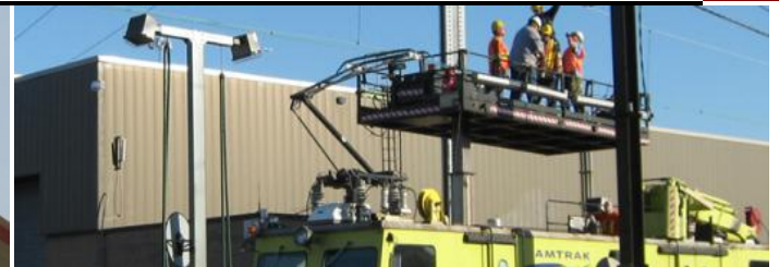
Install Catenary Assembly at B-929W in Sunnyside Yard.
