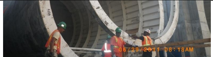
Carpenters Continue Installing Forms for LB B-C.
