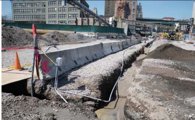
Trench Excavation for Installation of Temporary Utility Lines.
