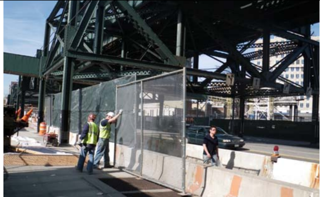
Site Walk Closure and Fencing for Slurry Wall Repair.
