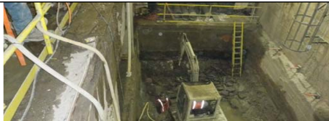
Hoeram Excavation at Shaft #2.
