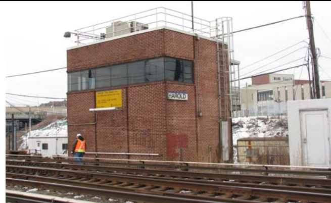
Harold Tower Supervisory Control System - Existing Tower.
