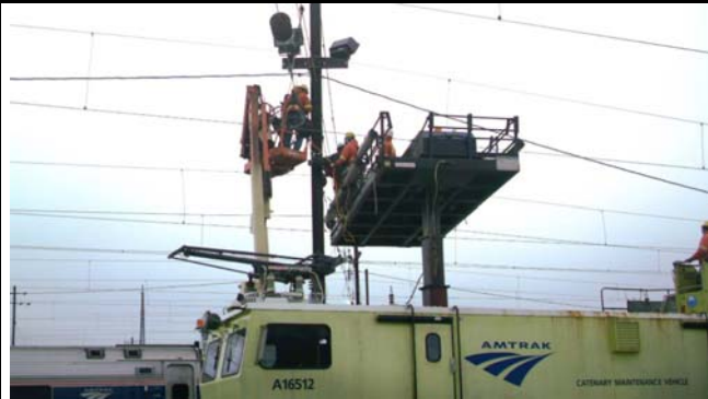
Transfer Catenary Wire B-923 in Sunnyside Yard.
