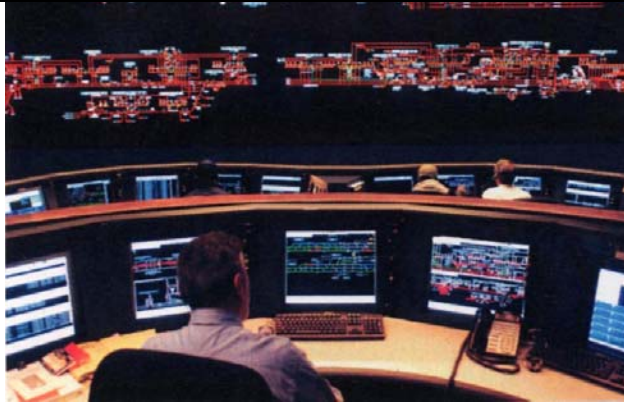
Supervisory Control System (Sample).
