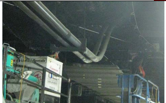
Net Installation at Platform R.
