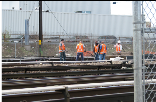
Pulling Communication Cable at 43rd Street.
