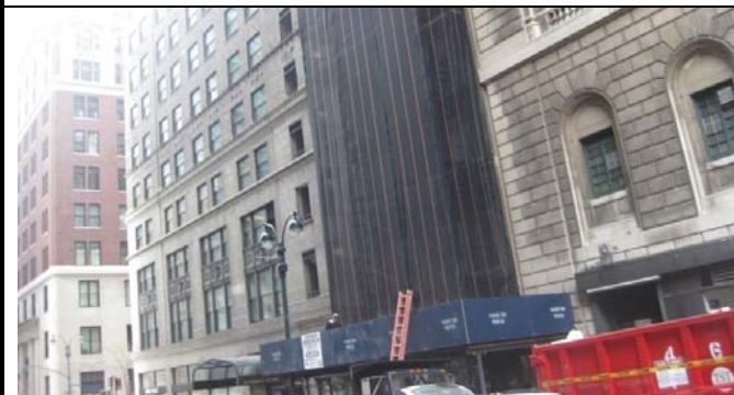
Sidewalk Bridge Completed 47 East 44 th Street.
