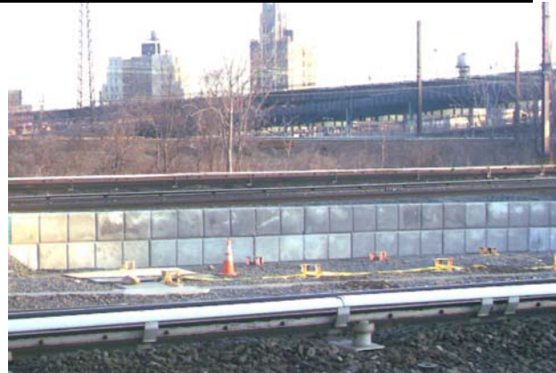
Installation of Retaining Wall East of Thomson Ave.
