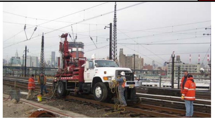
Drilling Piezometers at Sunnyside Yard.
