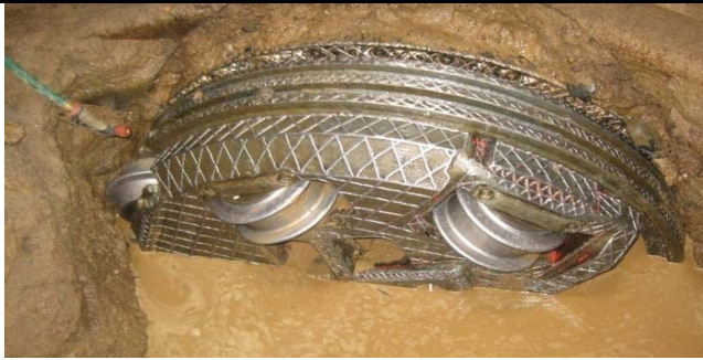
Micro-Tunnel Machine Breaks Out at Observation Shaft Run 6-7.
