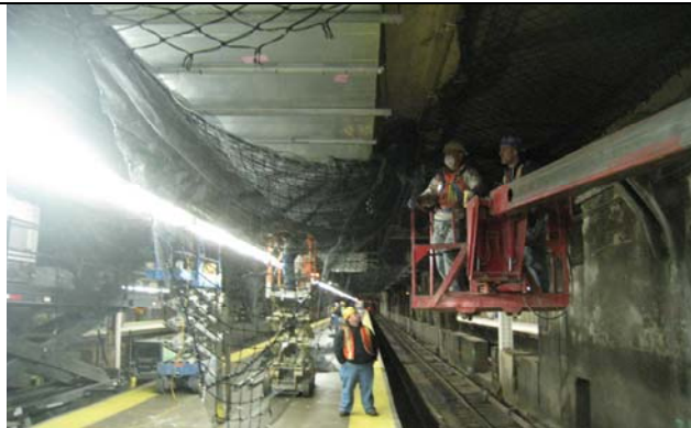
Net Installation at Platform T.
