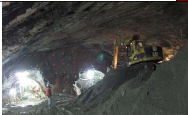
Mucking from the West Cavern.
