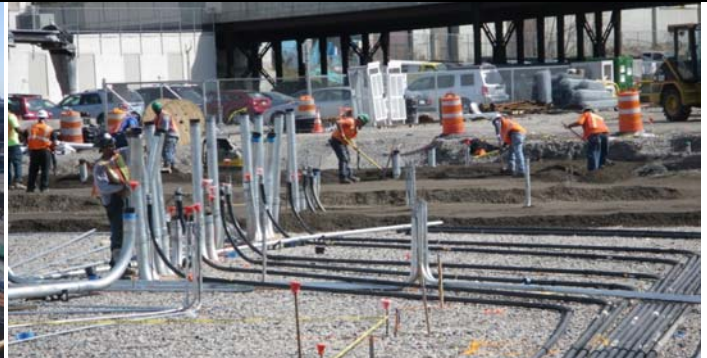
Installing Conduits at Temporary Substation.
