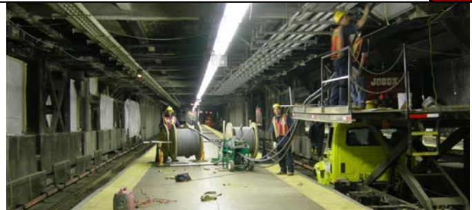
Cable pull for new 13.2KV feeder at Platform U.
