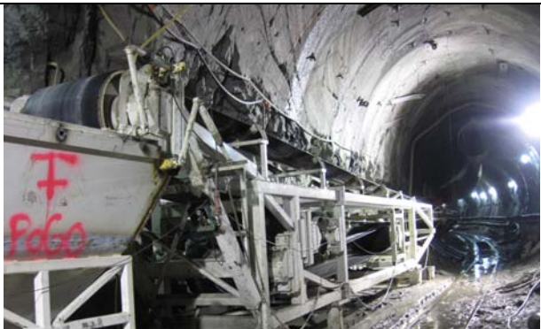
Hopper at Cross Passage #4.
