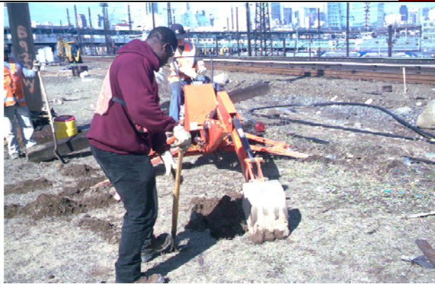
Trenching Conduit and Pull Box for AC Negative Return.
