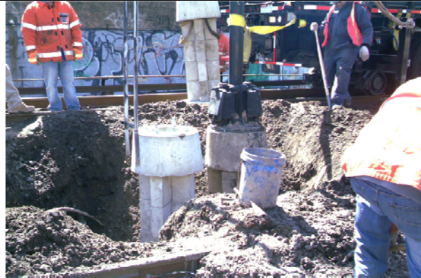
New Signal Foundation Installation at Hunterspoint Ave.
