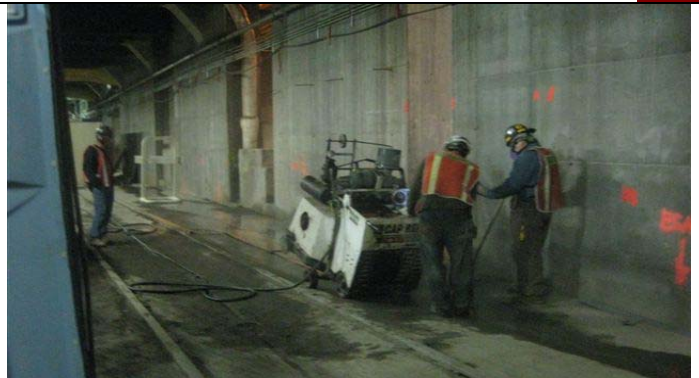
Sawcutting and Excavation at West Perimeter Wall.
