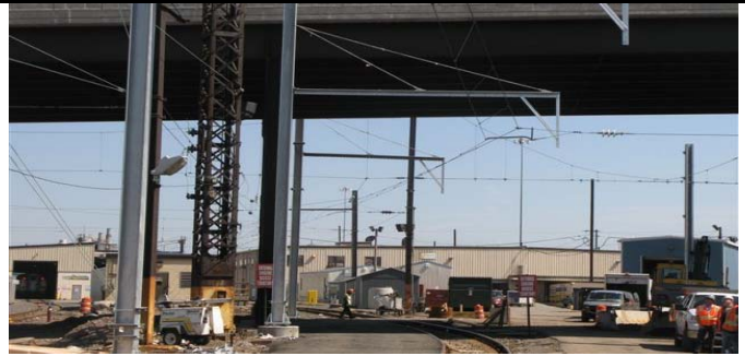
Installed Catenary Steel Structure Subset F in Sunnyside Yard.
