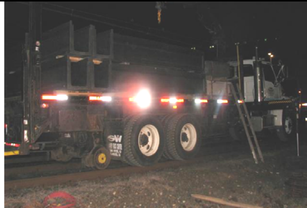
Material Handling of Signal Trough East of Thomson Ave.
