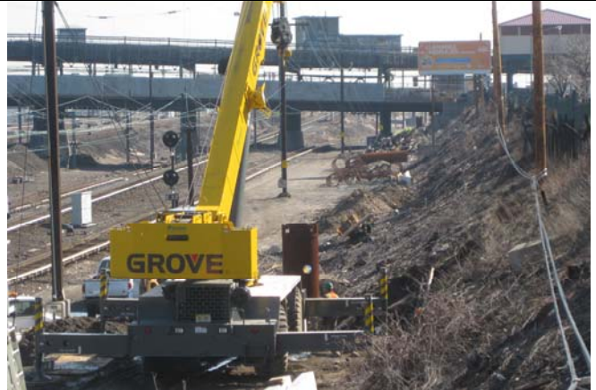
Installation of Steel Casing at Retaining Wall THOM-S2.
