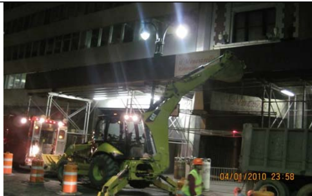
Trench Excavation for Utility Relocation on 50 th St.
