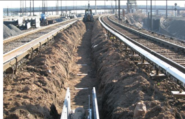
Trough Installation at East of Queens Blvd.
