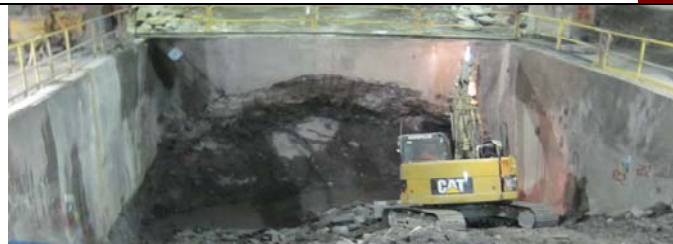
Ongoing Excavation at Wellway #4.
