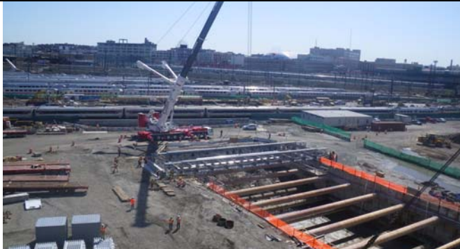
Installing the Vehicular Bridge near Northern Blvd.
