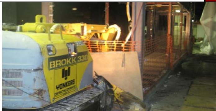
Demolition of Headhouse North of platform at East 245 Park Ave.
