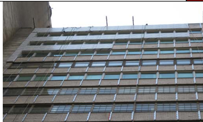
Cladding Installation at 300 Park Ave.
