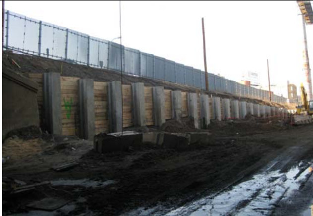
Installation of Retaining Wall THOM-S1.
