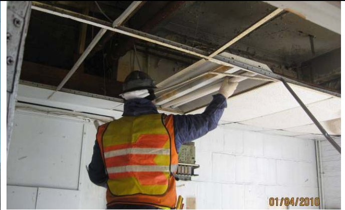
Removing Light Fixtures at Amtrak's Building 1, 2 and 5 in Preparation of Building Demolition.
