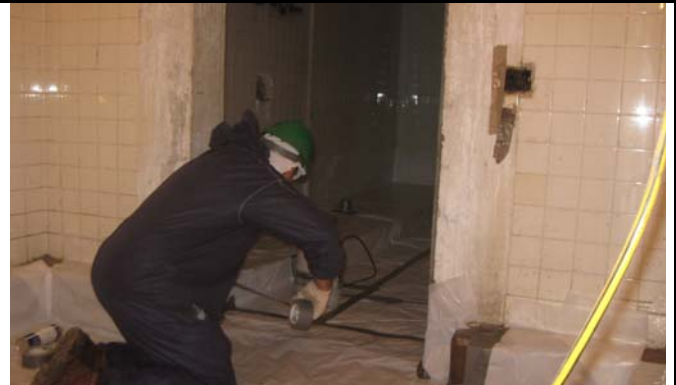
Preparation for Asbestos Abatement in Amtrak Buildings.
