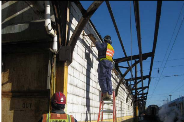
Removing Light Fixtures at Amtrak's Building 1, 2 and 5 in Preparation of Building Demolition.
