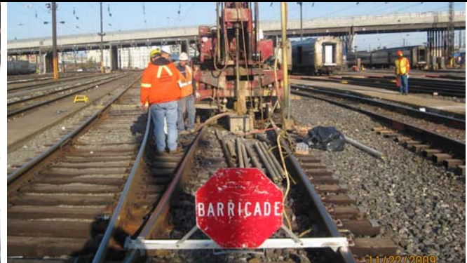
Drilling Inclinator in Sunnyside Yard.
