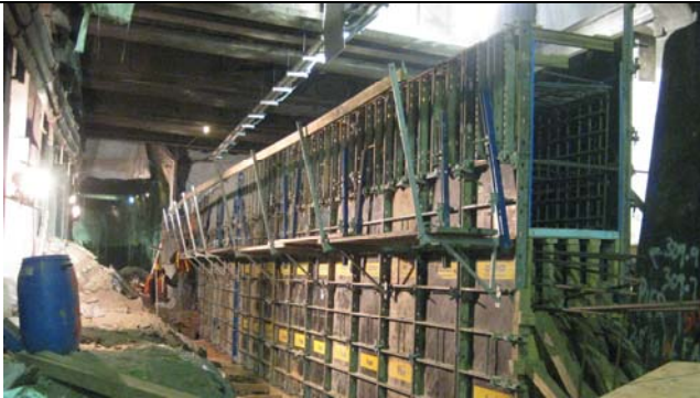
Formwork and Rebar for New Crash Wall.
