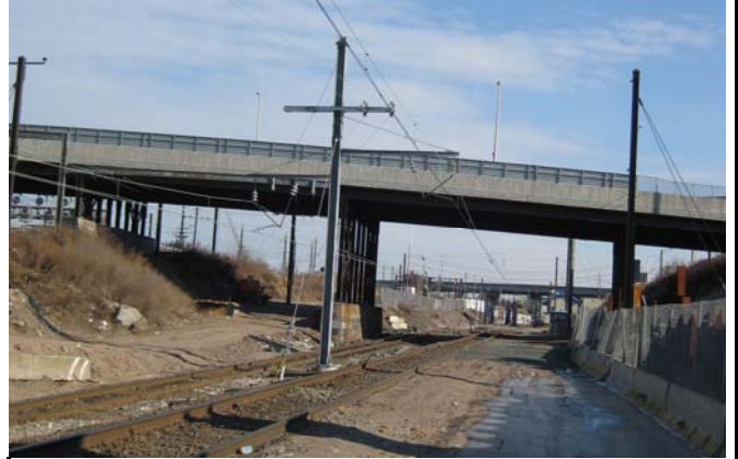
Construction Area for THOM-S2.
