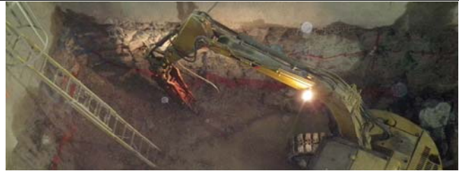
Hoe Ramming at Shaft #4.
