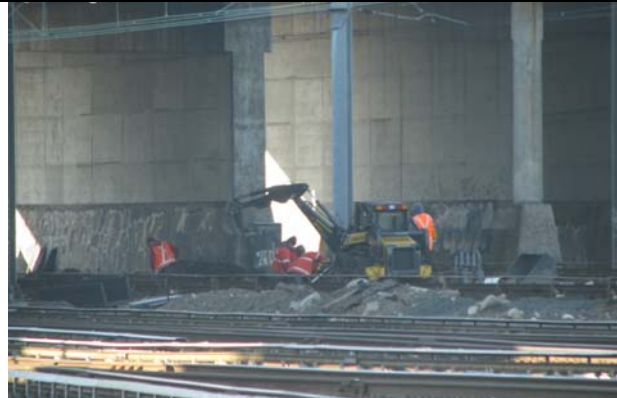
Trough Installation East of Point CIL Thomson Ave.
