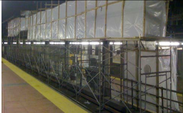
ACM Pipe Insulation Abatement at Track 37.
