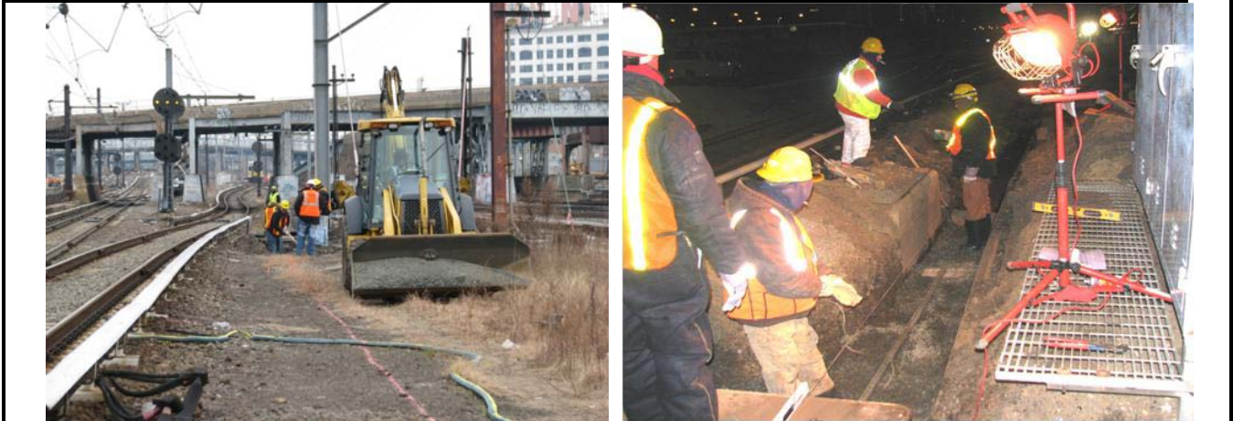
Trough Installation at East of Hunter Point.
