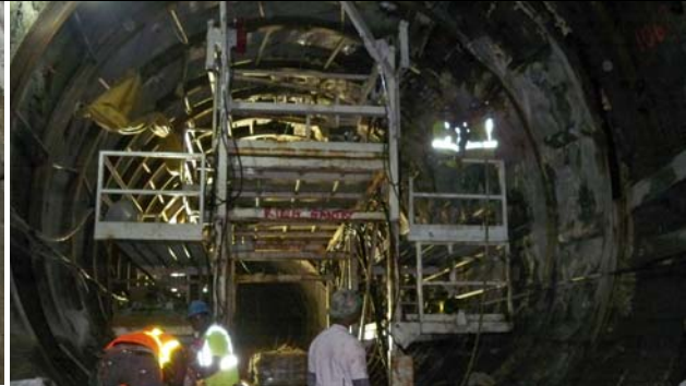
Ring Gantry at Rib 3 Cathedral..
