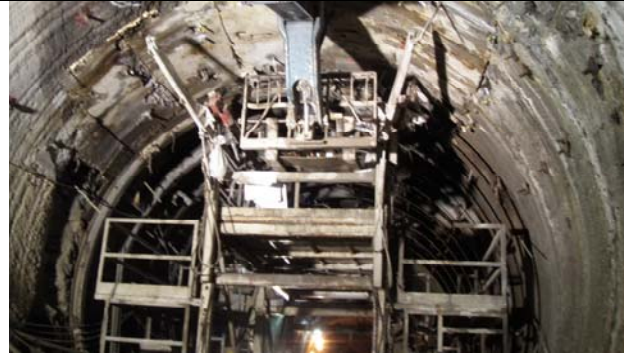
Ring Gantry Ready for Disassembly at GCT East Bound.
