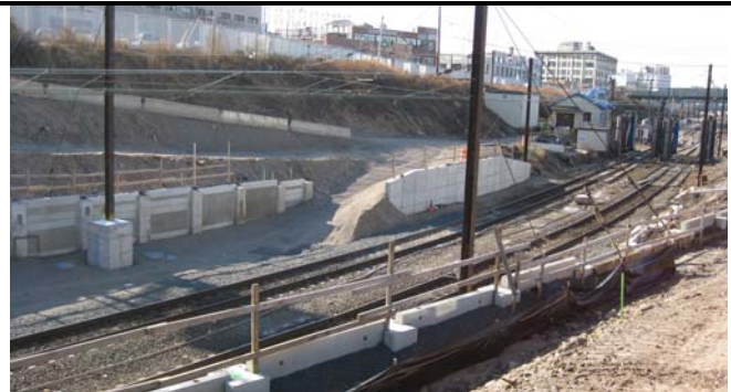
Installation of Retaining Wall 39-S1, 39S2 and 39-S3.
