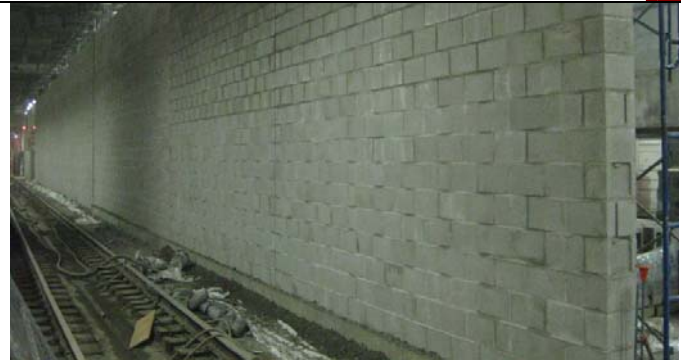
Concrete Masonry Unit Work at East Perimeter Wall.
