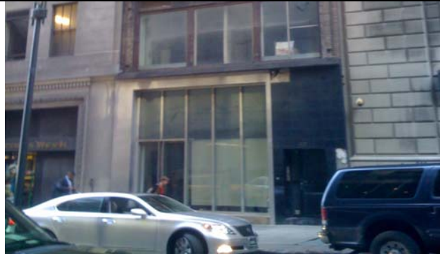
Existing Building to be Demolished at 47 East 44 th Street.
