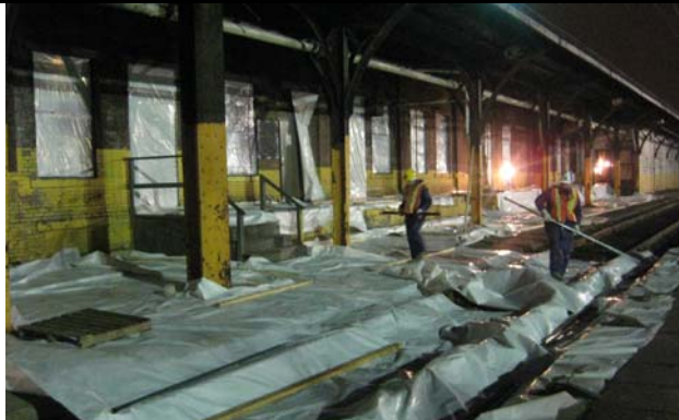
Asbestos Abatement of Canopy Along Amtrak Buildings.
