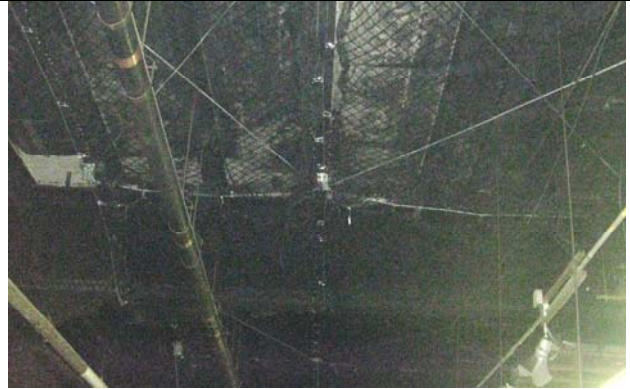
Netting Installation at Platform R.
