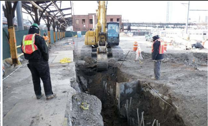
Exposing Top of Slurry Wall at Launch Shaft Area.
