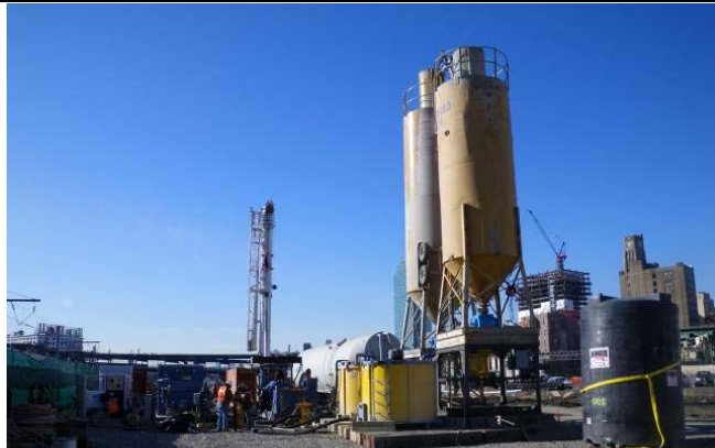
Mobilized Jet Grouting Equipment.
