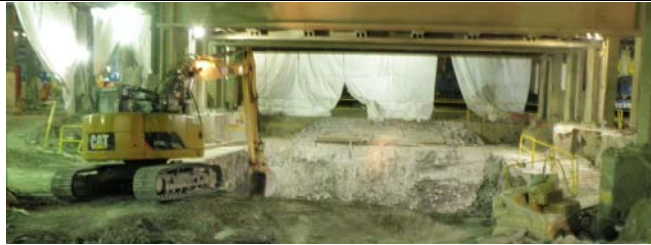
Mucking out at Wellway #4.
