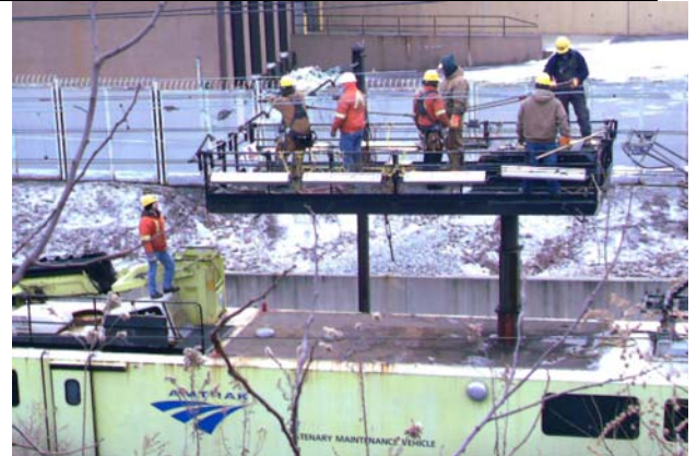
Relocating Catenary Wires at Loop Track.
