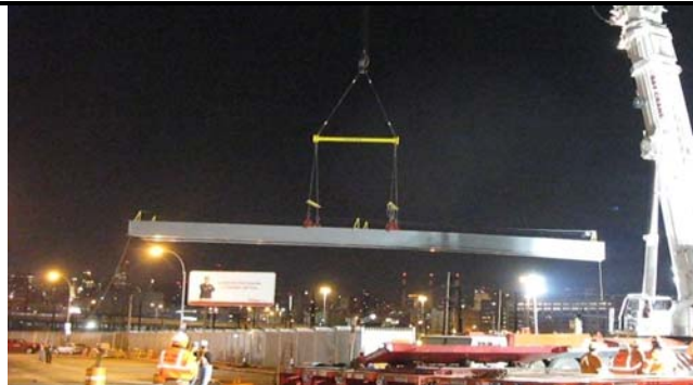
Installing Harold Access Bridge Girder.
