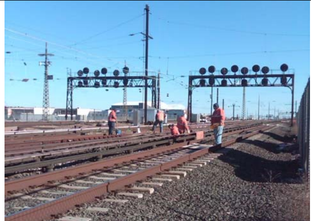
Install Conduit for 865 Crossover.
