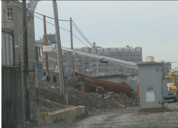
Relocate Communications Poles Along Skillman Ave.
