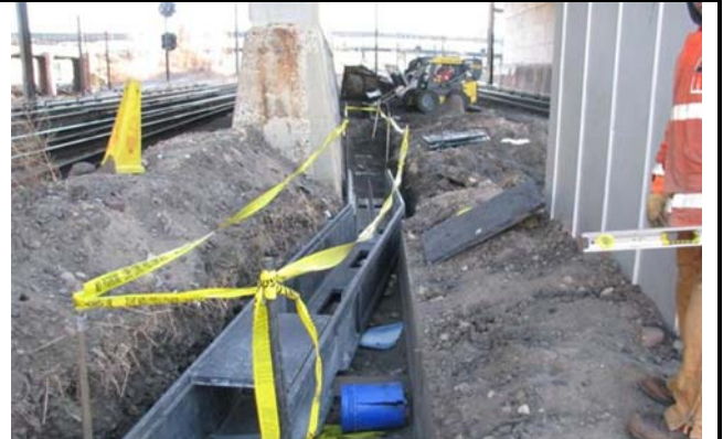
Trough Installation under Thomson Ave. East of Point CIL.
