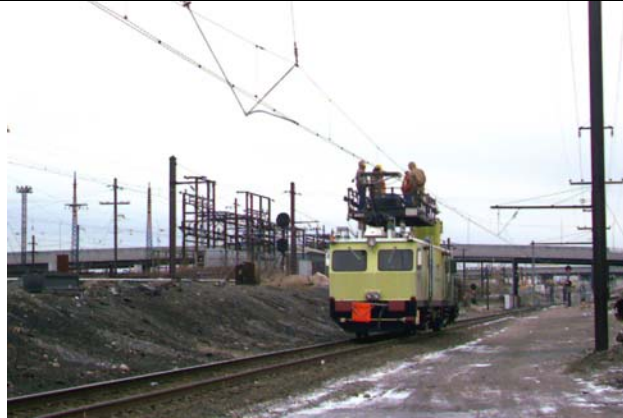
Relocating Catenary Wires at Loop Track.
