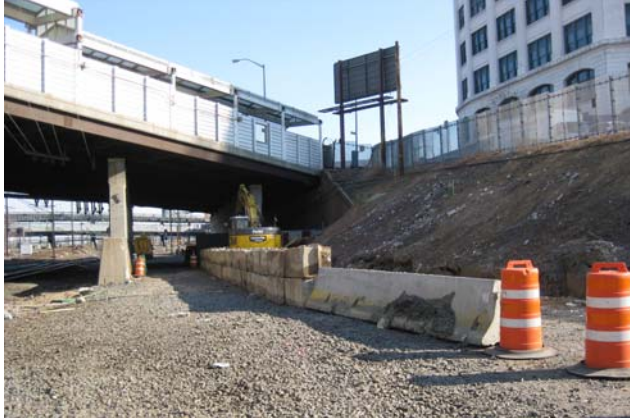
Construction Area for Retaining Wall THOM-S1.
