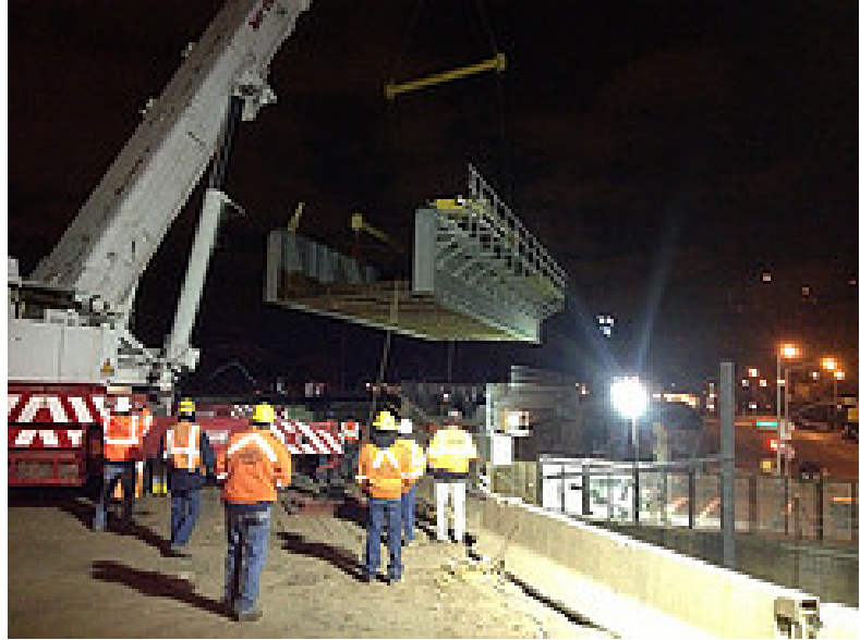
Installation of bridge span that will support eastbound tracks
