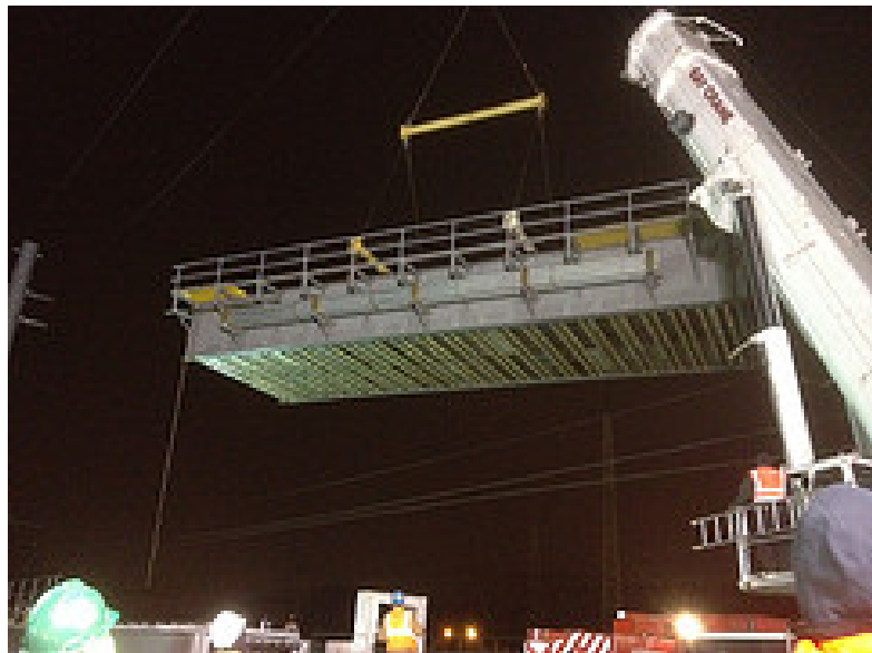
Installation of Westbound Bypass bridge span
