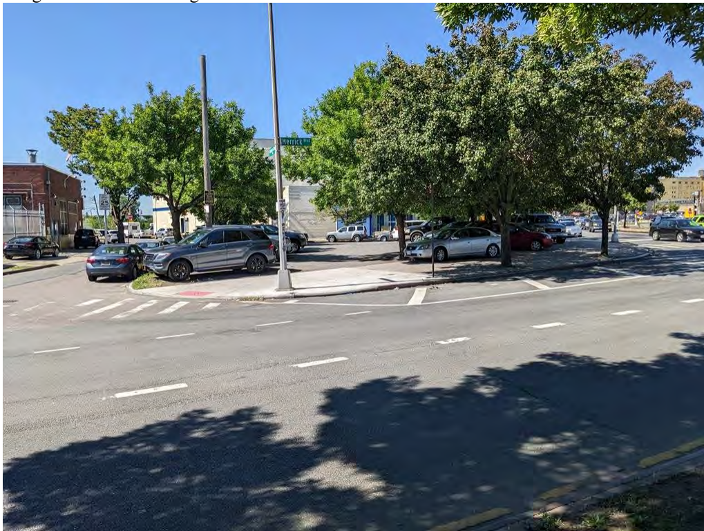
Photograph 16. The roadbed island portion of the project site, at the intersection of Merrick Boulevard (foreground) Tuskegee Airmen Way (left), and Liberty Avenue (right). View looking southwest.
