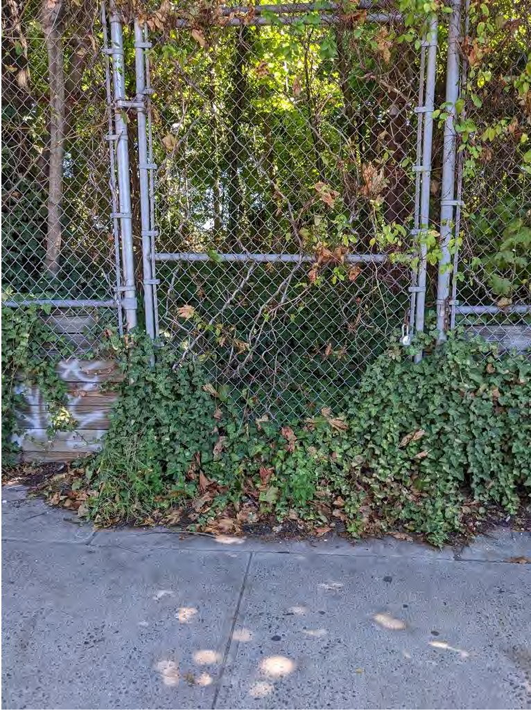
Photograph 10. The gate to the First Methodist Church of Jamaica historic cemetery from Guy R. Brewer Boulevard. There are stone steps leading from the sidewalk to the level of the cemetery. Note the wood retaining walls on either side of the gate. View looking northeast.
