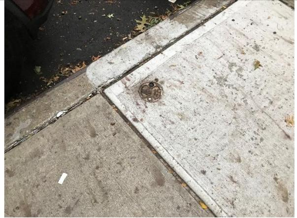
Photo 8: View of monitoring well observed on the southern sidewalk of West 28th Street.
