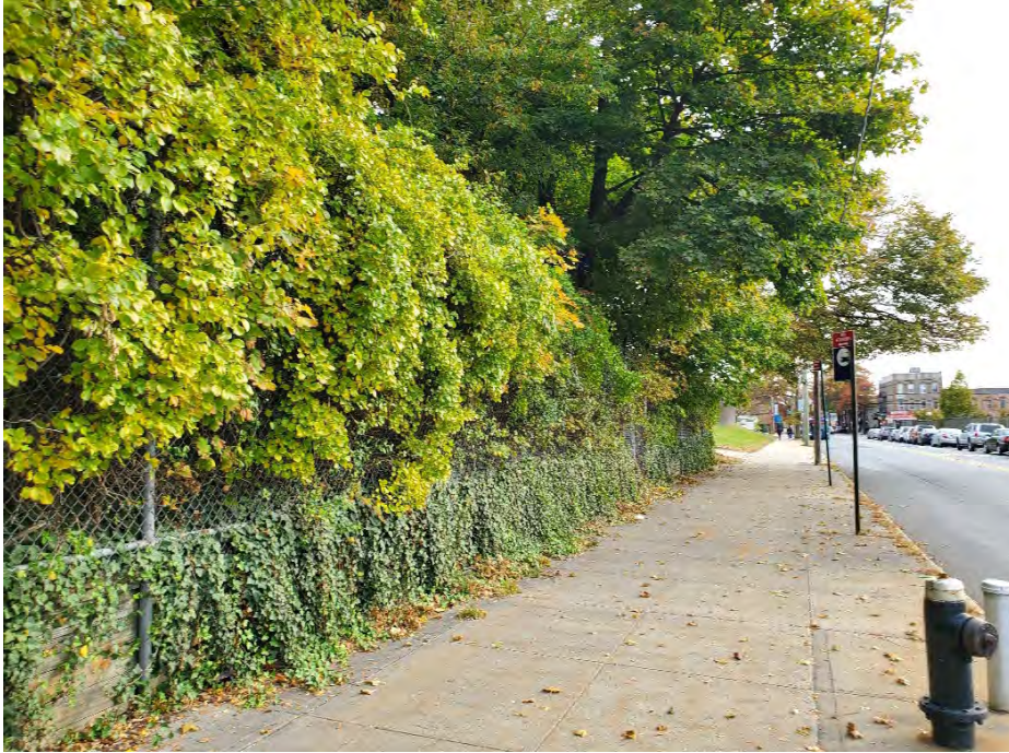
Photo 10: View facing south along Guy R. Brewer Boulevard between Liberty Avenue and Tuskegee Airmen Way. The Methodist Cemetery is located on the left but is obscured by overgrowth and chain-link fencing.
