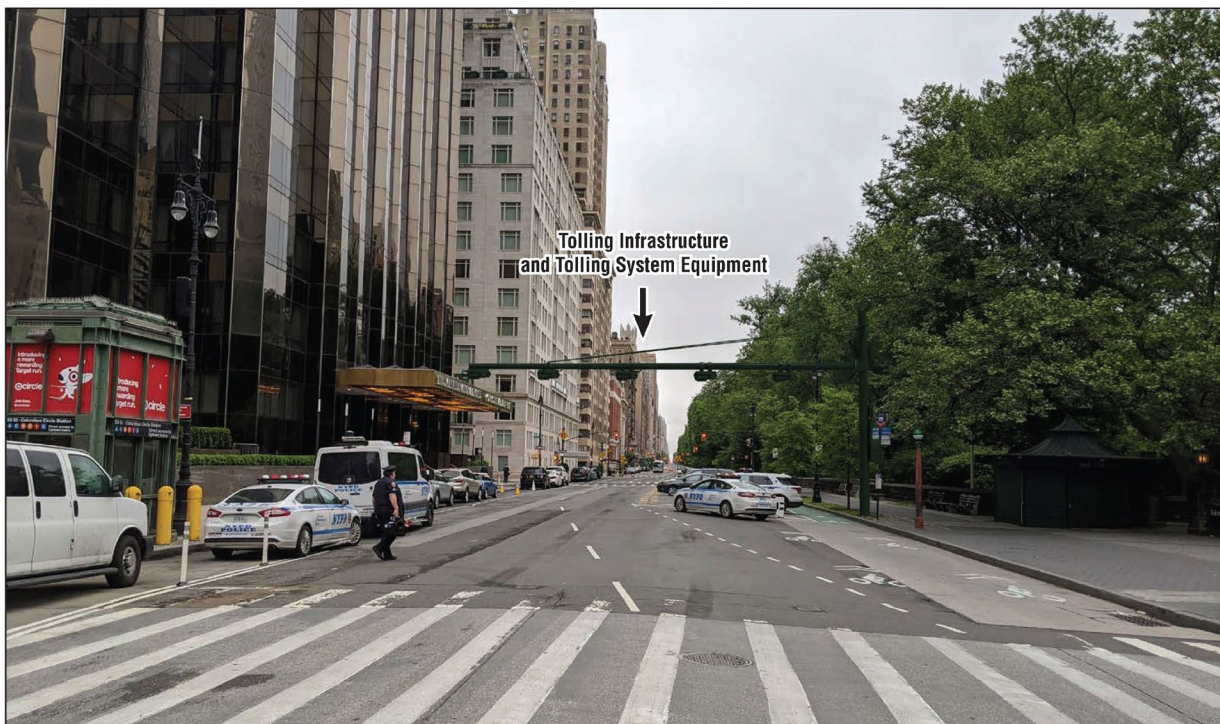
CBD Tolling Alternative, view north
