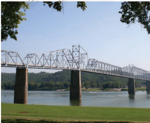
Milton Madison Bridge over the Ohio River between Kentucky and Indiana. Bridge projects can affect a variety of cultural and historic properties. (photo courtesy Wilbur Smith Associates/Michael Baker Engineers)
