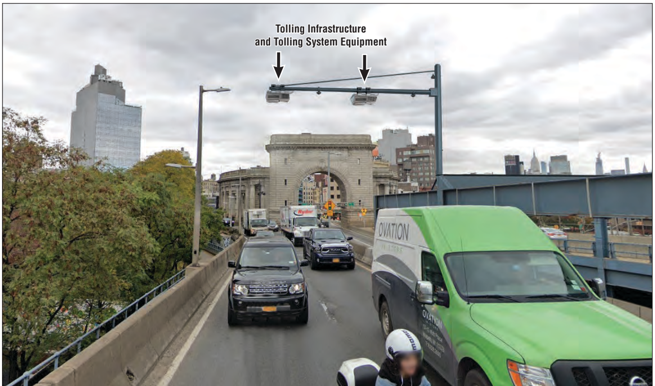
CBD Tolling Alternative, view west
