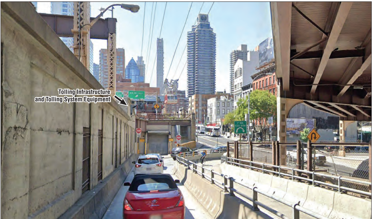
CBD Tolling Alternative, view west
