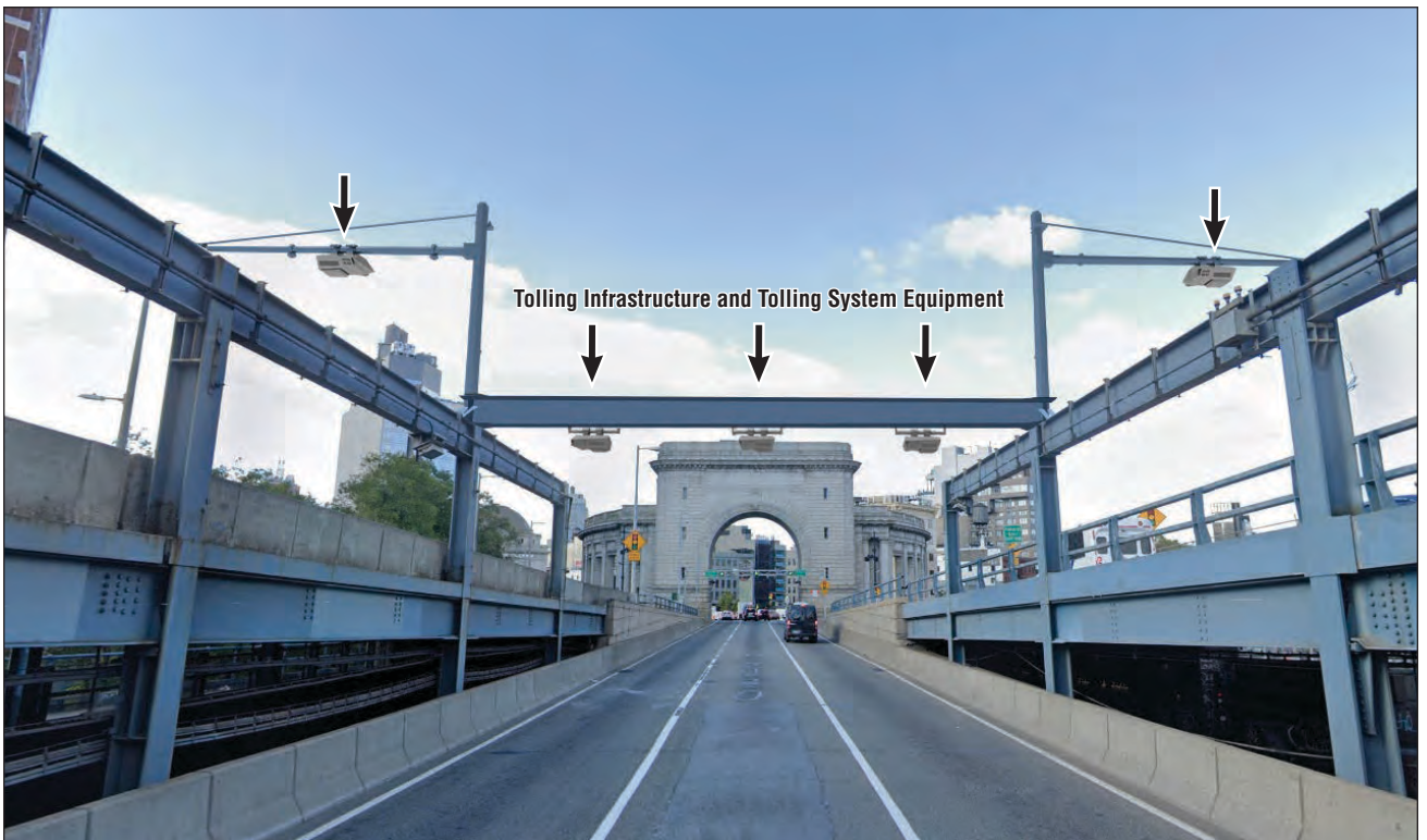
CBD Tolling Alternative, view west
