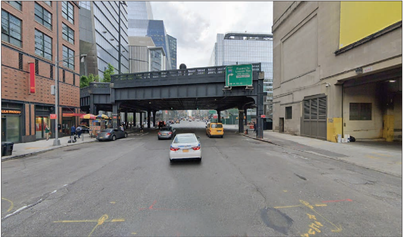
No Action Alternative, view north on Tenth Avenue
