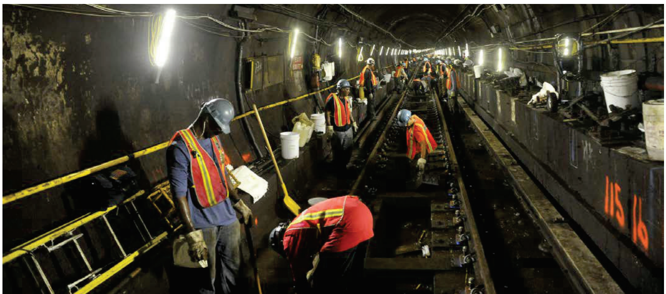
Figure 7: Post-Sandy Reconstruction on the MTA's Greenpoint Tubes (G Line)
