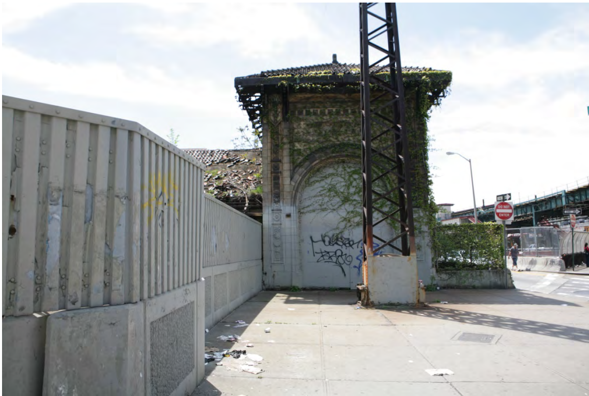
Photo 2. NYNH&H Railroad Westchester Avenue Station, Facing South, 2013
