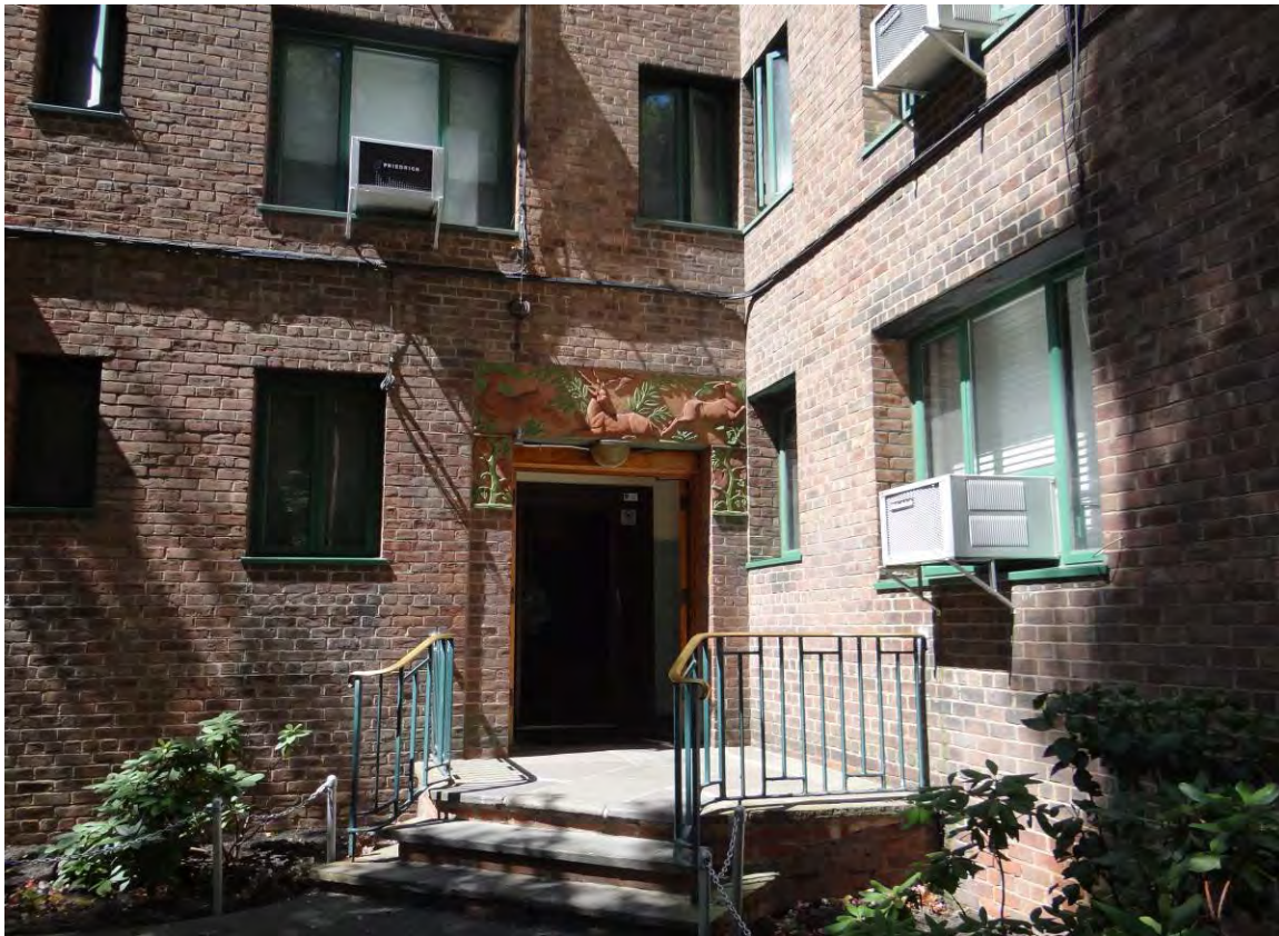
Photo 6. Parkchester, Typical Entrance and Replacement Windows, 2013
