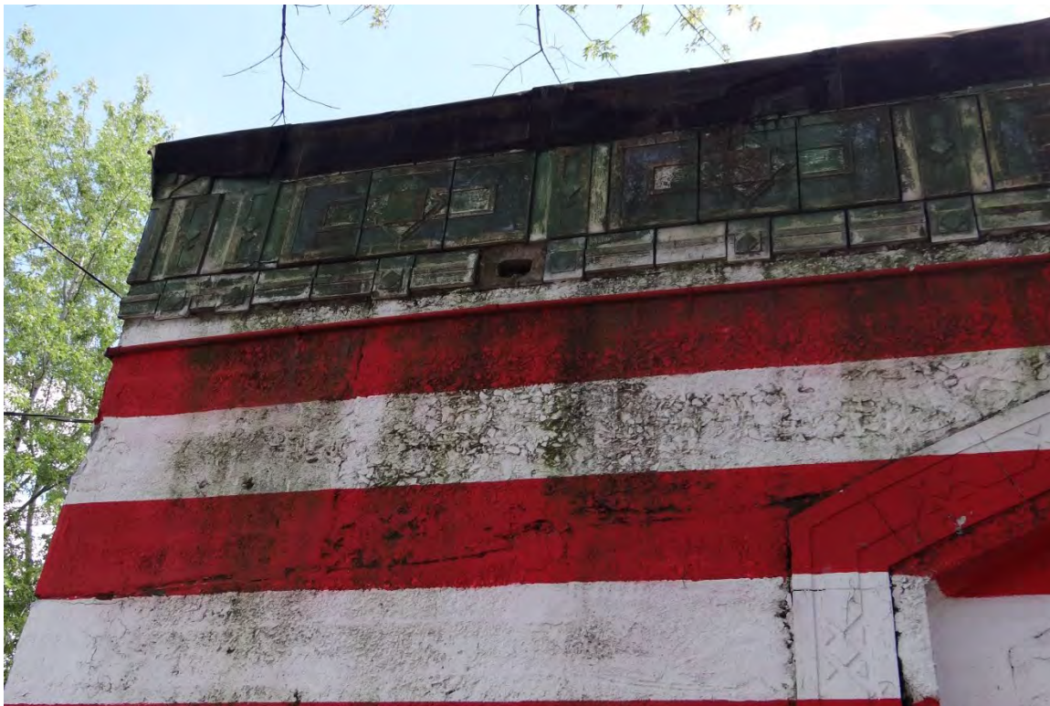
Photo 7. NYNH&H Railroad Morris Park Station, Facing South, 2013
