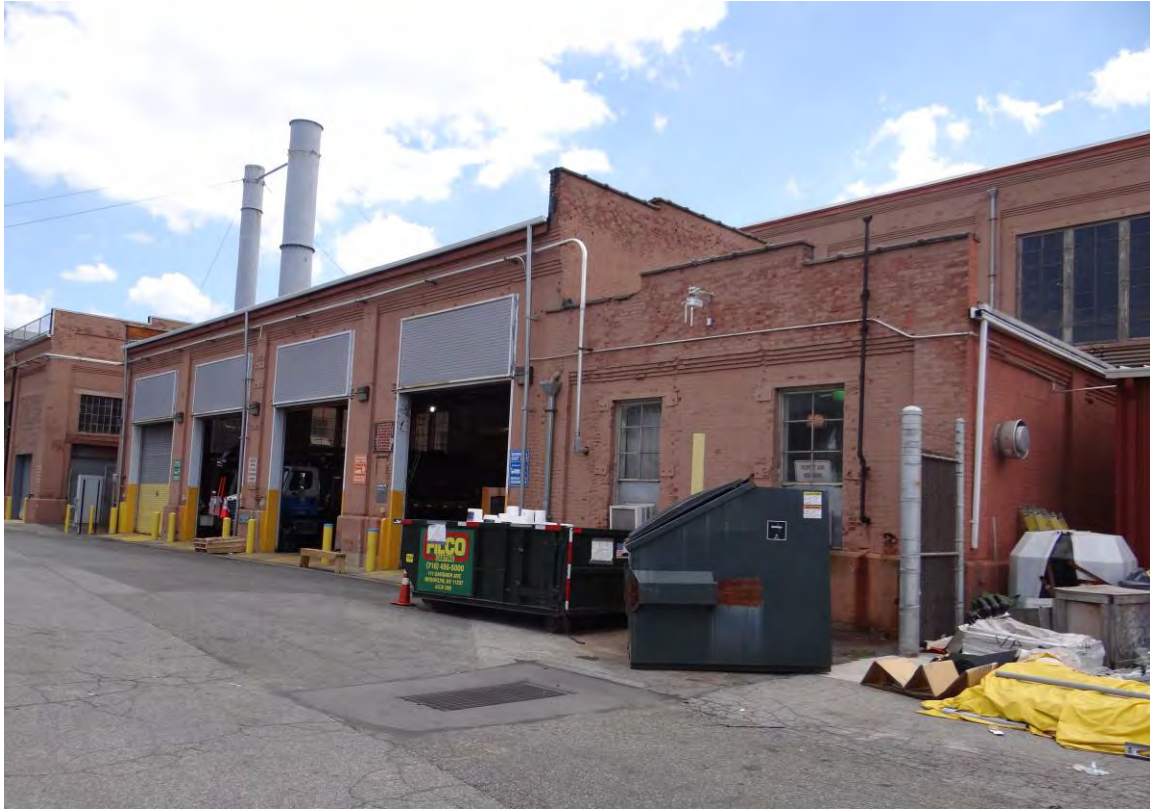
Photo 9. Former NYNH&H Railroad Van Nest Electric Locomotive Repair Shops. Former Cleaning Vat House and Blacksmith Shop, Facing East, 2013.
