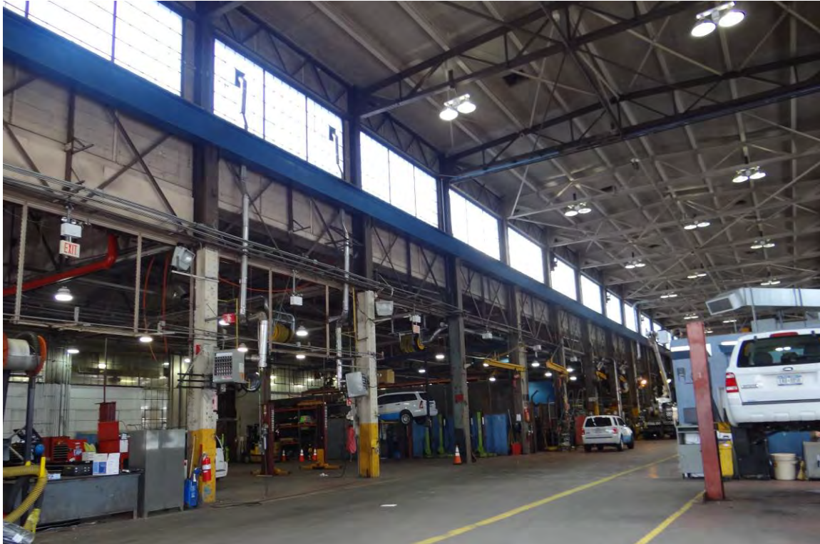
Photo 11. Former NYNH&H Railroad Van Nest Electric Locomotive Repair Shops. Interior, 2013.
