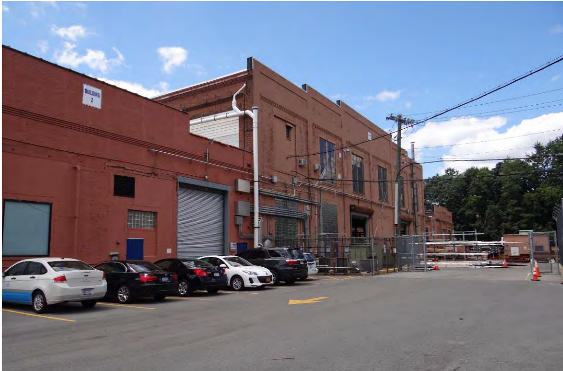
Photo 4. Former NYNH&H Railroad Van Nest Electric Locomotive Repair Shops, East Elevation, Facing Northwest, 2013
