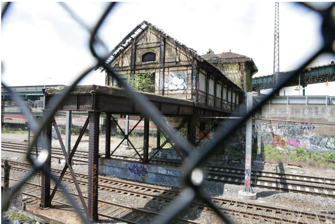
Photo 10. NYNH&H Railroad Westchester Avenue Station, Facing West, 2013
