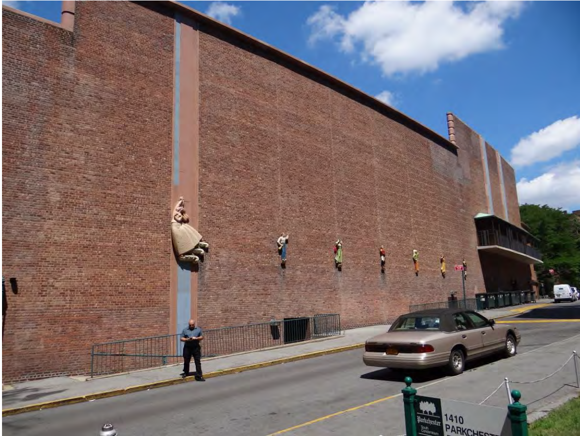
Photo 17. Parkchester, Terra Cotta Figures, Movie Theater Rear Elevation, 2013
