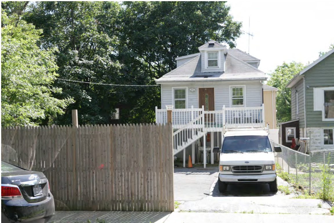
Photo 4. Modified Bungalow at 2227 Boller Avenue, June 2013
