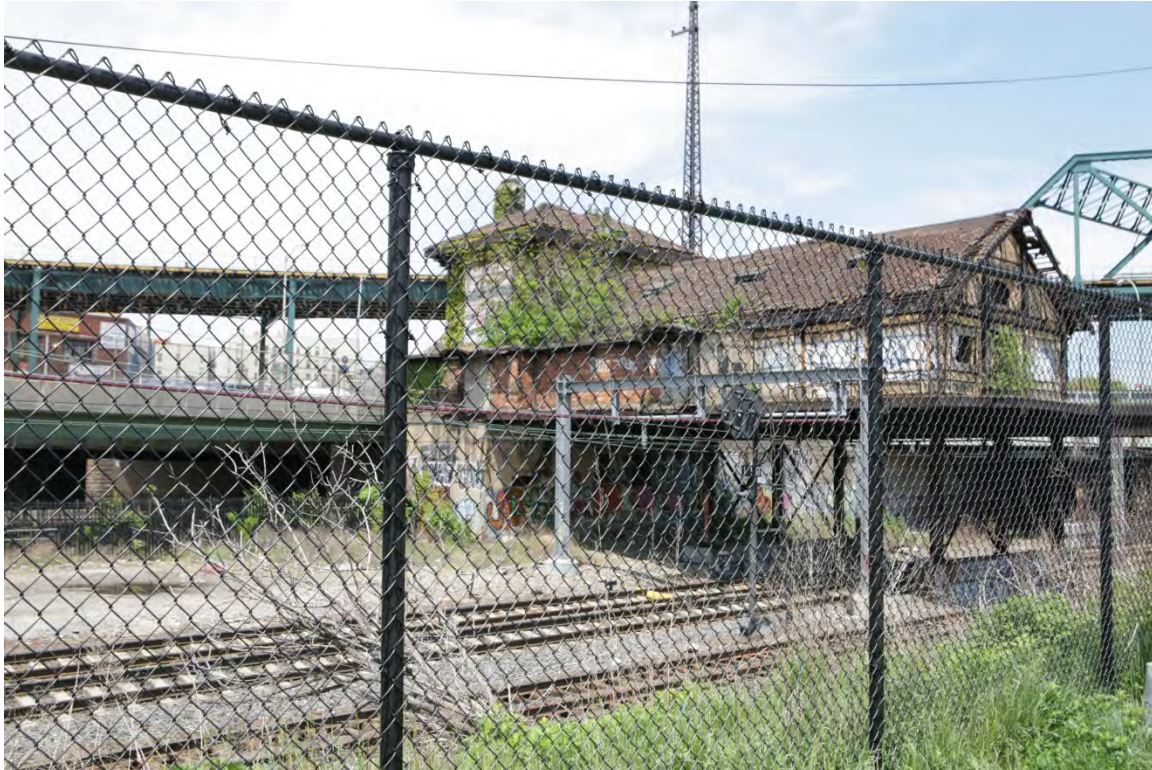
Photo 9. NYNH&H Railroad Westchester Avenue Station, Facing Northwest, 2013
