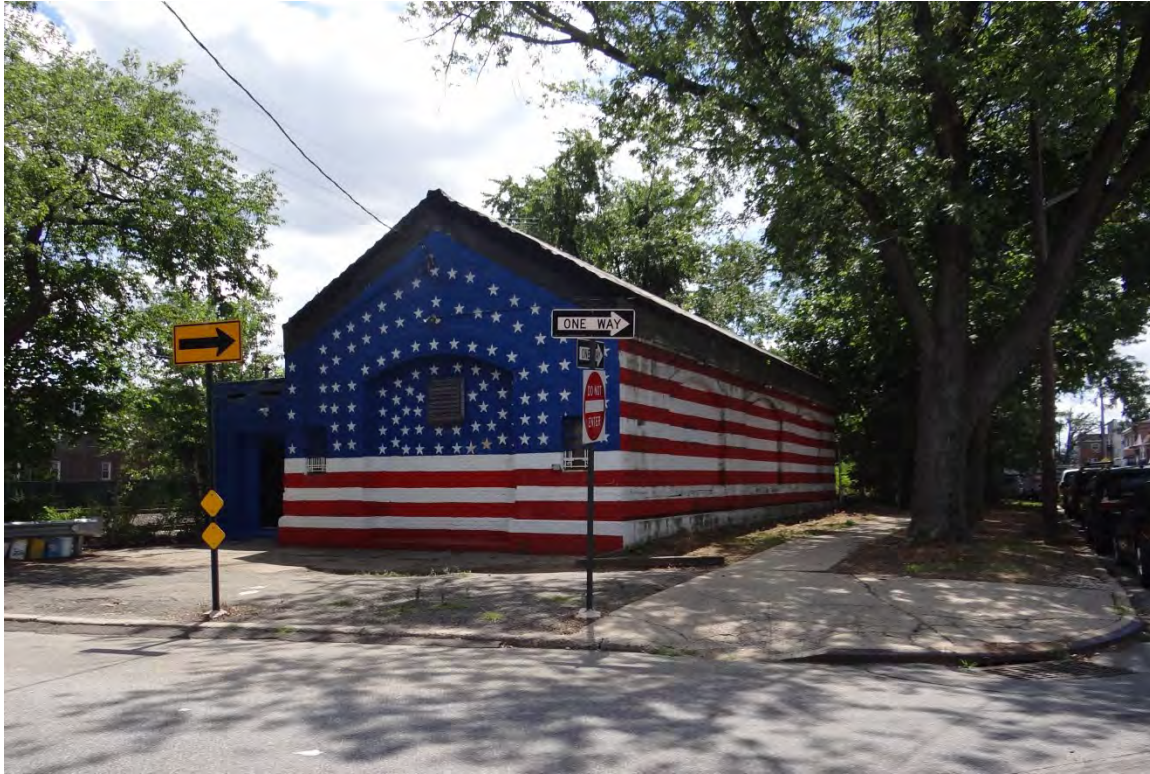
Photo 1. NYNH&H Railroad Morris Park Station, Facing Southwest, 2013
