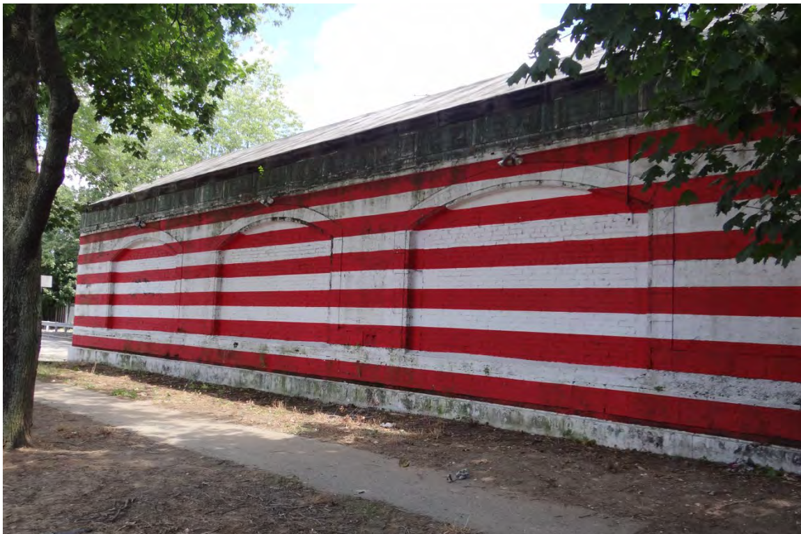
Photo 4. NYNH&H Railroad Morris Park Station, Facing Southeast, 2013
