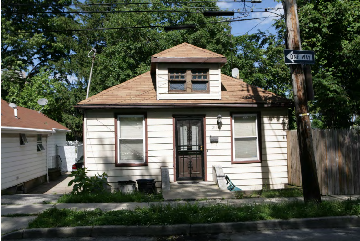
Photo 1. Baychester Village Bungalow, 2198 Palmer Avenue, Facing Northeast, June 2013
