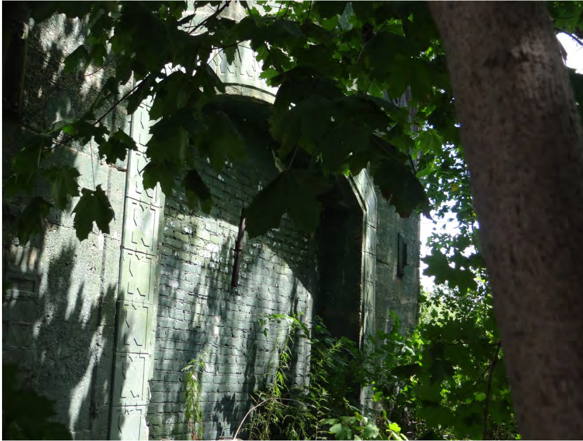
Photo 3. NYNH&H Railroad Morris Park Station, Facing Southeast, 2013
