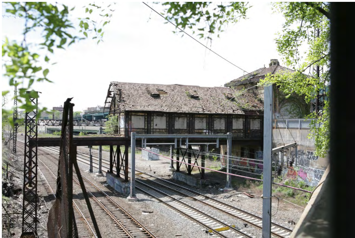
Photo 8. NYNH&H Railroad Westchester Avenue Station, Facing Southwest, 2013
