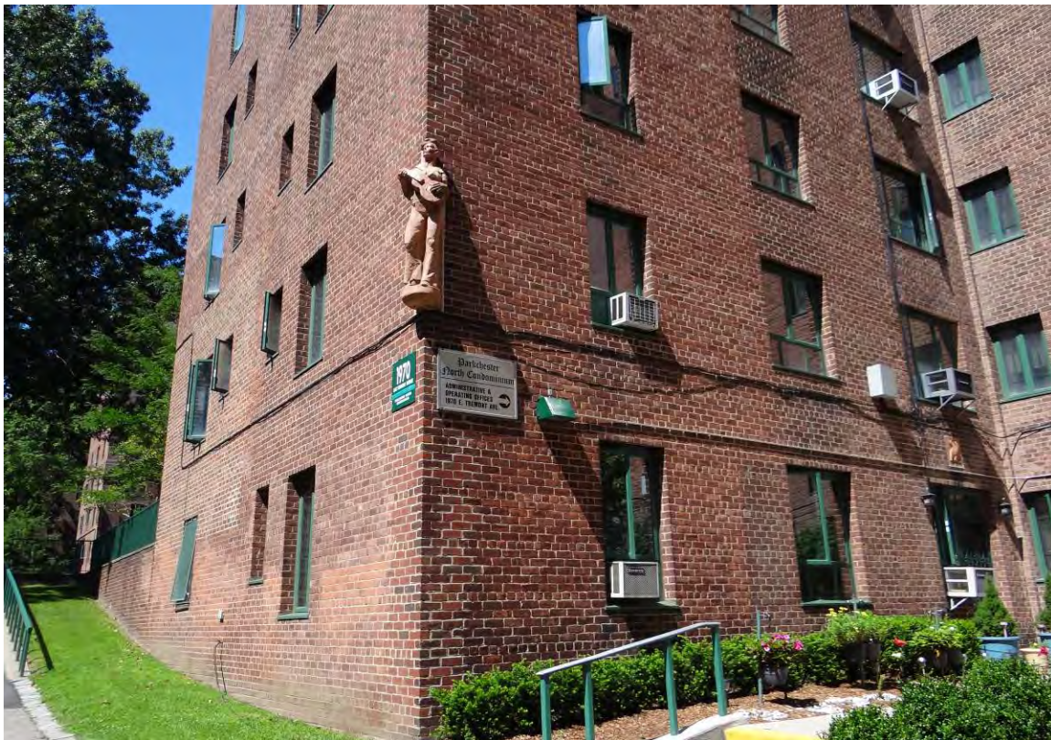
Photo 8. Parkchester, Replacement Windows, 2013
