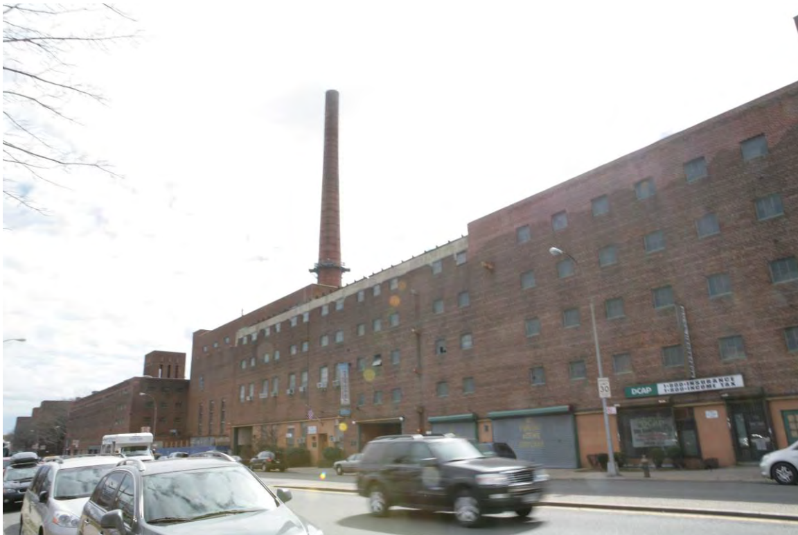
Photo 4. Parkchester, View from East Tremont Avenue, Facing Southeast, 2013
