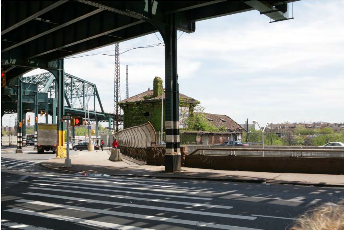
Photo 1. NYNH&H Railroad Westchester Avenue Station, Facing East, 2013
