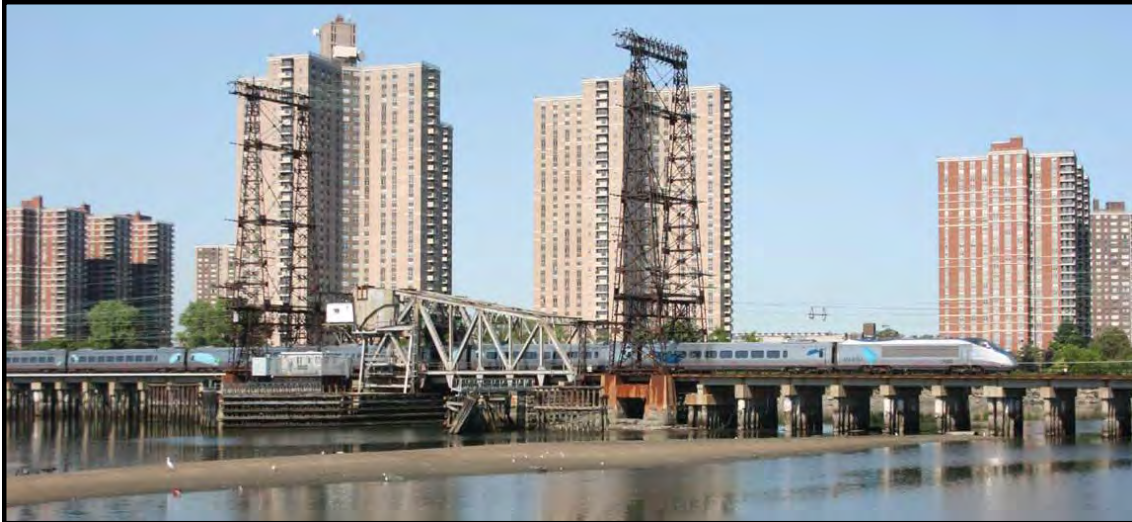
Photo 19. Amtrak Hell Gate Line (HGL) Bascule Bridge over Pelham Bay and Hutchinson River, View West. May 2013
