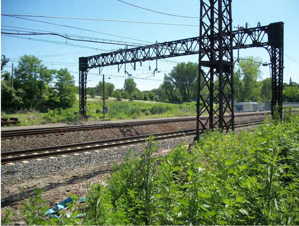
Photograph 5. Proposed Co-Op City Station project site south of Bruckner Expressway. Facing south from Erskine Place.
