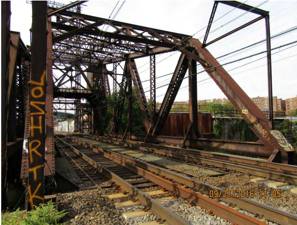
Bridge Deck Structural System – Looking Northwest
