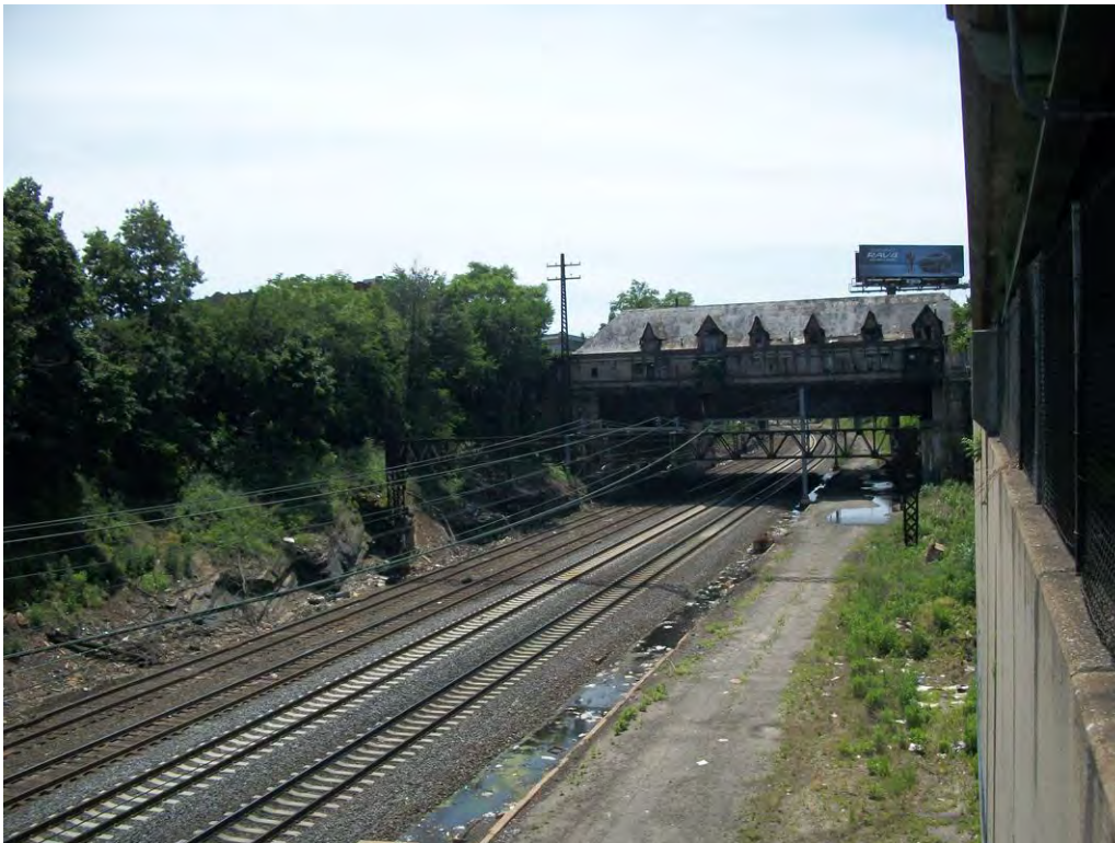
Photograph 6. Rear of extant train station over railroad right-of-way. Note that the tracks are depressed below the station and surrounding terrain. Facing south.
