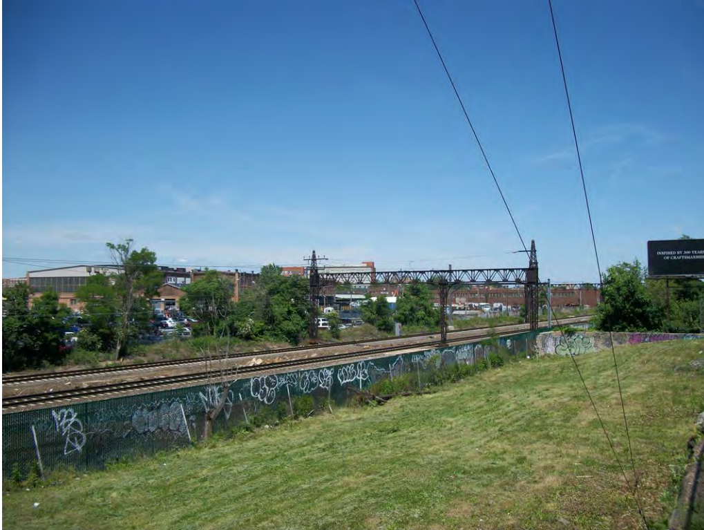
Photograph 3. View of existing track right-of-way and project site. Facing northeast from East Tremont Avenue.
