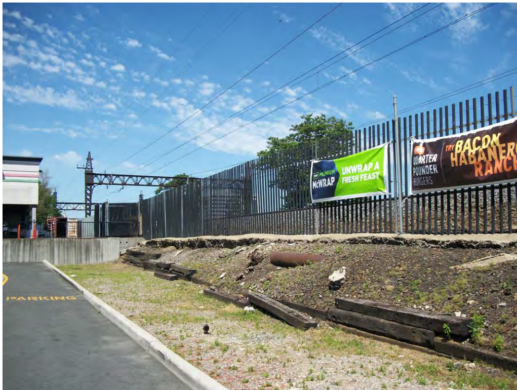
Photograph 5. Proposed Morris Park Station site. Facing northeast from rear of 1820 Eastchester Road.
