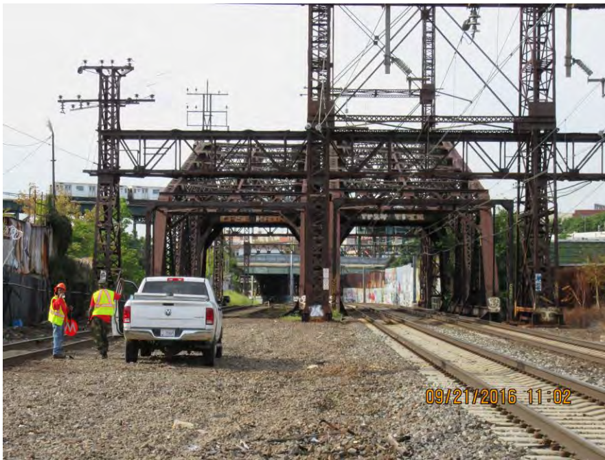
Elevation – Looking Backstation
