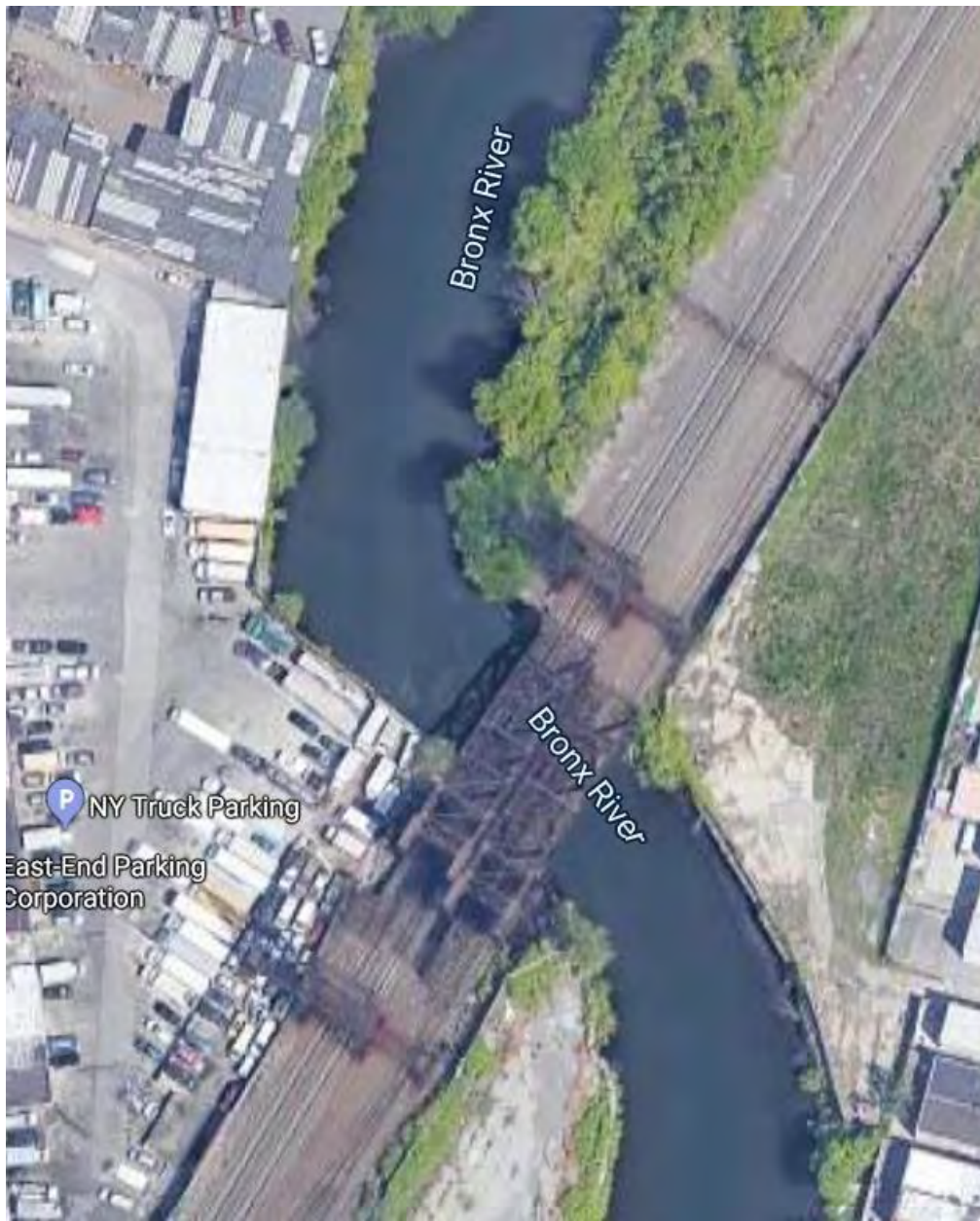
Photograph 1: Aerial photograph of extant Bridge #3.40, the extant Bascule Bridge, over the Bronx River. The third span was located to the northwest of the extant bridge. Note the concrete bulkhead along both the north and south sides of the river (Google 1/10/2020).
