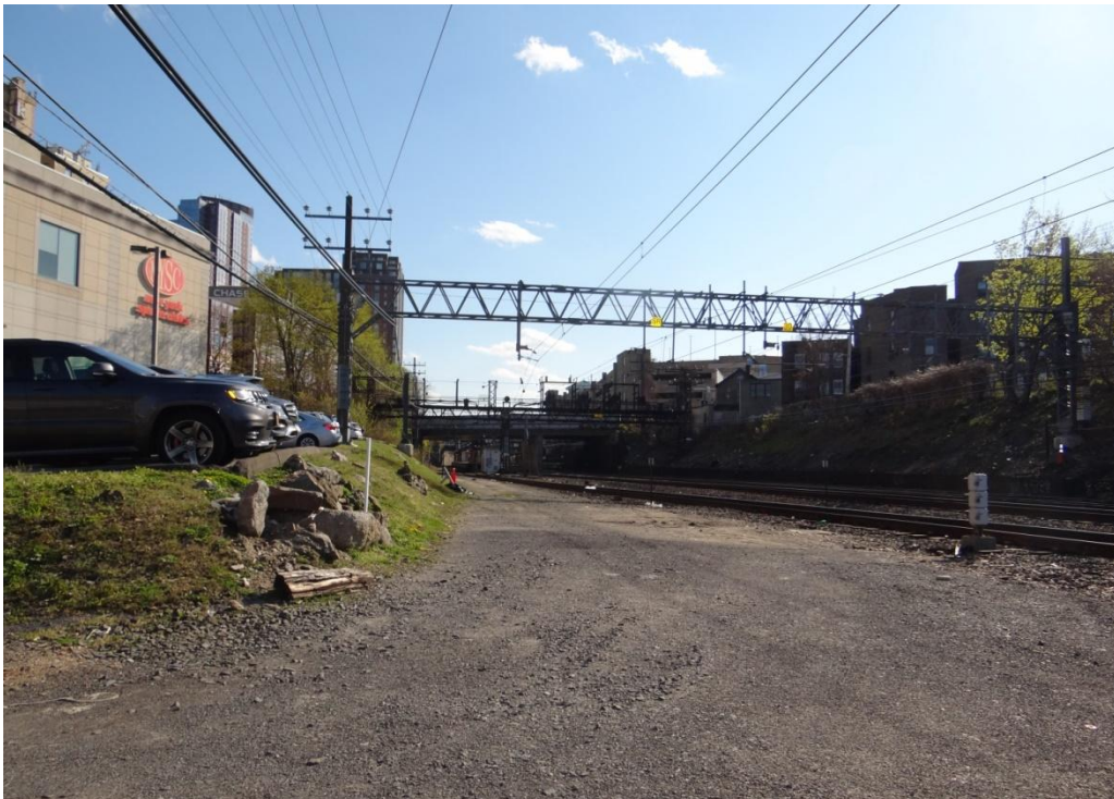
Source: Lynn Drobbin, 2020 Photo 12. New Rochelle Yard, Behind Trump Plaza, Facing South towards North Avenue
