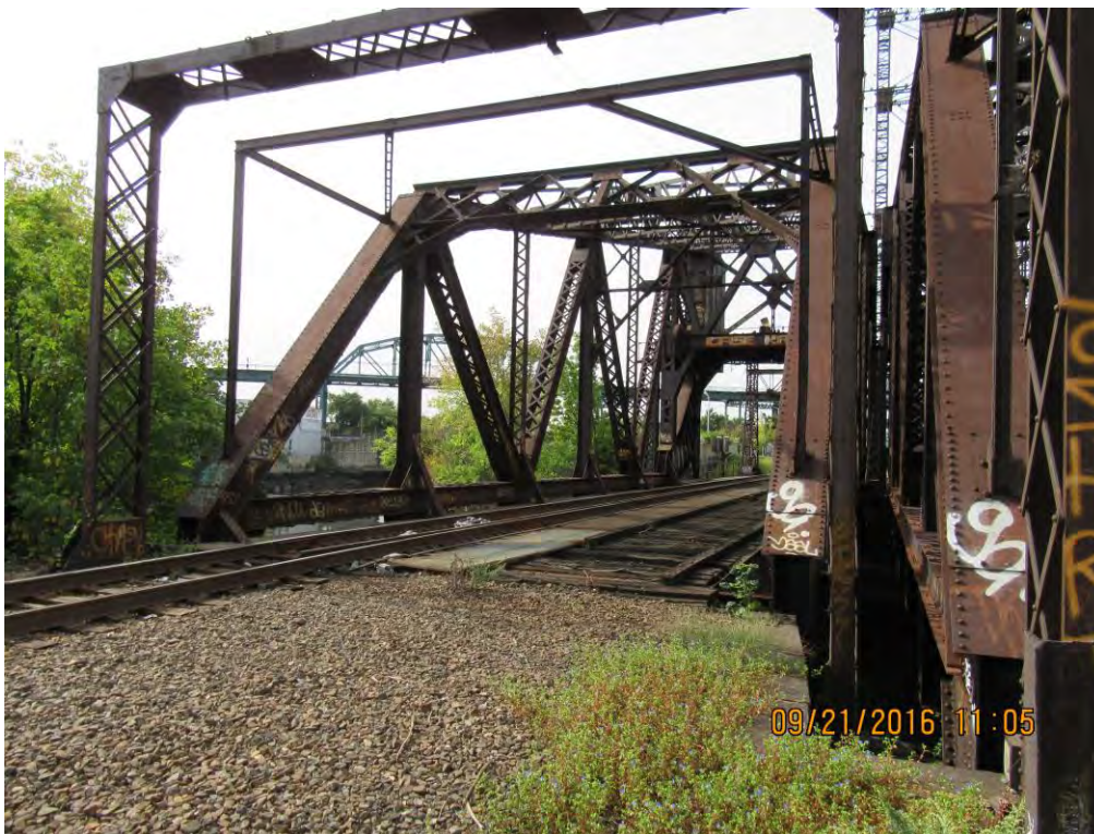
Bridge Deck Structural System – Looking Southwest
