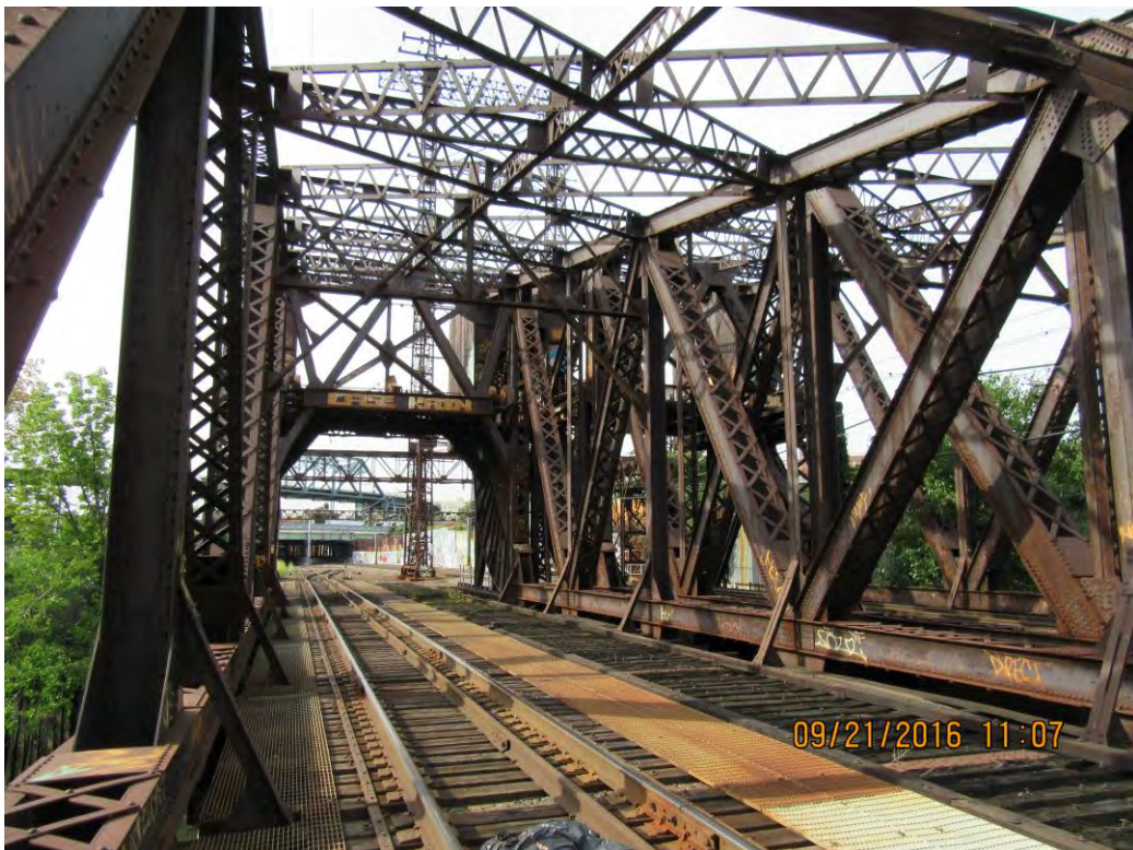
Bridge Deck Structural System – Looking West
