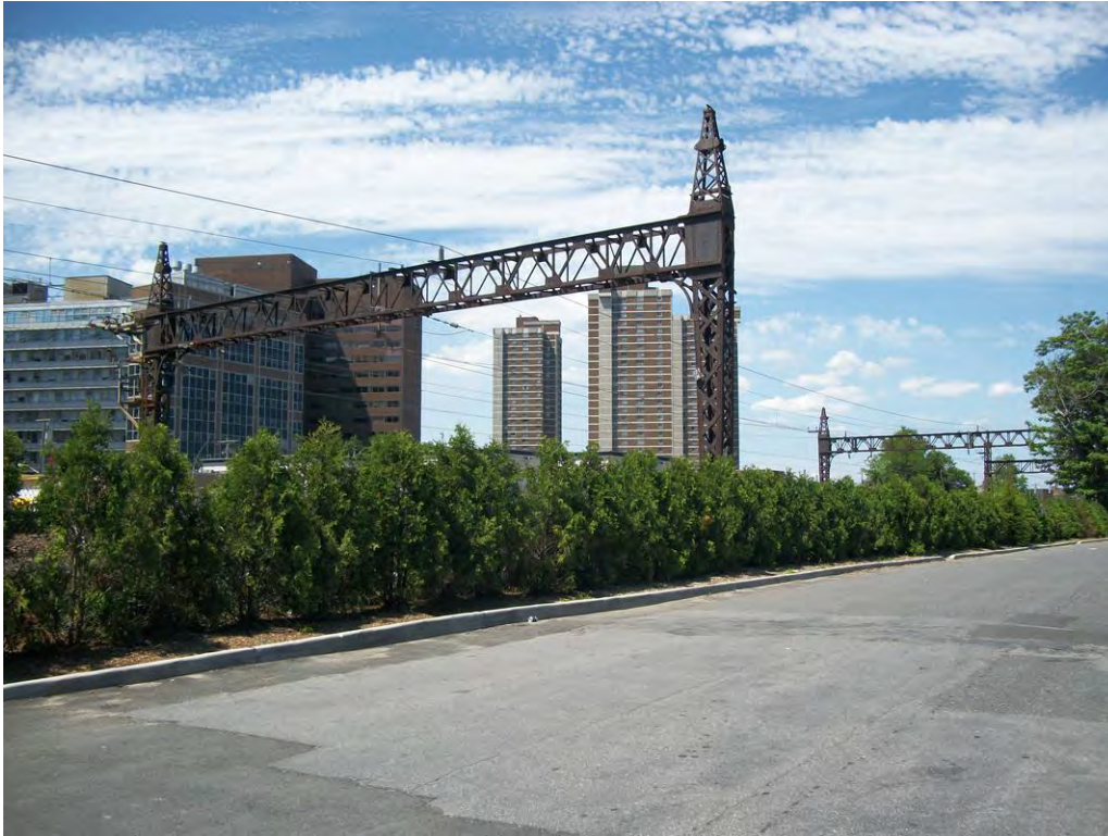
Photograph 1. Proposed Morris Park Station site. Facing north from Bassett Road.
