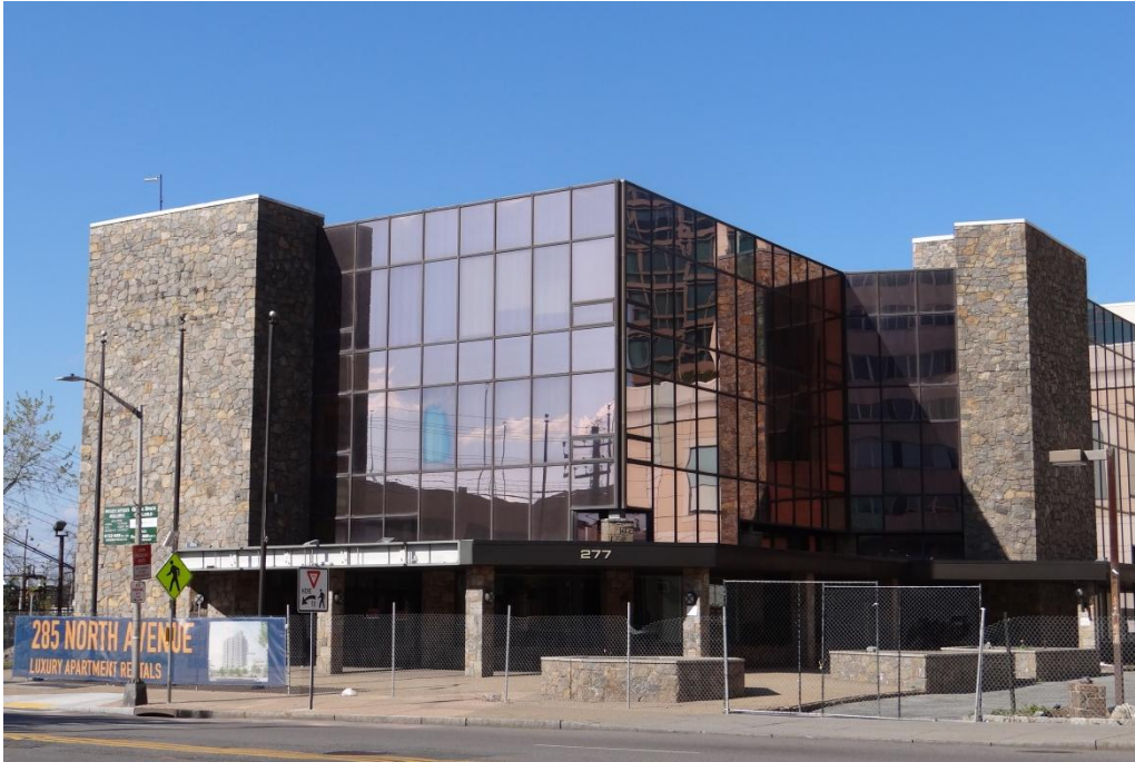
Source: Lynn Drobbin, 2020 Photo 37. 277 North Avenue, Facing Northwest
