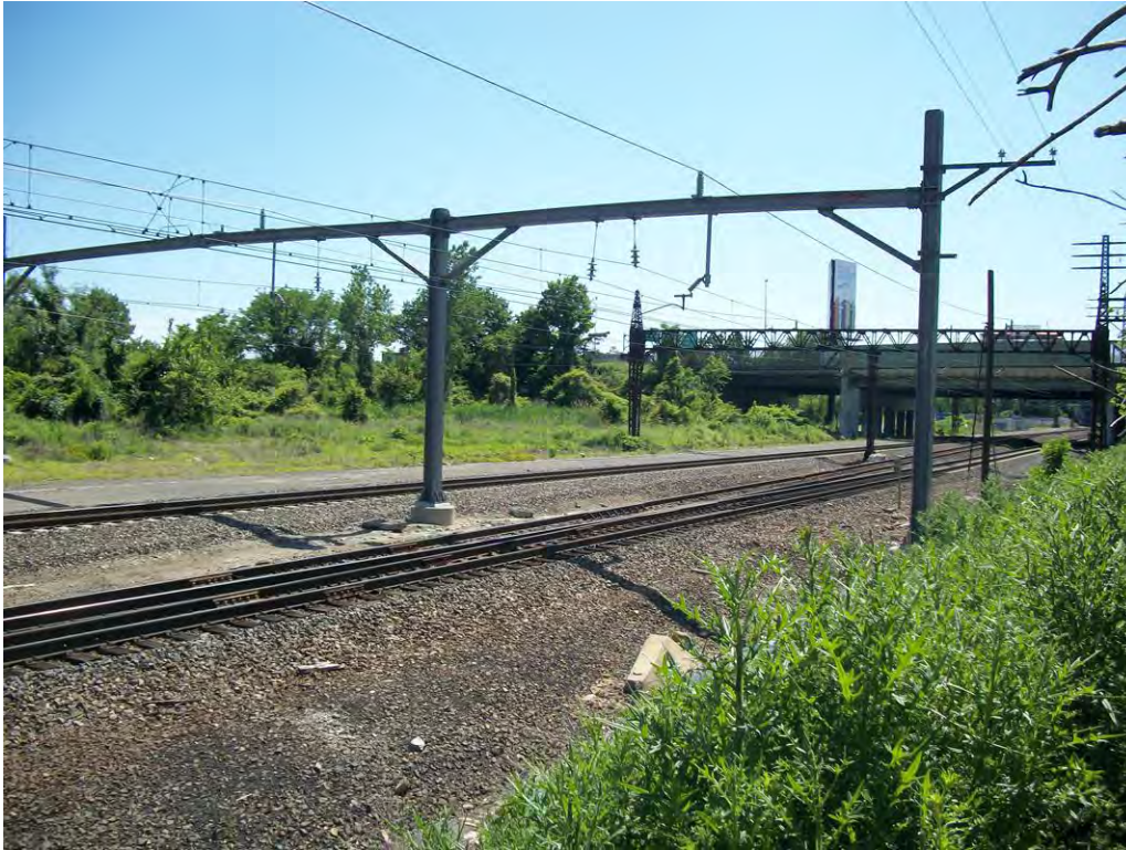
Photograph 1. Existing railroad tracks at proposed Co-Op City Station site. Facing southwest from Erskine Place.
