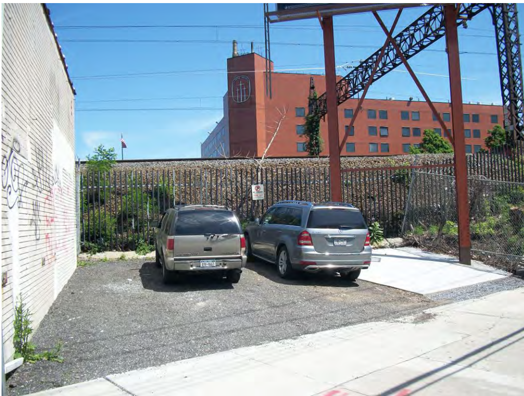
Photograph 4. Proposed Morris Park Station site showing existing railroad tracks on elevated embankment. Facing south from Eastchester Road.
