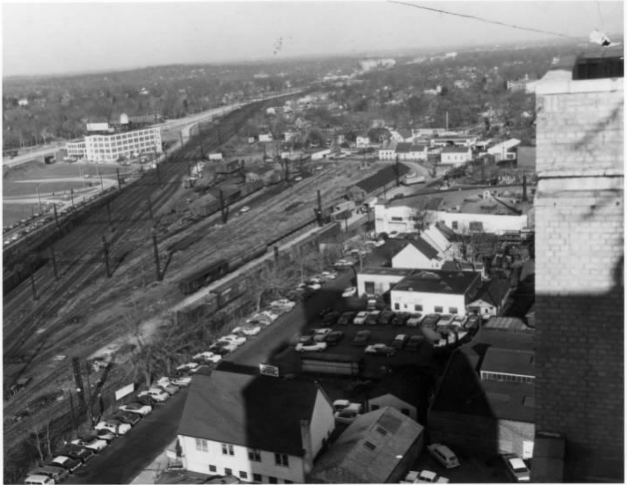
Credit: New Rochelle Public Library Local History Collection. Citation Guide: https://nyheritage.org/ Historic Photo 4. View of Freight Yard c.1955 from atop the "K" Building, Facing Northwest
