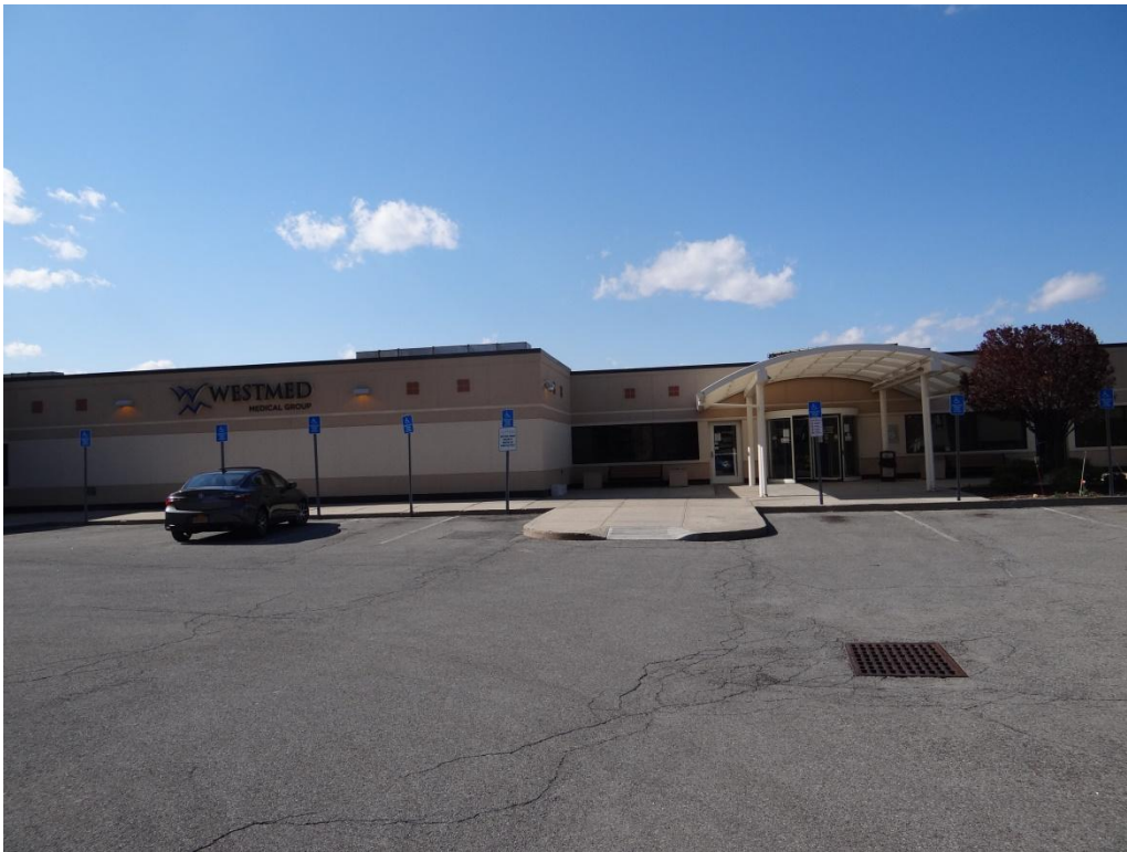
Source: Lynn Drobbin, 2020 Photo 38. WestMed Medical Office, Facing West
