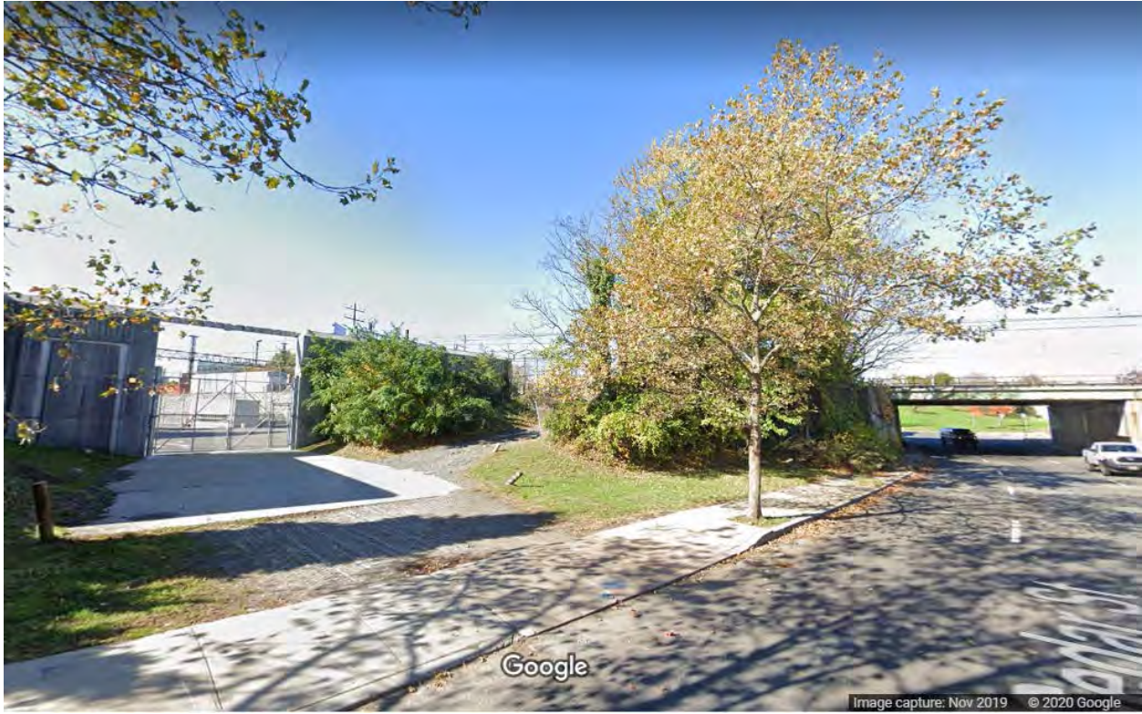
Photograph 5: Facing northwest from Cedar Street to substation (left) and railroad bridge (right). (Google 2019)
