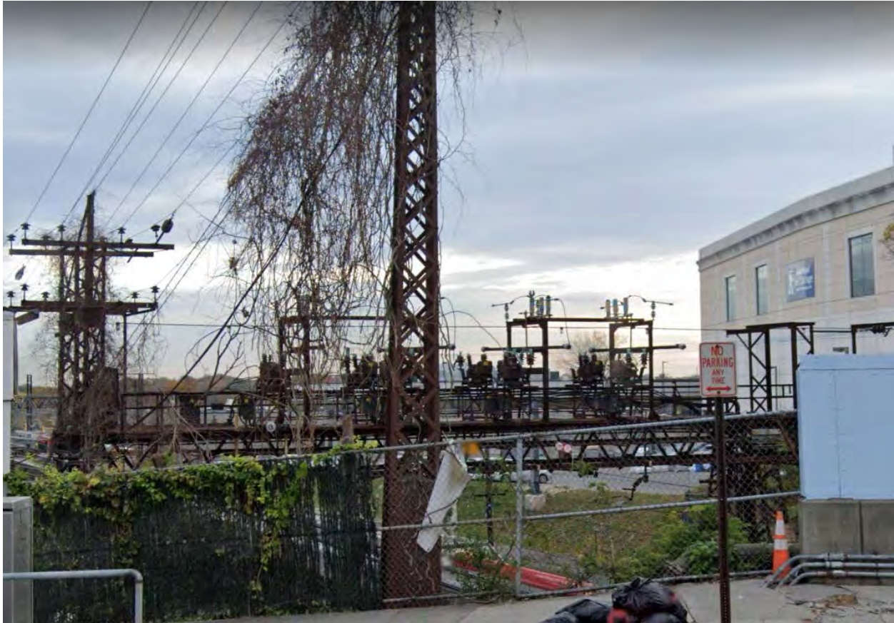
Photograph 1: Facing east from North Avenue Bridge over railroad tracks. (Google 2019)
