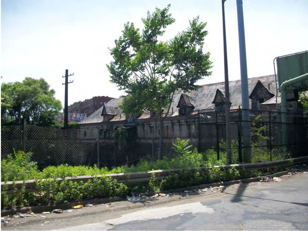
Photograph 7. Rear of extant Hunts Point Avenue train station with railroad tracks beneath the station. Facing south from Bruckner Expressway Ramp.
