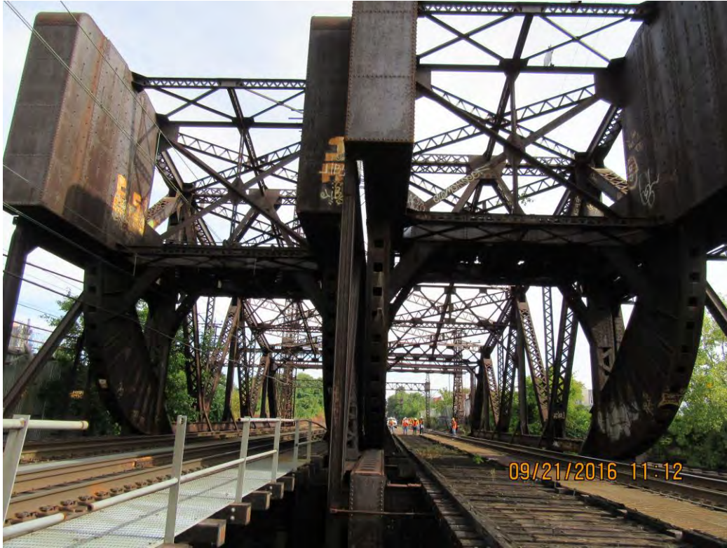
Bridge Deck Structural System – Looking East
