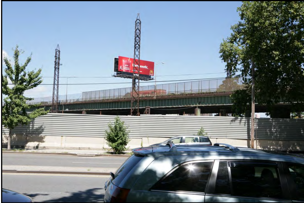
Photo 23. Cross Bronx Expressway (I-95) over Sheridan Expressway (I-895), Bronx River, Bronx River Avenue and Amtrak Hell Gate Line (HGL), View North. May 2013
