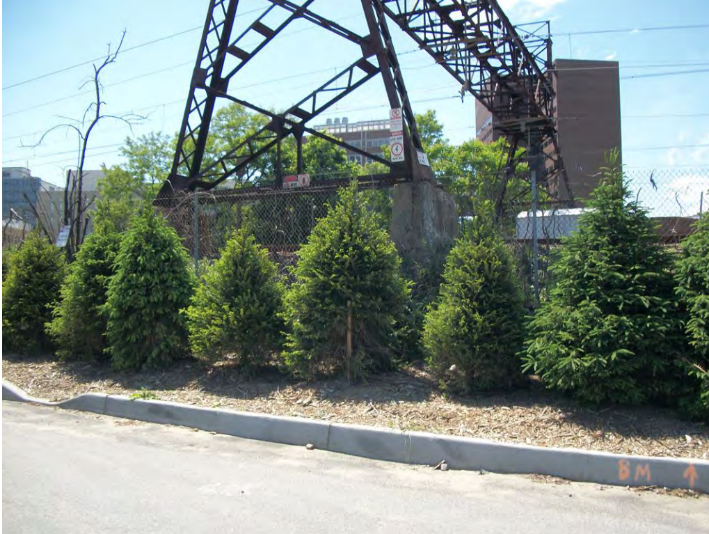
Photograph 3. Proposed Morris Park Station site. Facing west from Bassett Road.
