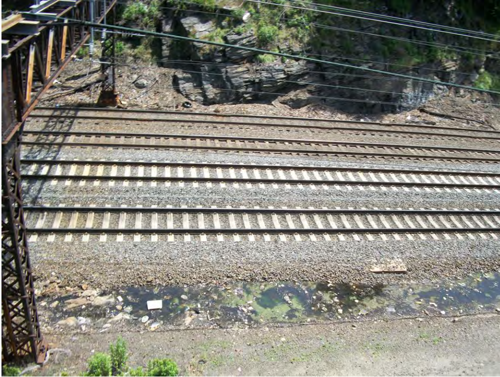
Photograph 3. Close-up of exposed bedrock cut and tracks at proposed Hunts Point Avenue Station Site. Facing east from west side of tracks.
