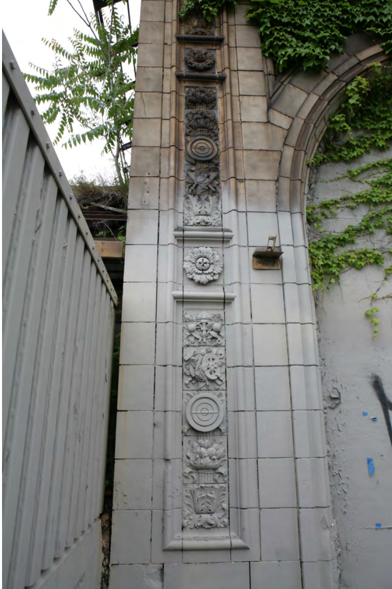
Photo 75. Terra Cotta Tile, Former NYNH&H Railroad Westchester Avenue Station, Detail, Facing South
