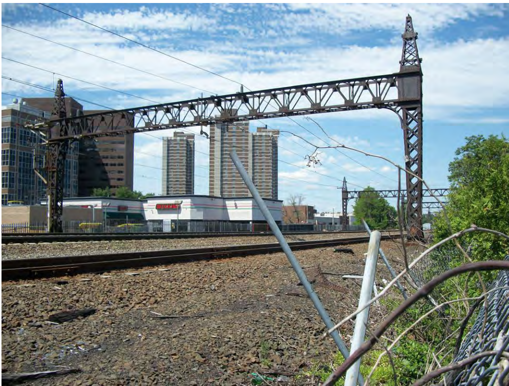
Photograph 2. Proposed Morris Park Station site. Facing north from Bassett Road.
