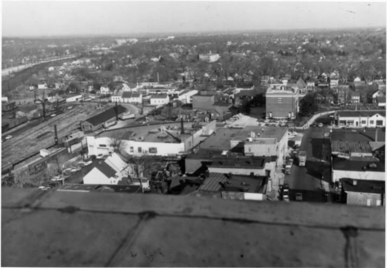
Credit: New Rochelle Public Library Local History Collection. Citation Guide: https://nyheritage.org/ Historic Photo 3. View of Rail Yard Atop "K" Building, Looking North, c.1950
