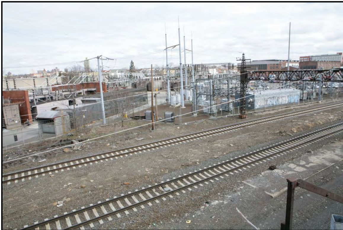
Photo 6. Existing Con Edison and Amtrak Substations, View North, March 2013
