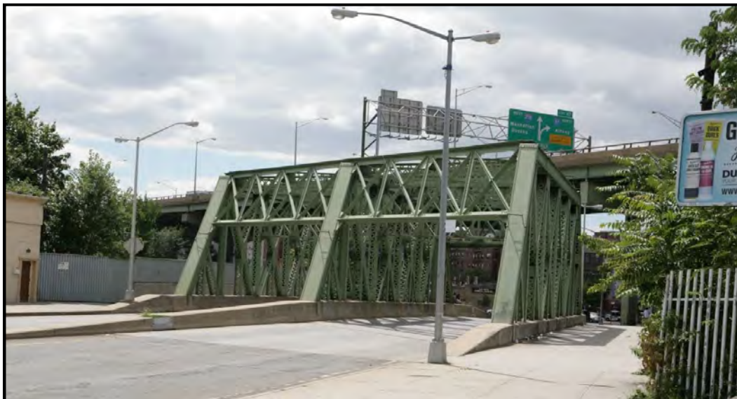
Photo 32. Lafayette Avenue Bridge over Amtrak HGL, View West, May 2013
