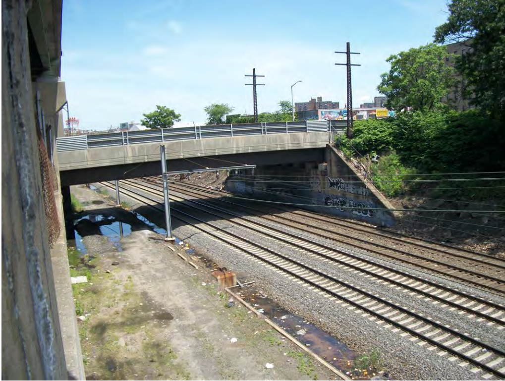
Photograph 5. Railroad cut. Facing northeast from Bruckner Boulevard toward Faile Street overpass.
