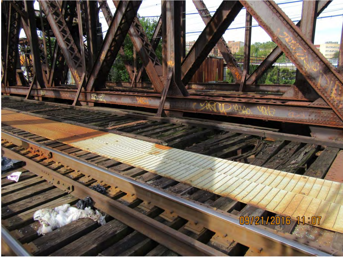
Bridge Deck Structural System – Looking Northwest
