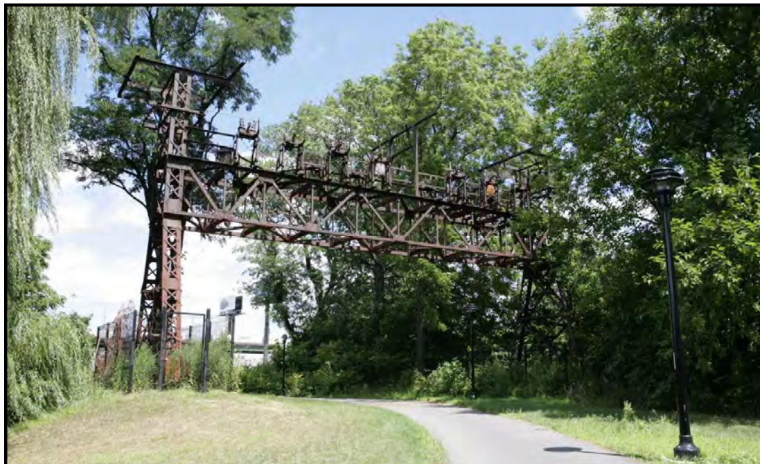
Photo 25. New York, Westchester & Boston Railway Anchor Bridge, View Northeast, May 2013
