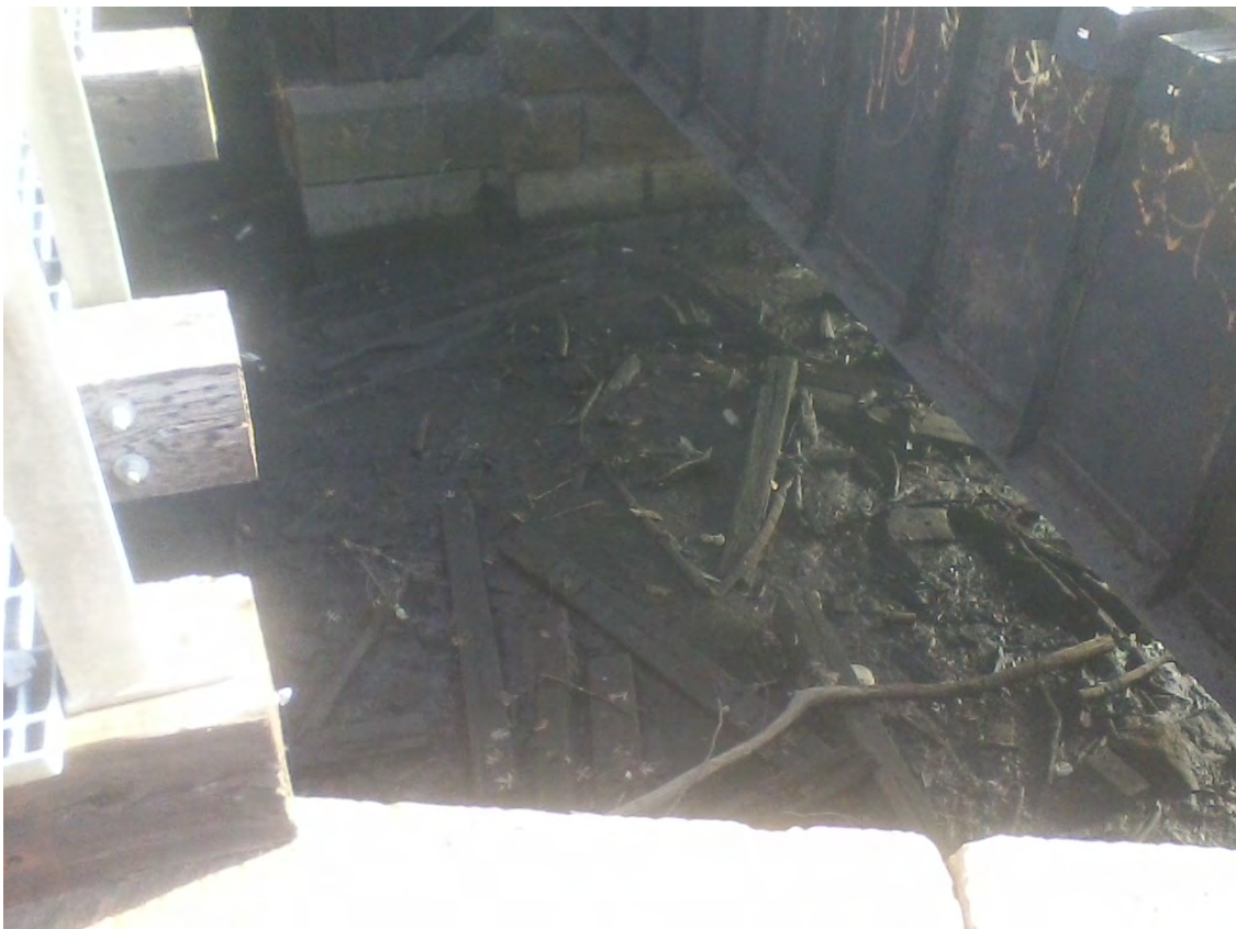
Photo 4 – Intertidal shoreline beneath existing drawbridge, low tide.
