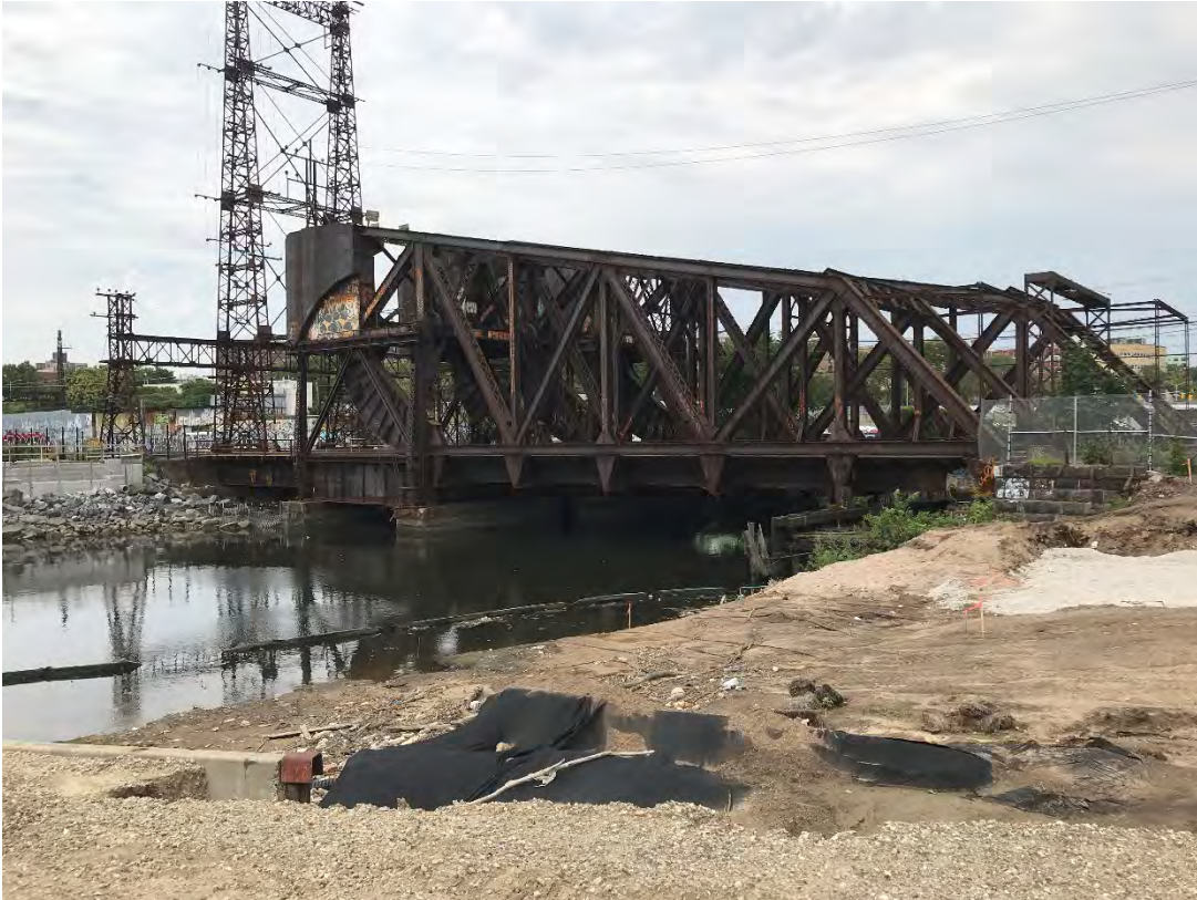
Photo 1 – Existing Amtrak Hell Gate Line drawbridge across the Bronx River.
