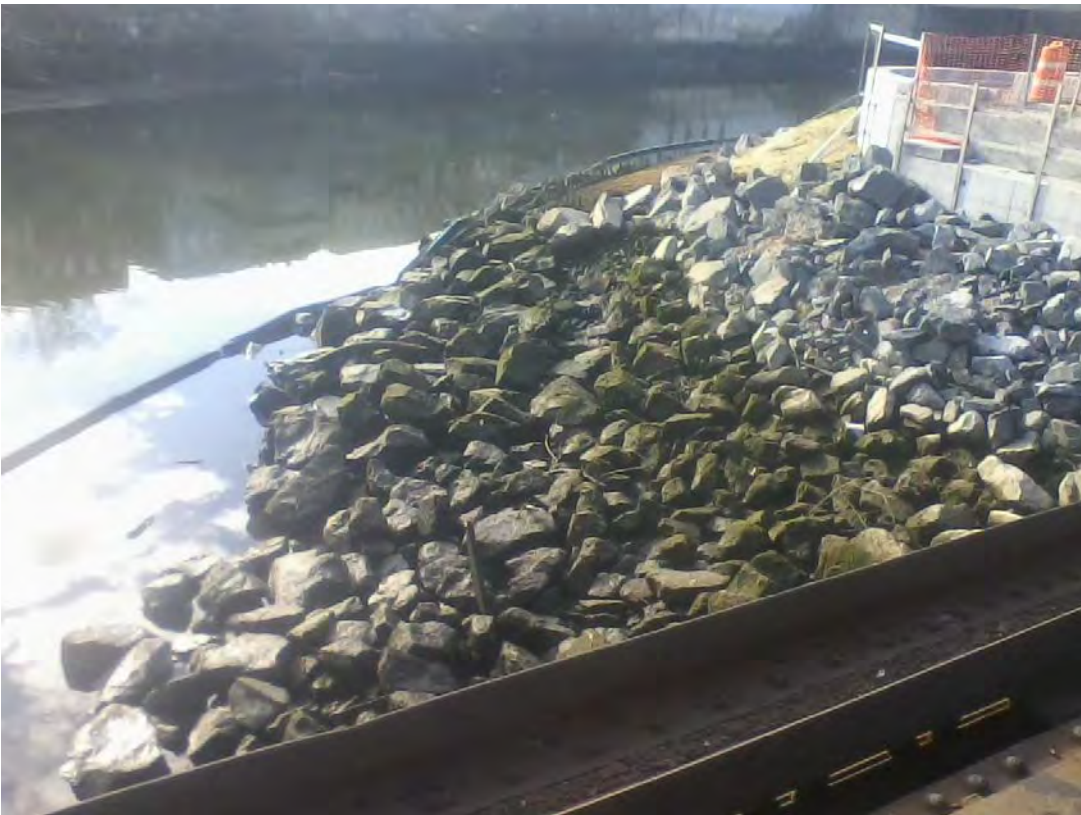
Photo 2 – Rip-rap along shoreline on west side of existing drawbridge.
