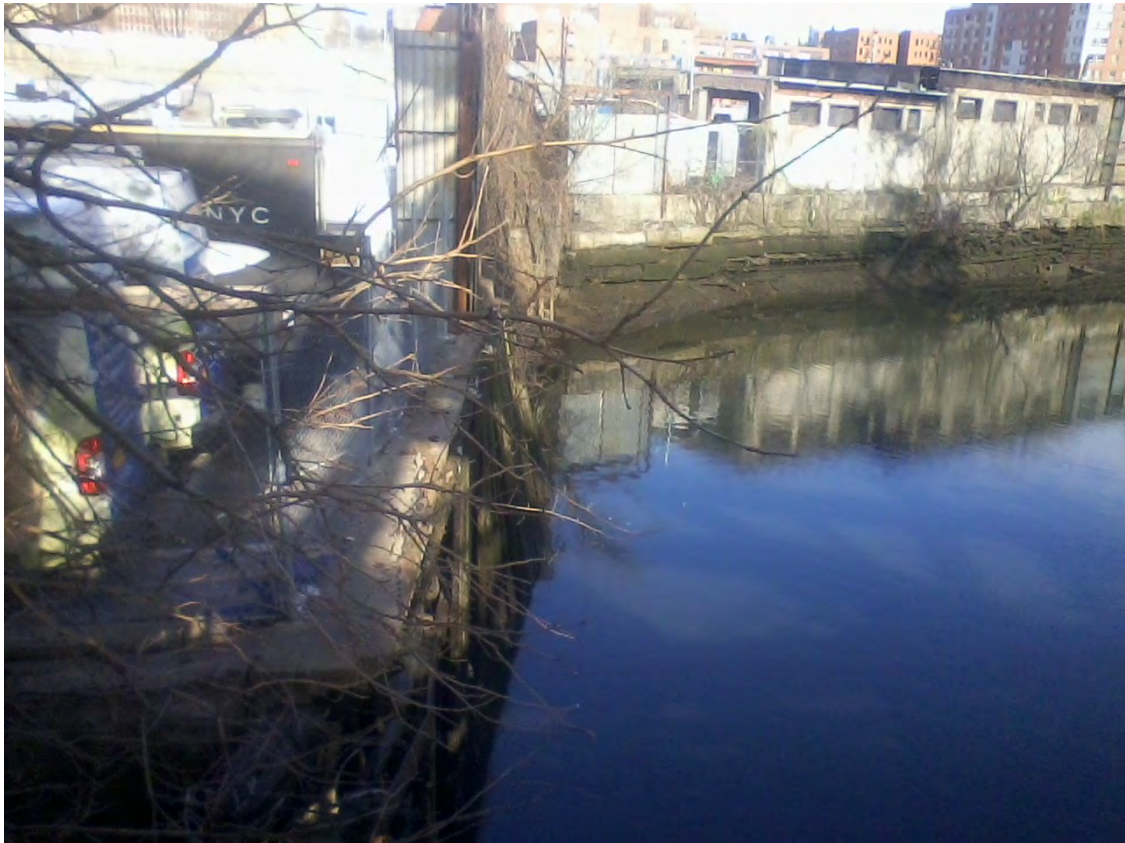
Photo 3 – View looking upstream from west side of existing drawbridge.
