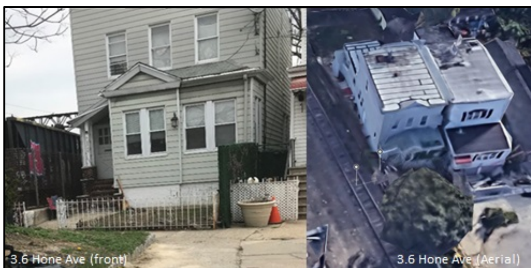
Figure 16-26. Receptor 3.6 – Hone Avenue Location Relative to Nearest Track on Railroad Right-of-Way
