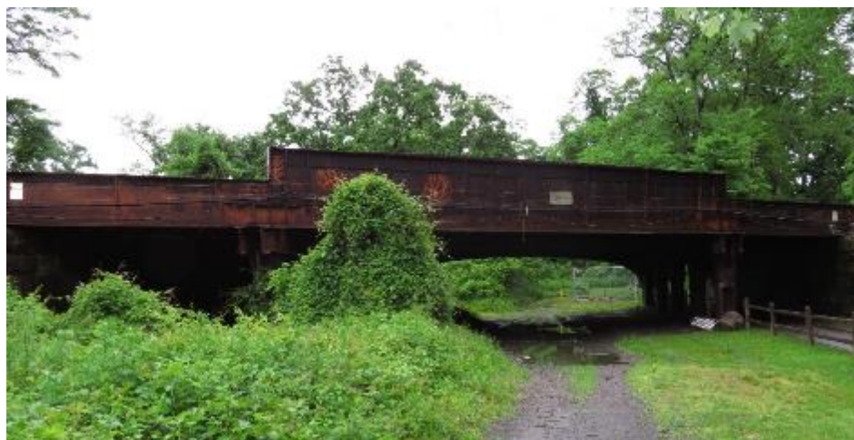
View of altered south side of the bridge
