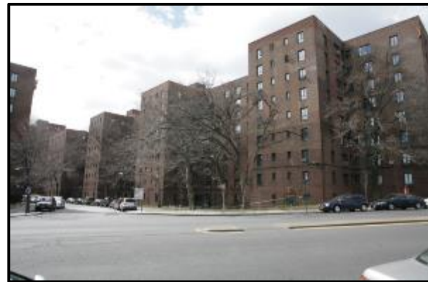
Photo 9-13. Parkchester Apartment Complex, E. Tremont Avenue, Facing Southwest. July 2013
