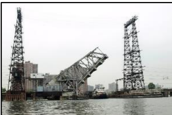
Photo 9-8. Amtrak Hell Gate Line Bascule Bridge over Pelham Bay and Hutchinson River, View Northwest. May 2013
