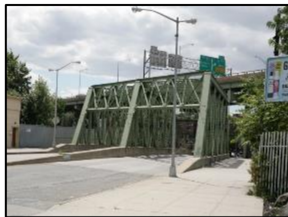
Photo 9-1. Lafayette Avenue Bridge over Amtrak Hell Gate Line, View West. May 2013
