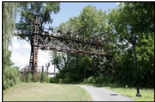
Photo 9-5. New York, Westchester & Boston Railway Anchor Bridge, View Northeast. May 2013
