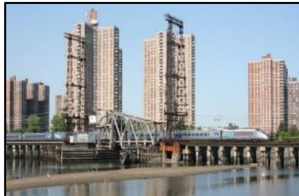
Photo 9-7. Amtrak Hell Gate Line Bascule Bridge over Pelham Bay and Hutchinson River, View West. May 2013
