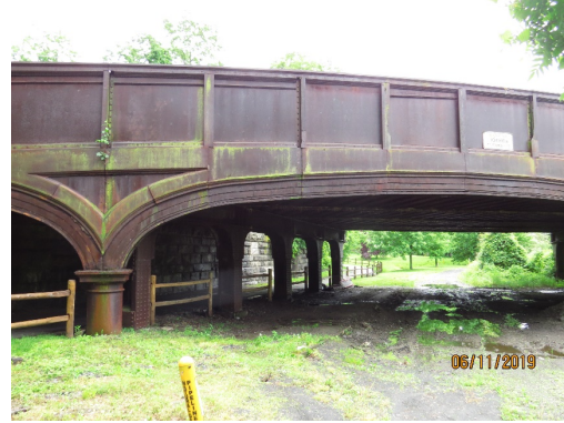
Photo 6-21. Segment 4: View looking southeast at Pelham Lane Pathway Bridge
