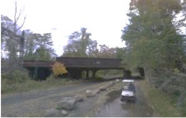
Photo 6-20. Segment 4: View looking northwest at Pelham Lane Pathway Bridge
