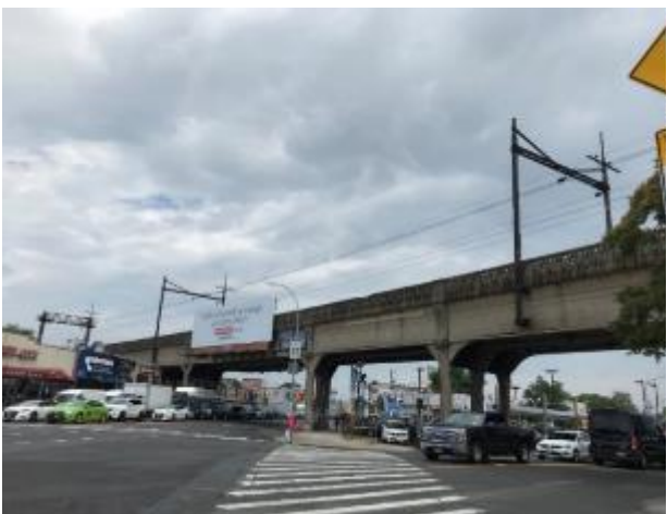
Photo 6-1. Segment 1: View of elevated tracks looking east from Northern Boulevard
