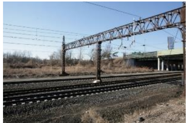
Photo 6-19. Segment 3: View looking southwest on Erskine Place at I-95 overpass
