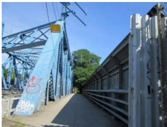
Photo 6-10. Segment 3: View looking north on Unionport Road Bridge
