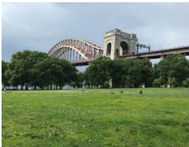
Photo 6-2. Segment 1: View of Hell Gate Bridge looking northwest from Astoria Park
