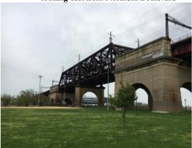
Photo 6-3. Segment 1: View of Randall's Island Connector looking northeast from Randall's Island Park
