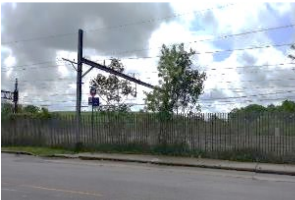
Photo 6-18. Segment 3: View looking south on Erskine Place at Pelham Bay Park
