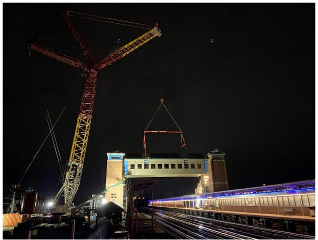
The picture above depicts the installation of the pedestrian overpass at the Elmont Station on the Main Line of the Long Island Rail Road. The work was done as part of Contract 6353 and took place over an outage during the weekend of March  $18^{th} - 20^{th}$ .
