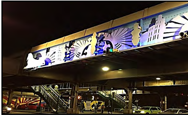
125th St. Lighting Improvement Project (SBMP)
