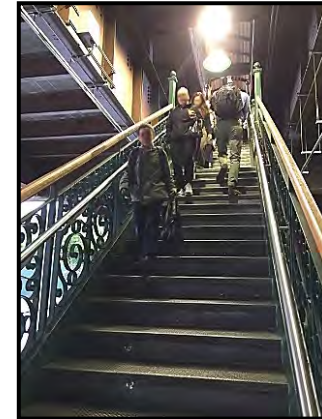
125th St. Stair Replacement Project (SBMP)
