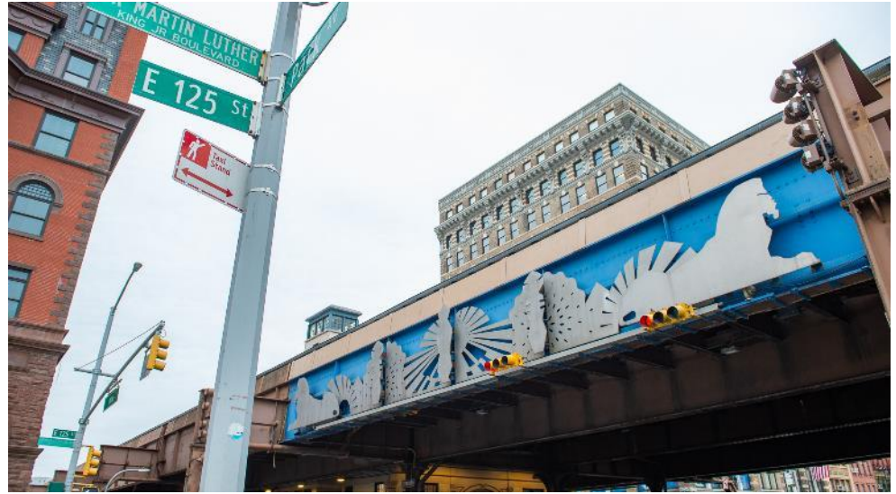
Harlem – 125th Street, Art Installation: Harlem Encore, 1999
