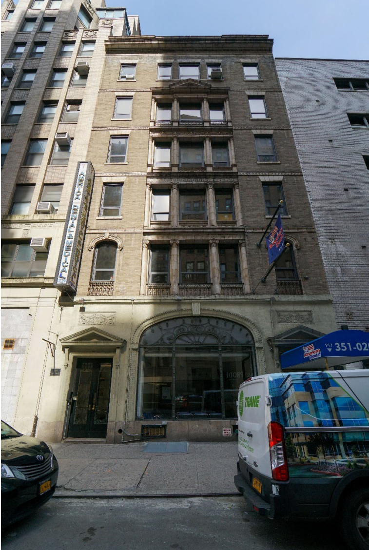
View facing north on West 30th Street
