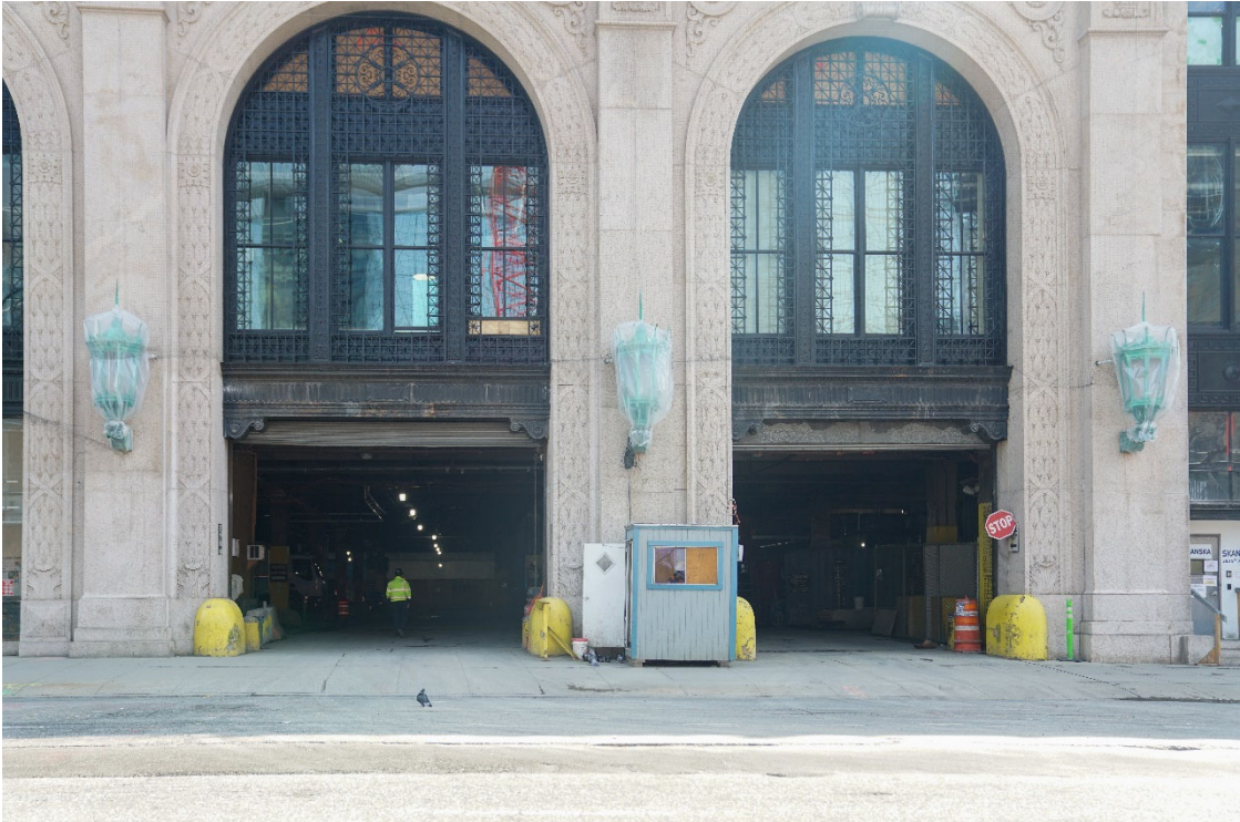
View facing north on West 31st Street
