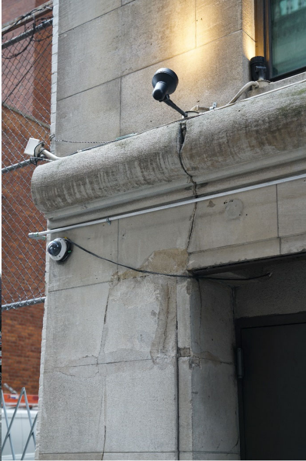
View of façade on West 31st Street
