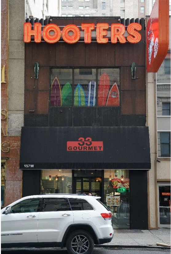
View facing north on West 33rd Street
