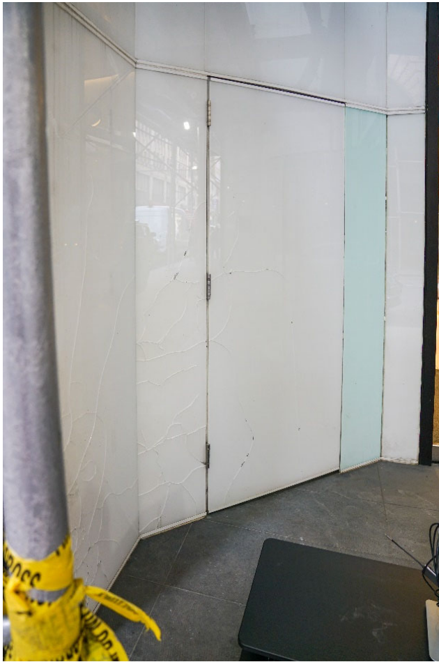
View of façade left of entryway
