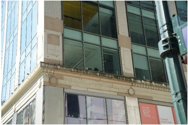
View of façade on corner of West 33rd Street and Avenue of the Americas
