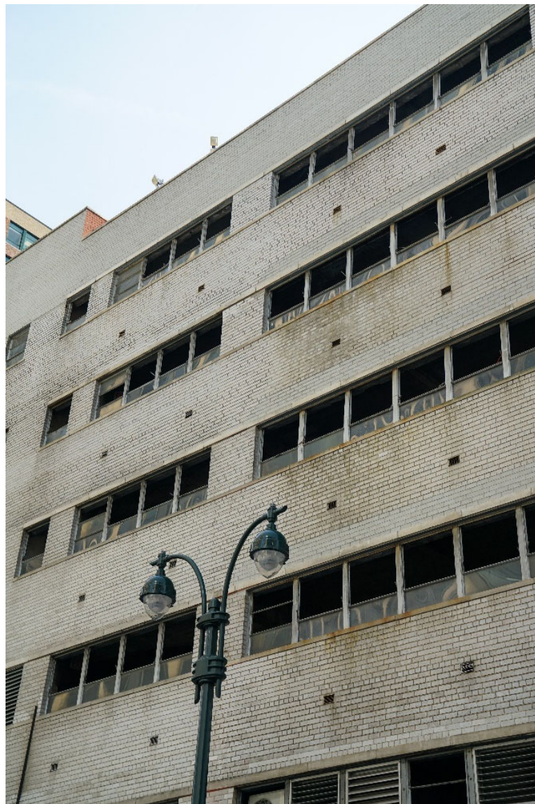
View of façade on West 31st Street
