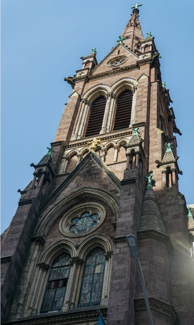
View of façade on West 30th Street
