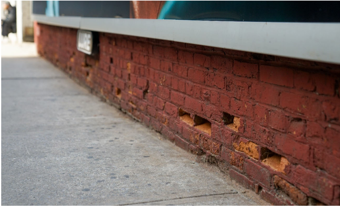
View of façade on West 30th Street
