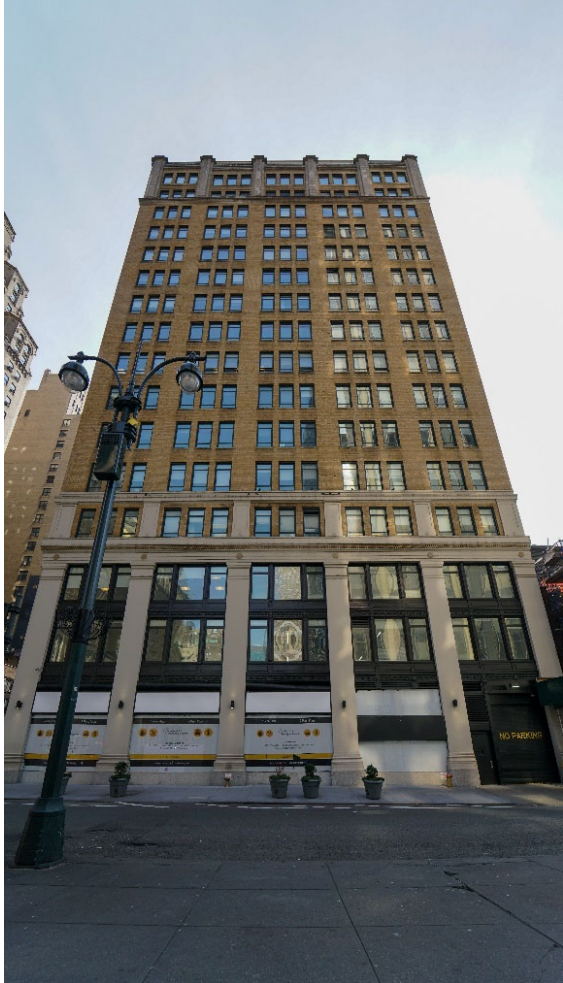
View facing south on West 31st Street
