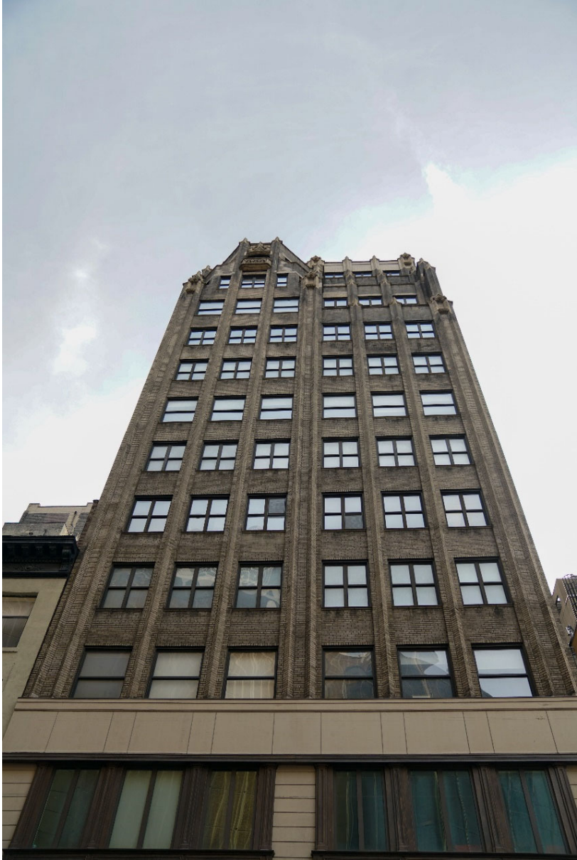
View facing south on West 31st Street
