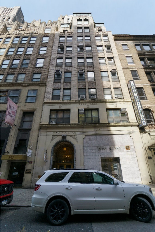
View facing north on West 30th Street
