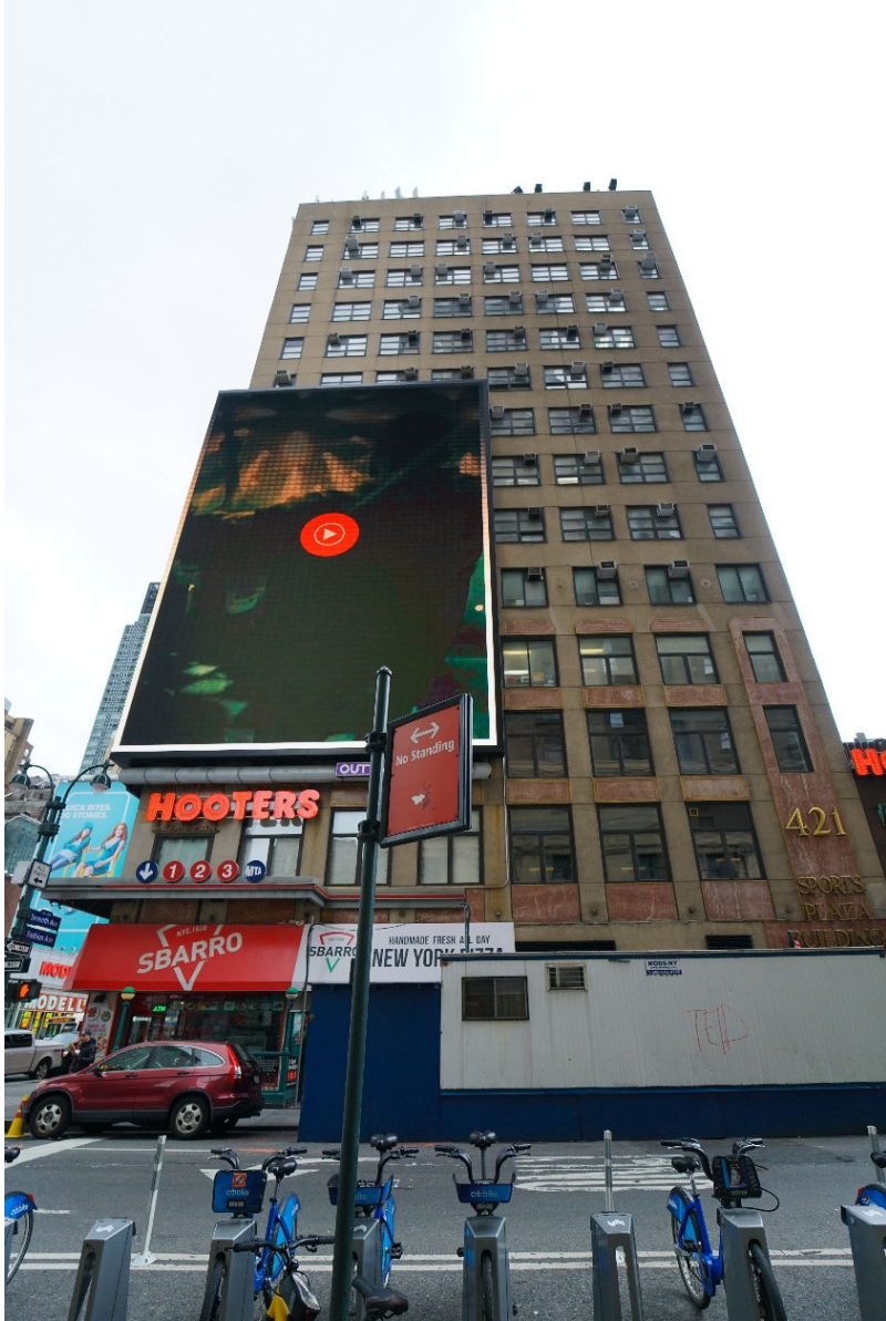
View facing north on West 33rd Street
