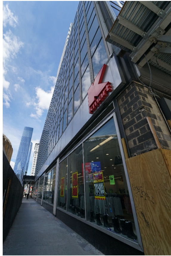
View facing west on West 33rd Street
