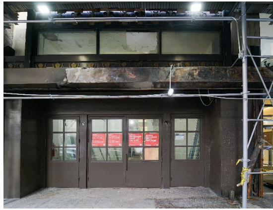
View facing north on West 30th Street
