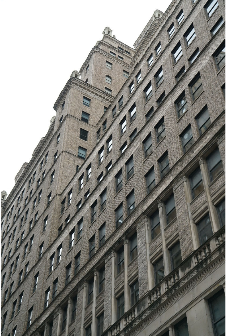
View of façade facing northwest on West 31st Street
