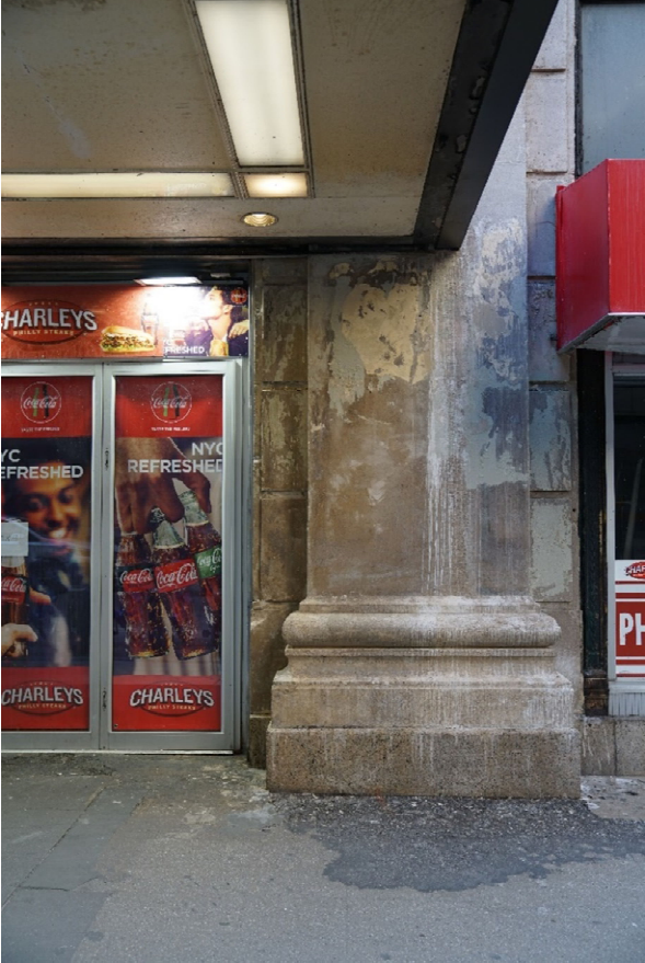
View of facade next to entrance on West 33rd Street
