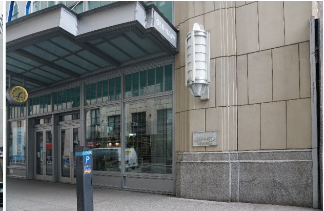
View facing north on West 33rd Street
