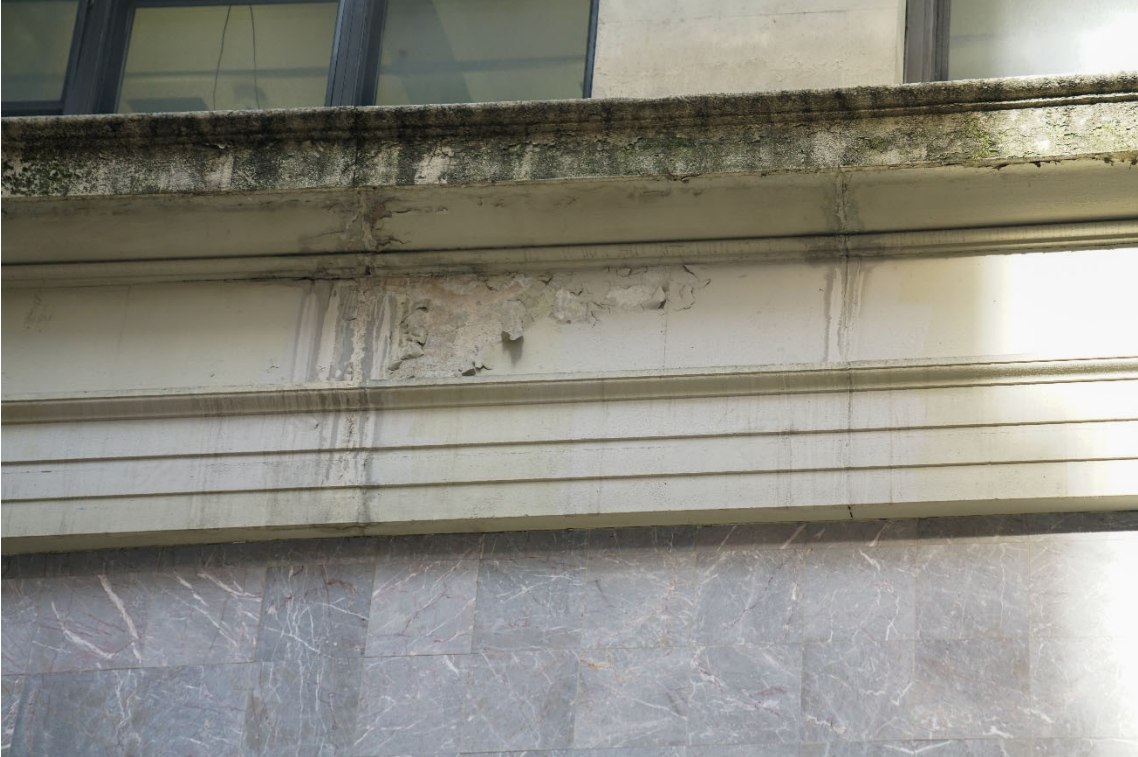
View of façade
