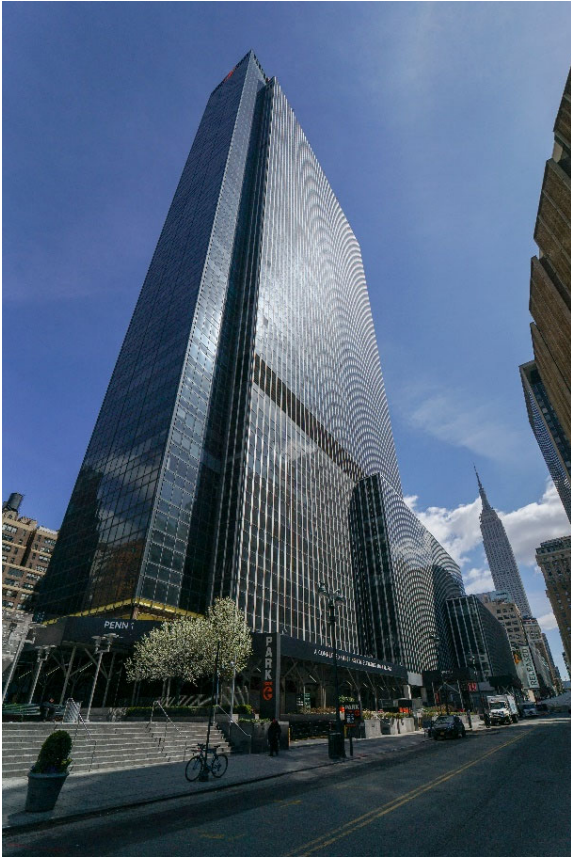
View facing northeast on West 33rd Street
