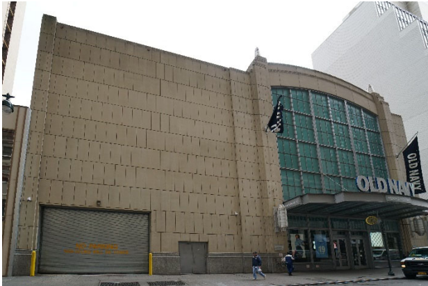
View facing north on West 33rd Street
