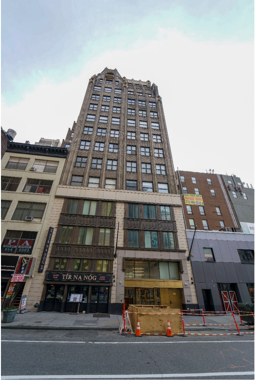
View facing south on West 31st Street
