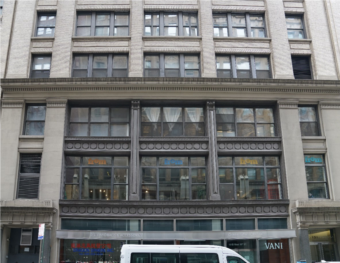
View facing north from West 30th Street
