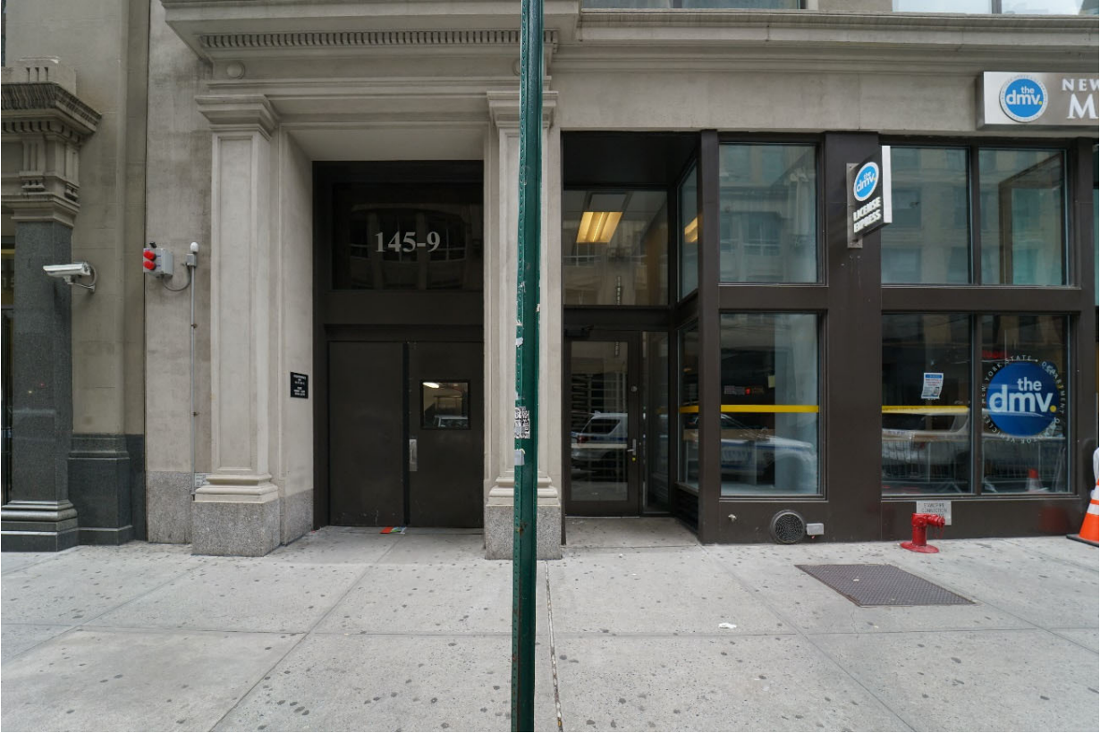
View facing north from West 30th Street
