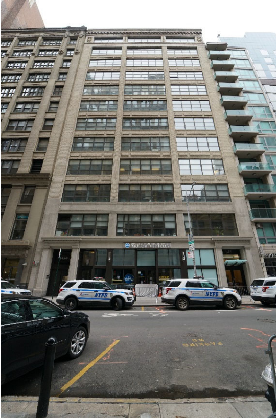
View facing north from West 30th Street
