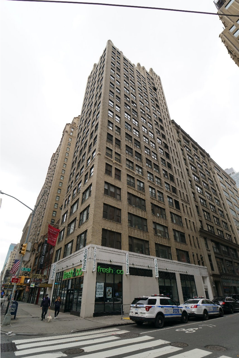
View facing northeast on West 30th Street
