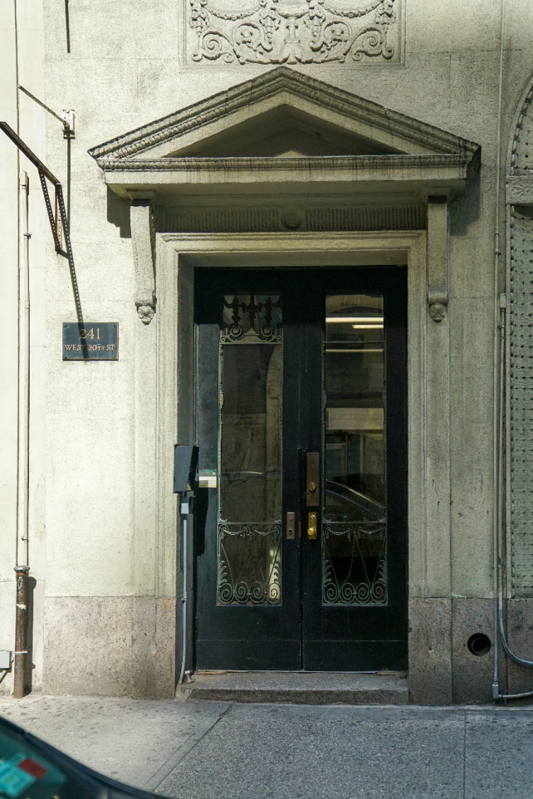
View facing north on West 30th Street
