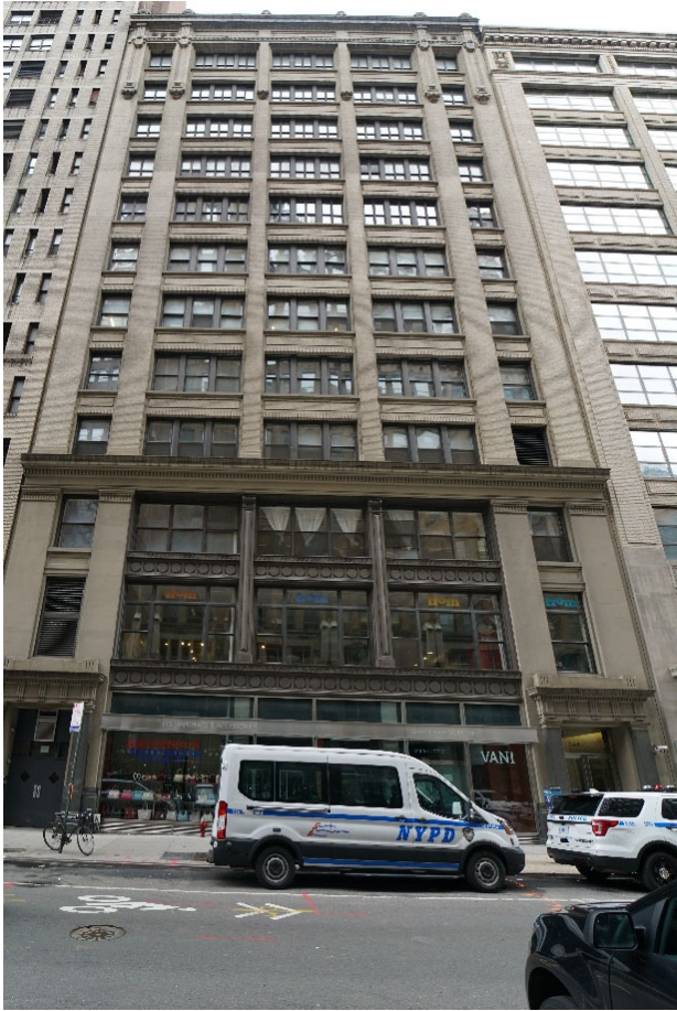
View facing north from West 30th Street
