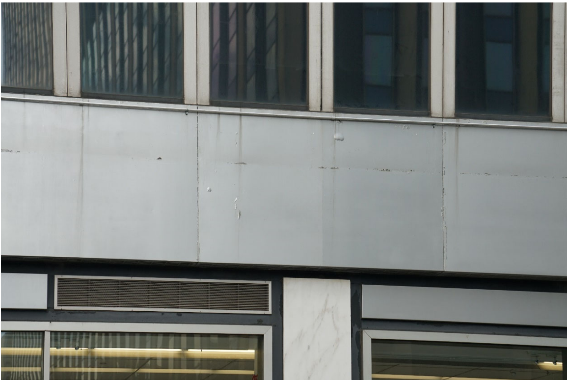
View of façade
