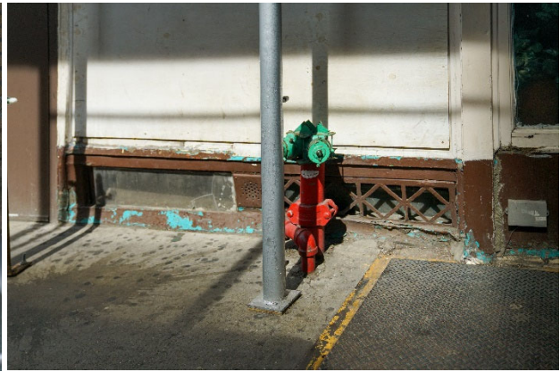
View of foundation
