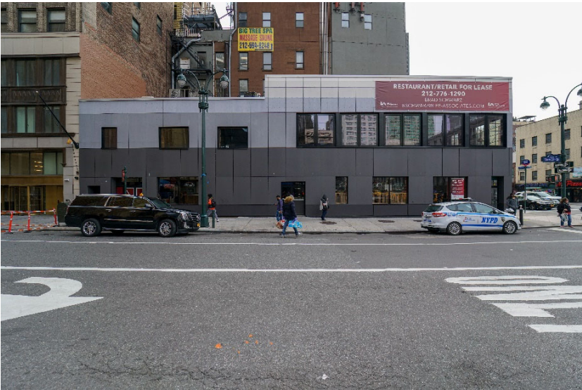
View facing south on West 31st Street
