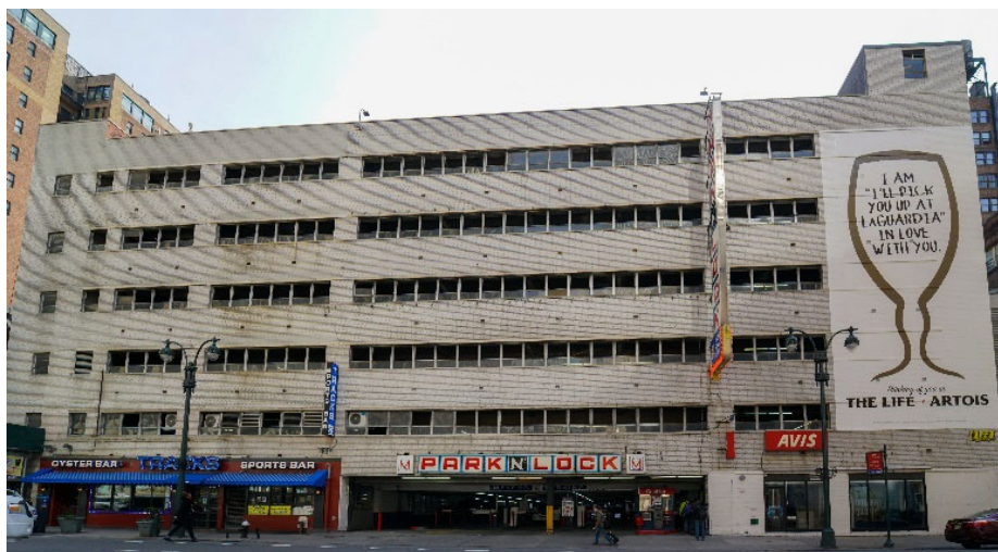
View facing south on West 31st Street
