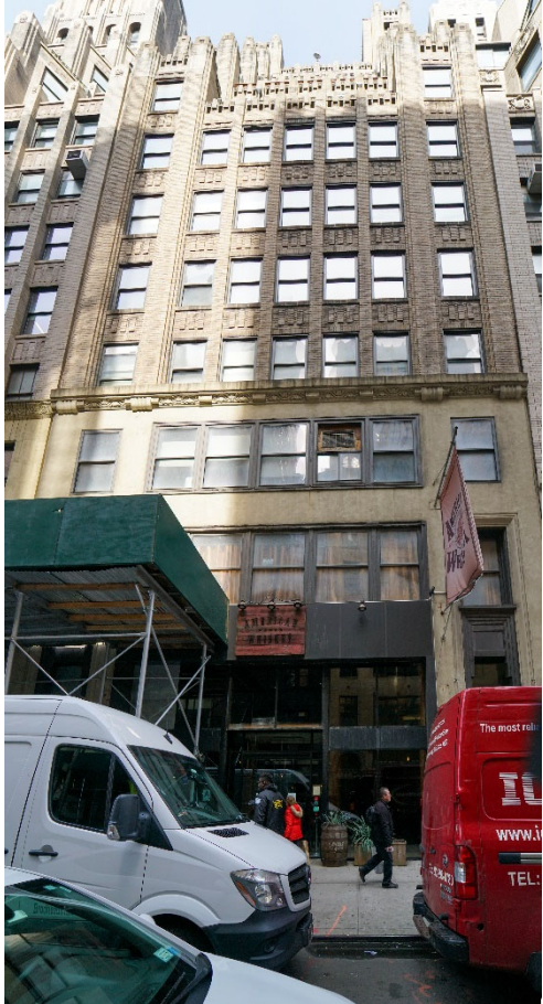
View facing north on West 30th Street
