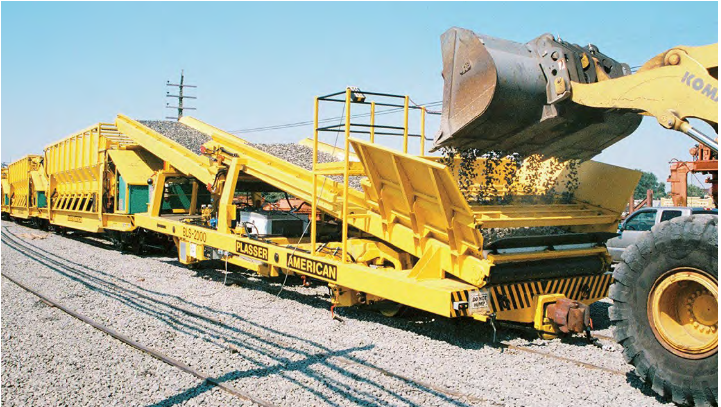
Ballast Placement
