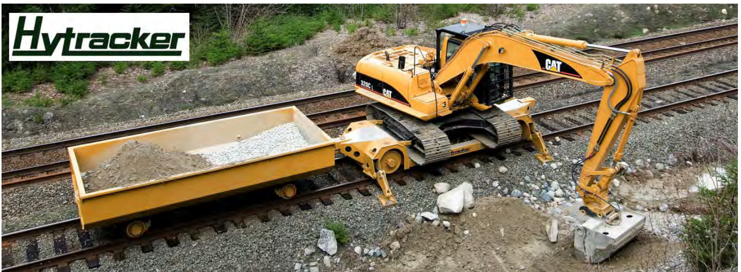
Side Load Rail Car with Ditching Gondola and Excavator
