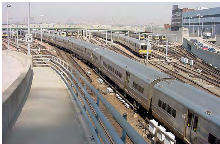
Rail Road WSSY Control System Upgrade
