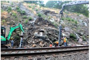
Rock slope remediation is the process of removing trees and debris from unstable rock faces
