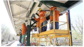
inspecting & repairing roofing, polishing shelter house glass, replacing "scratchitti" film on all windows (and replacing damaged ones), fixing ADA safety warning strips and renewing "Watch the Gap" stenciling on the platforms.
