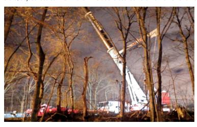
At the site of the old bridge piers. at about 2 AM, after the last New Haven line train has passed: Here, a 100-ton hydraulic crane lifts a 30-inch diameter by 65foot tubular truss. This supporting structure was lowered to, and spanned across the old bridge piers. It is at this point along our
