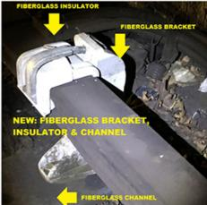
They developed a new fiberglass bracket design, and fiberglass channel design, materials that provide longevity and ample insulation.
