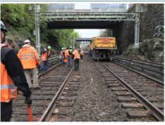
we will be replacing about 4,000 feet of rail and about 2,000 rail ties, removing and replacing about 600 feet of ballast (the cut stone under the tracks that provides support, and drains excess water), inspecting all of the track in that section for possible defects, and testing the rail for safety.
