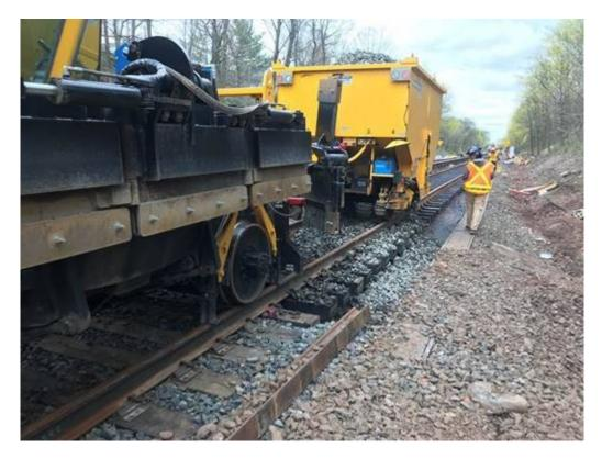
The photo depicts a ballast hopper dropping ballast onto new trackwork including new railroad ties, contact and running rail, that was recently installed between Tysens Lane and the Jefferson Avenue Station as part of Phase I of the Mainline Track Replacement Program for the Staten Island Railway under Contract T-80280.
