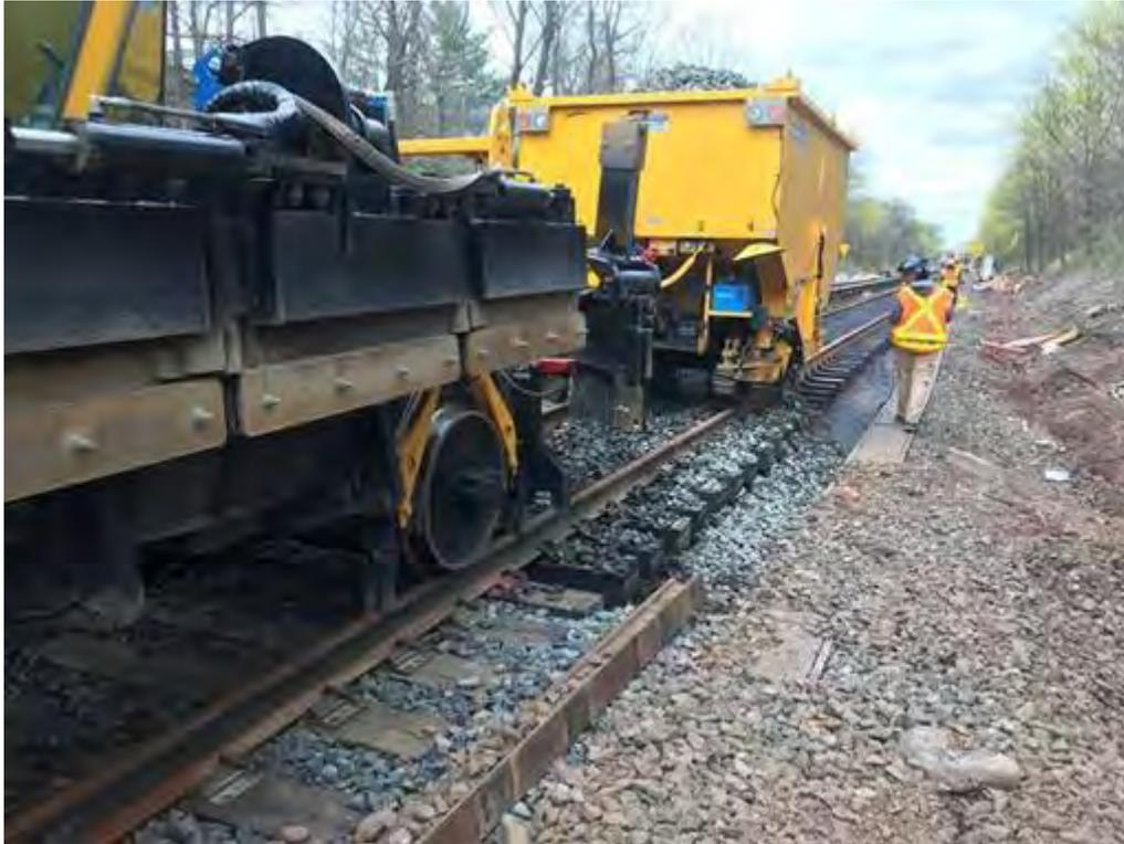
The photo depicts a ballast hopper dropping ballast onto new trackwork including new railroad ties, contact and running rail, that was recently installed between Tysens Lane and the Jefferson Avenue Station as part of Phase I of the Mainline Track Replacement Program for the Staten Island Railway under Contract T-80280.
