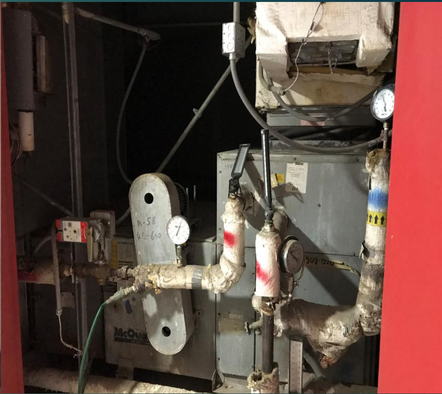
Existing Unit on the second floor
