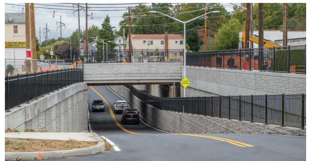
The Urban Avenue crossing closed Mar 8, 2019 and reopened as an underpass Sep 6, 2019.
