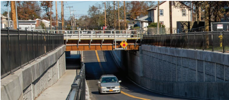
The Covert Avenue crossing closed on Apr 15, 2019 and reopened as an underpass on Oct 12, 2019.
