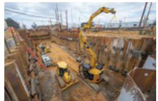
The South 12 Street crossing closed on Oct 24, 2020 and is being rebuilt as an underpass for pedestrians, to open in summer 2021.
