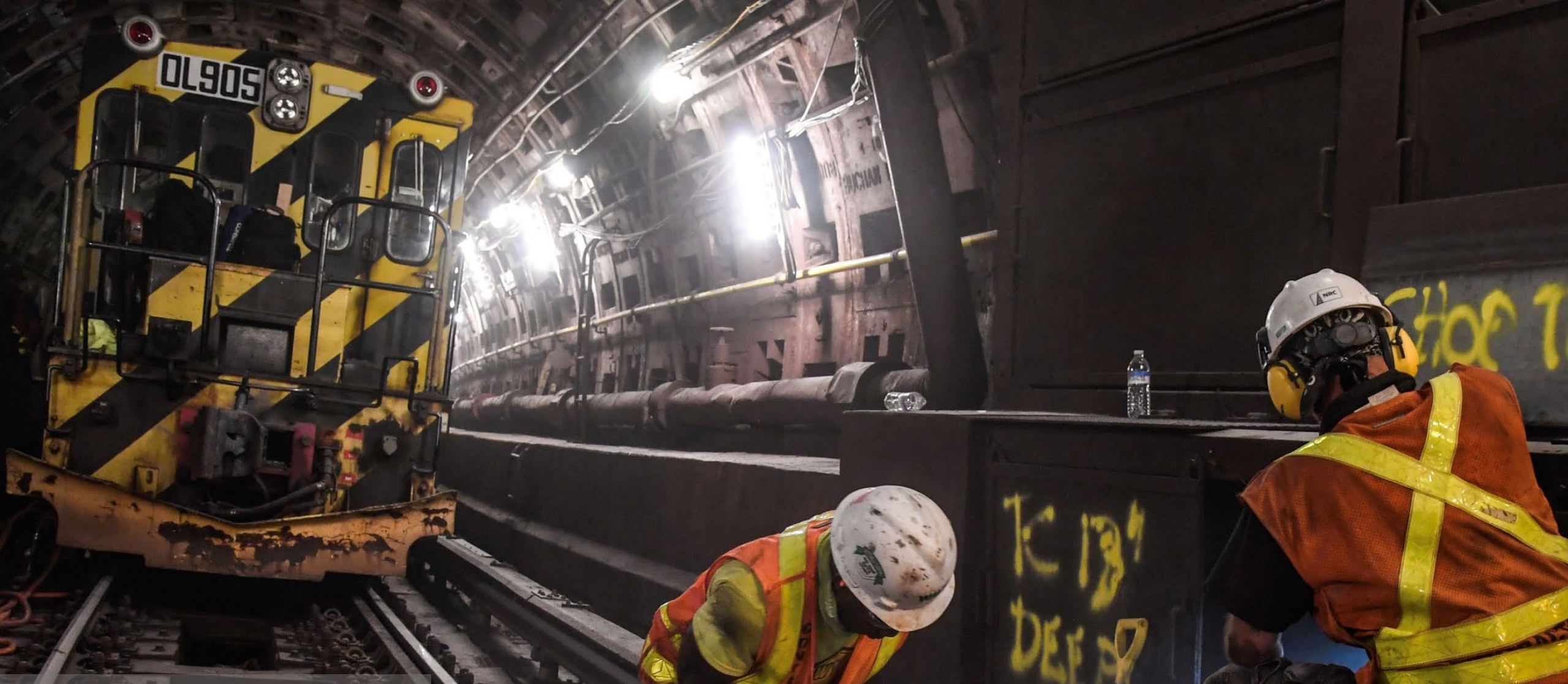
Photo: NYCT Track Replacement - Archer Ave. Line - Queens
