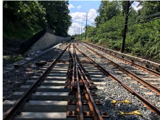
New Eastern Crossover (Looking West)
