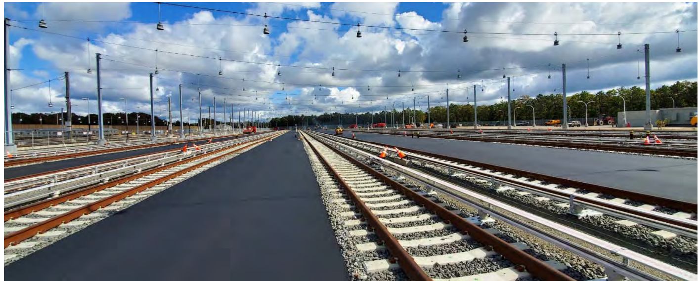
OVERVIEW OF THE NEARLY COMPLETED YARD,
