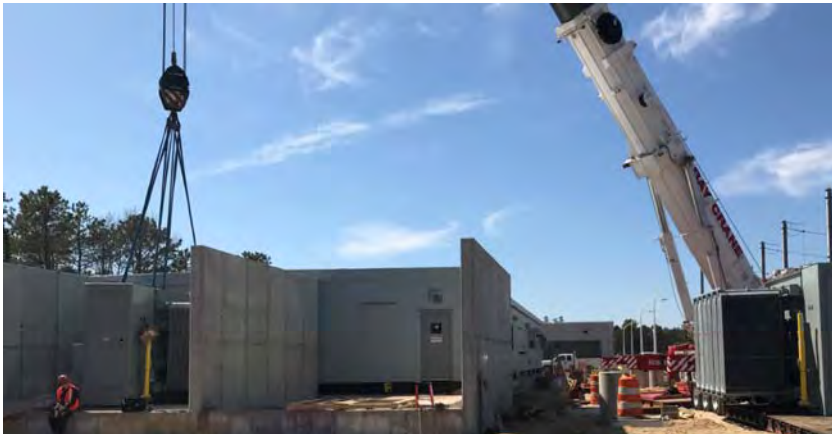
INSTALLATION OF THE NUMBER 2 RECTIFIER
