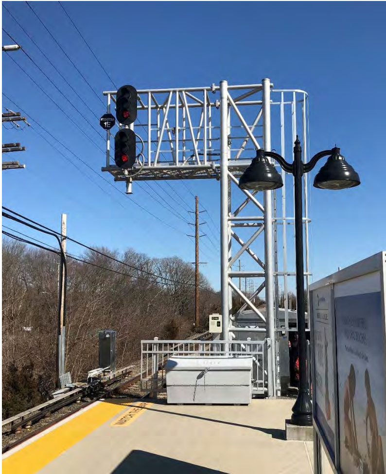
Signal Bridge, Montauk Track 1
