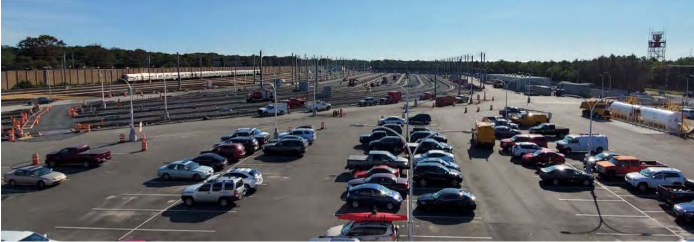
OVERVIEW OF THE NEARLY COMPLETED YARD, LOOKING EAST
