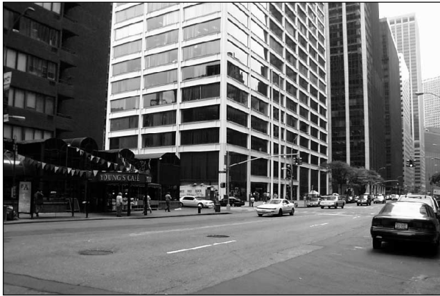
East side of Water Street, view south from Fletcher Street 6
