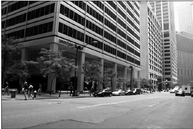
East side of Water Street, view south from Gouverneur Lane 8
