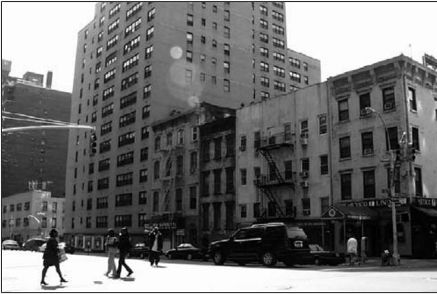
West side of Second Avenue, view south from 26th Street 1
