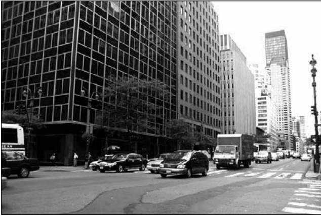
West side of Second Avenue, view north from 42nd Street 1
