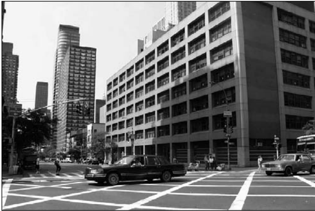
West side of Second Avenue, view south from 57th Street 3
