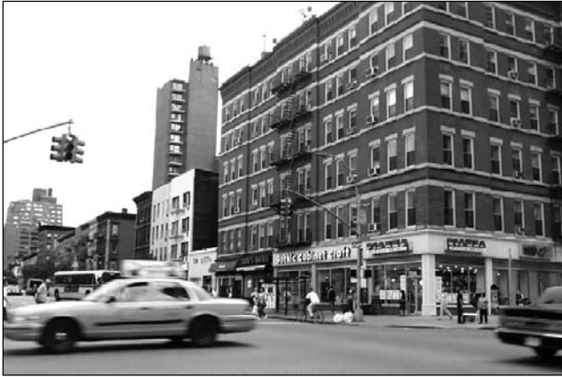
West side of Second Avenue, view south from 86th Street 1
